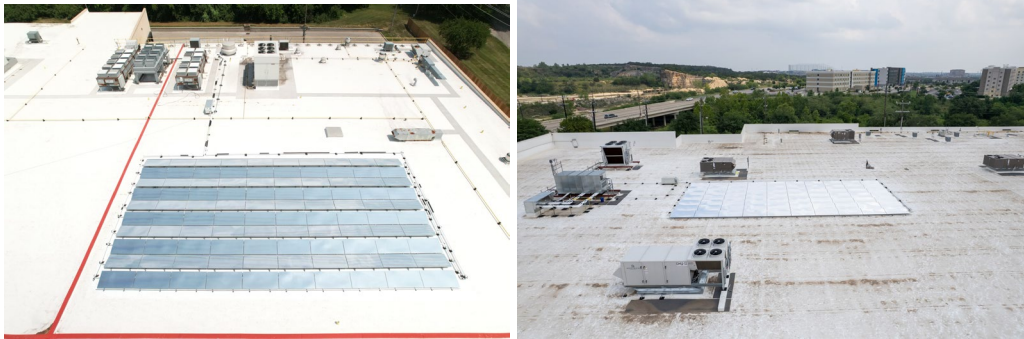
Figure 30: SkyCool arrays deployed in 2023; the left image shows an array of 100 panels and the right image an array of 70 panels
