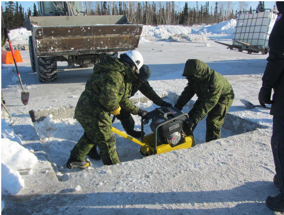
Figure B-4. Vibratory plate compactor consolidating the top of a completed lift.
