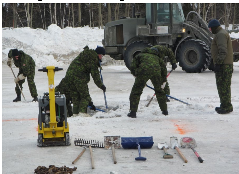
Figure B-3. Manual leveling of snow blown into crater.
