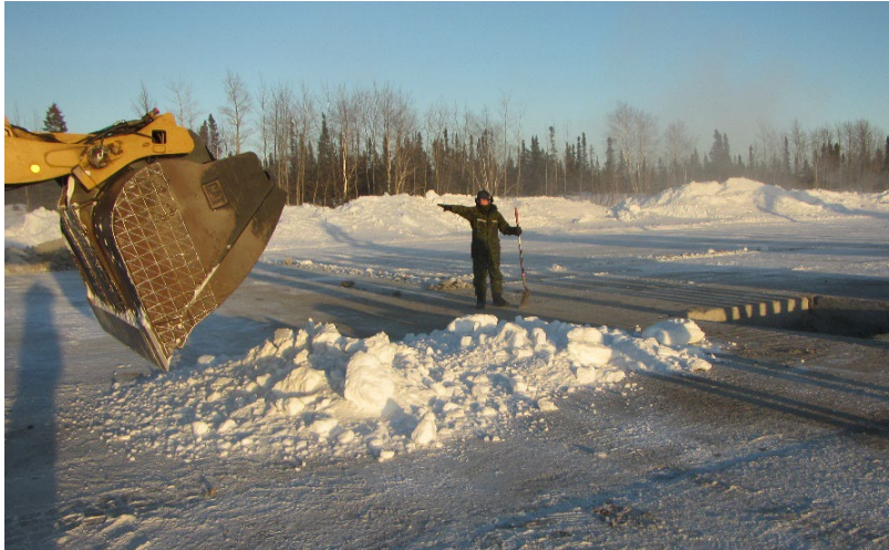
Figure 41. Placing snow from stockpile adjacent to repair.
