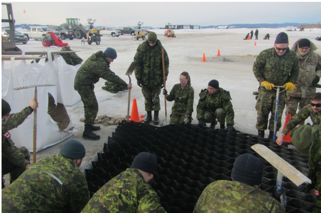
Figure 46. Expanding geocells inside repair.
