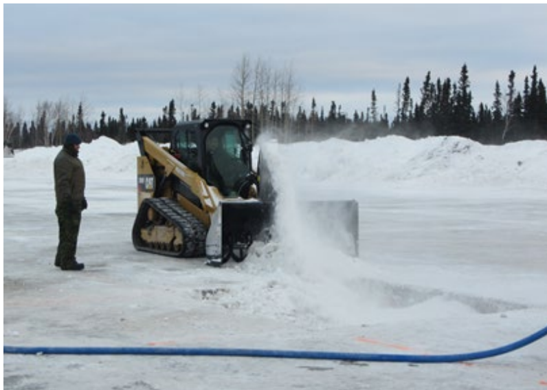
Figure 31. Snowblower mixing wetted snow and ejecting it into the crater in preparation for manual leveling and compacting in prescribed lifts.
