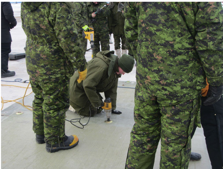
Figure 53. Tightening of FRP connector bushings with impact wrench.
