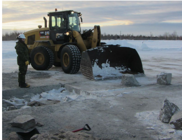
Figure 38. Debris removal with front-end loader.
