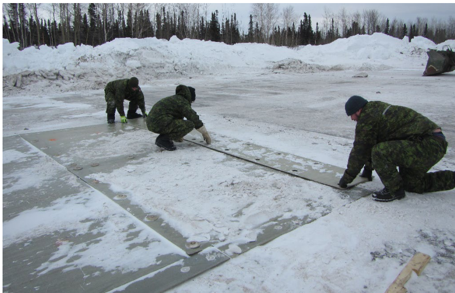
Figure 52. Installation of FRP anchor panel.
