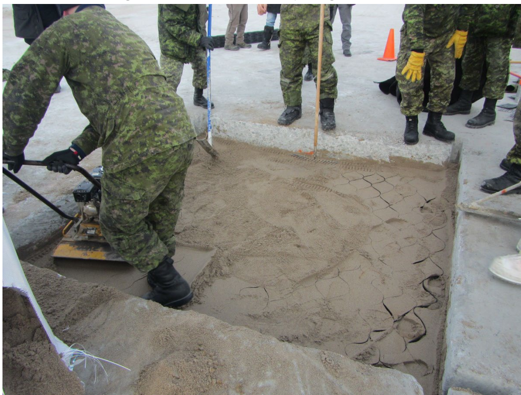
Figure 48. Compaction of first layer of geocell backfill.
