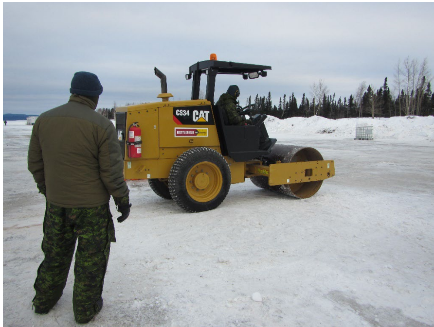
Figure B-5. Vibratory drum roller compacting top of a completed crater patch.
