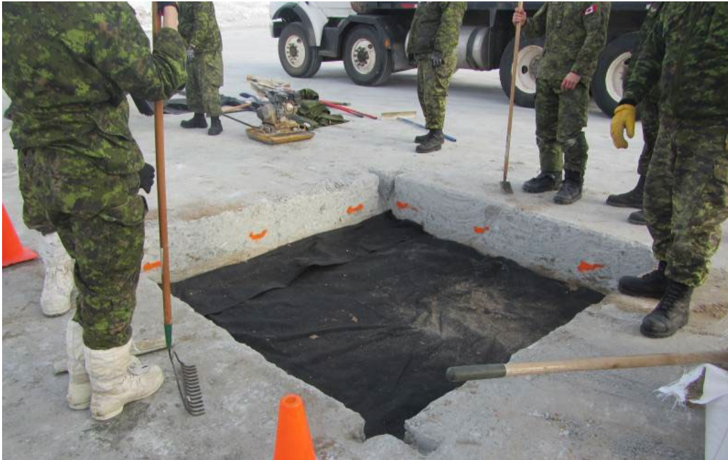
Figure 45. Geotextile installed below geocell layers.
