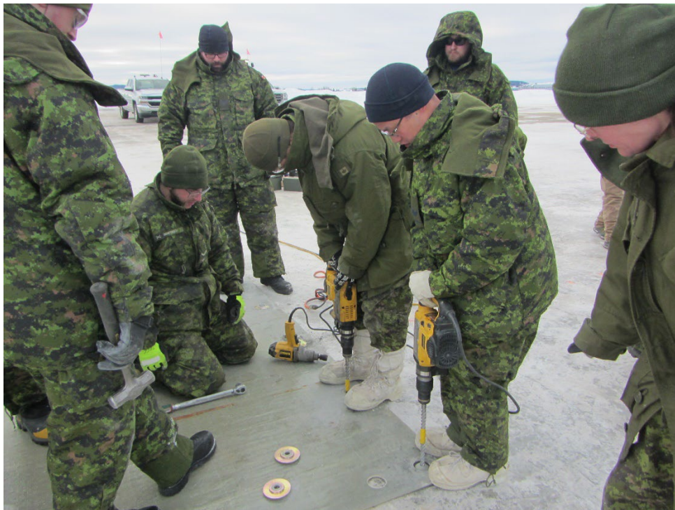
Figure 54. Drilling anchor hole with spotter.
