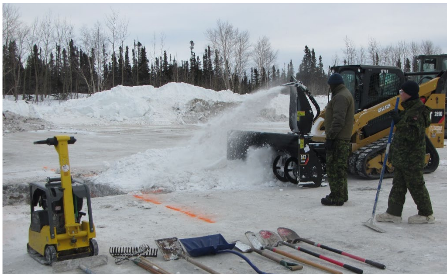
Figure B-2. Snow being blown into crater in lifts in preparation for leveling and compaction.
