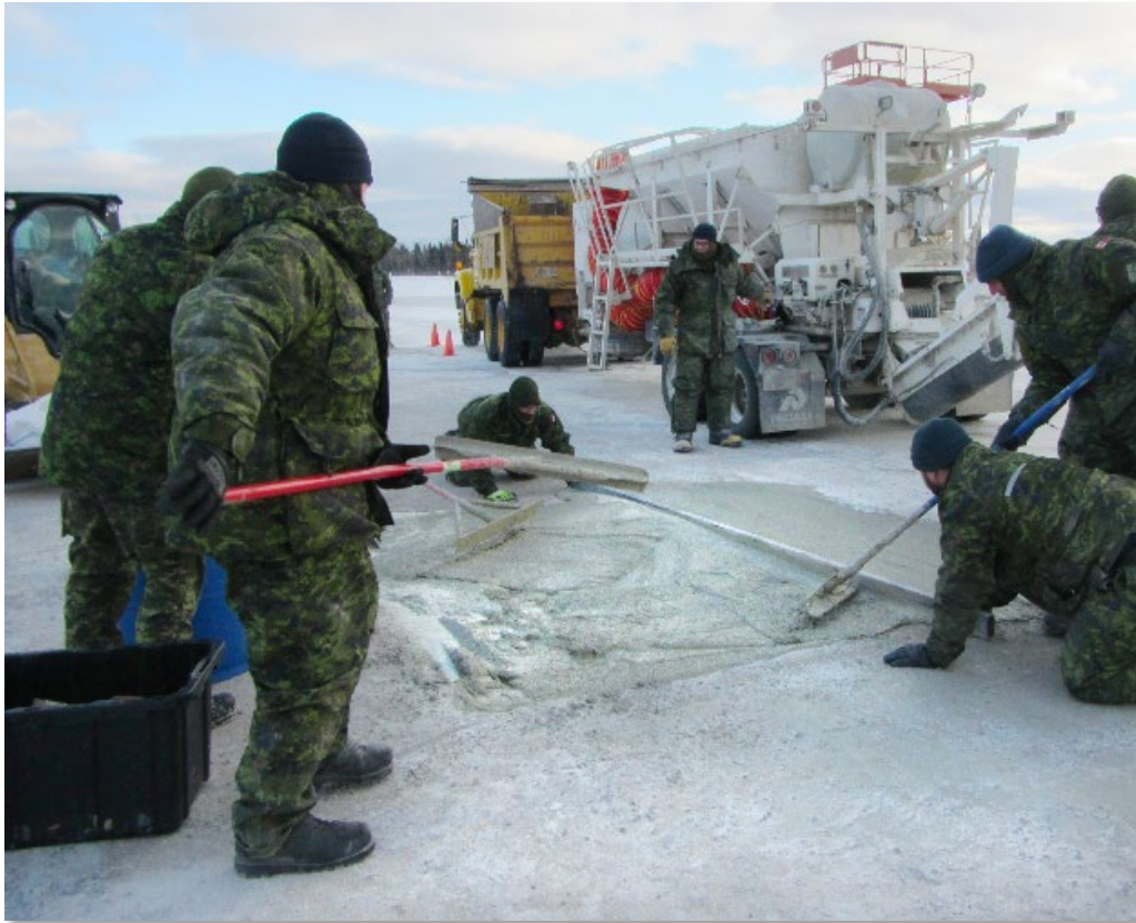
Figure 57. Striking off RSC with magnesium screed bar.
