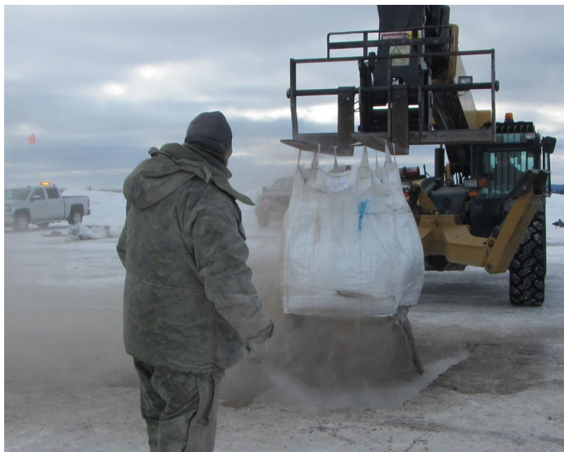
Figure 49. Placement of dry RSFF.
