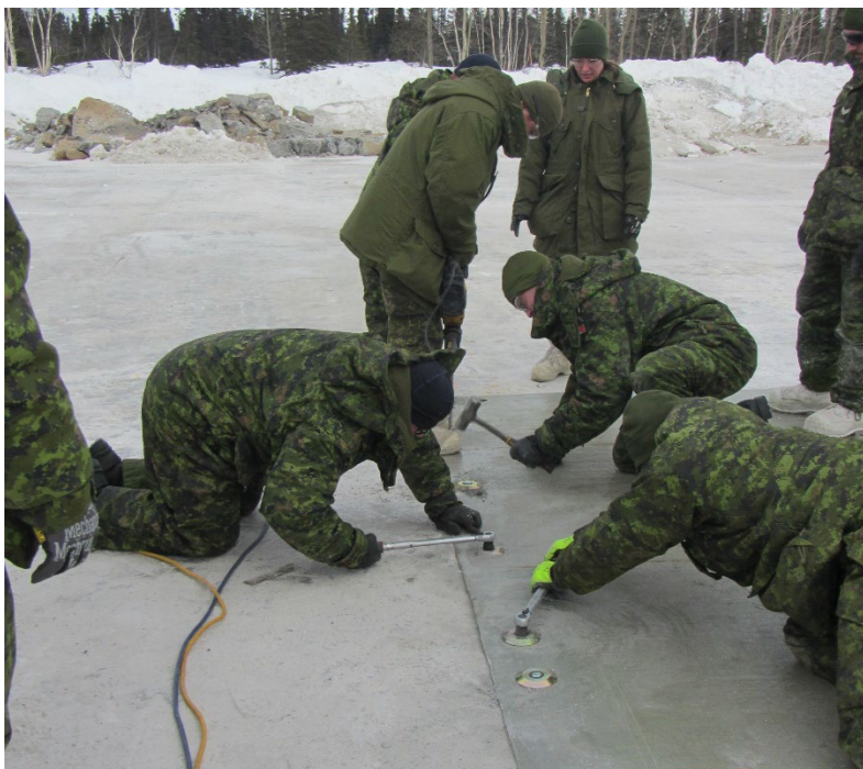
Figure 55. Final torque check on installed anchor.
