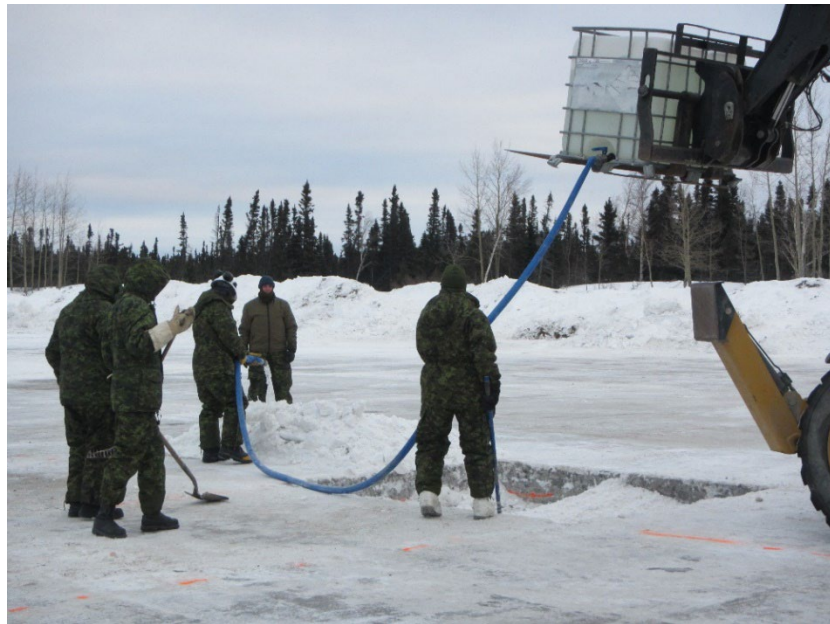
Figure 30. Adding water to harvested snow.
