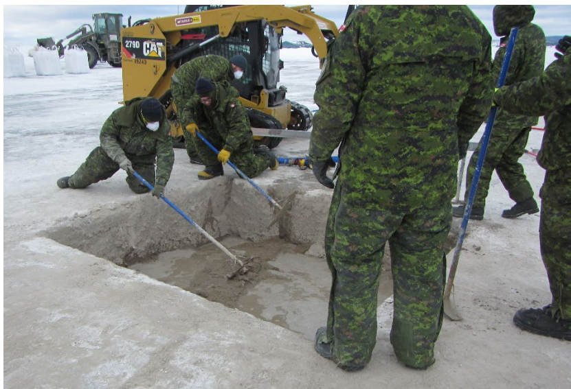
Figure 50. Leveling dry RSFF with hand tools.
