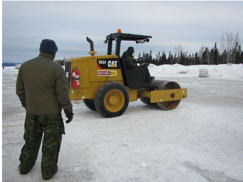
Figure 44. Compaction of final lift of snow-water slurry with vibratory roller compactor.
