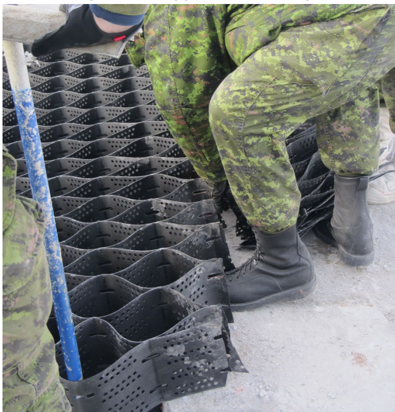
Figure 47. Cutting geocells to proper length.
