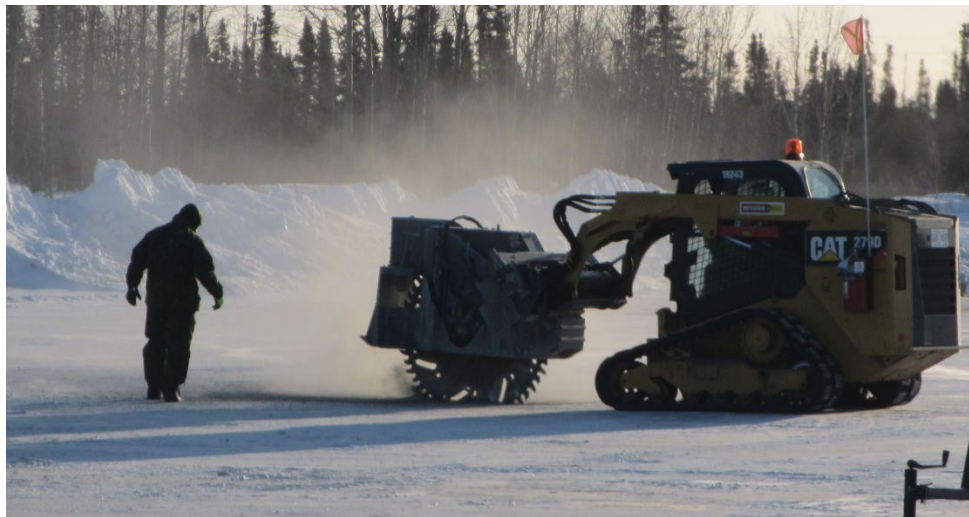
Figure 39. Pavement cutting with CTL, saw attachment, and spotter.
