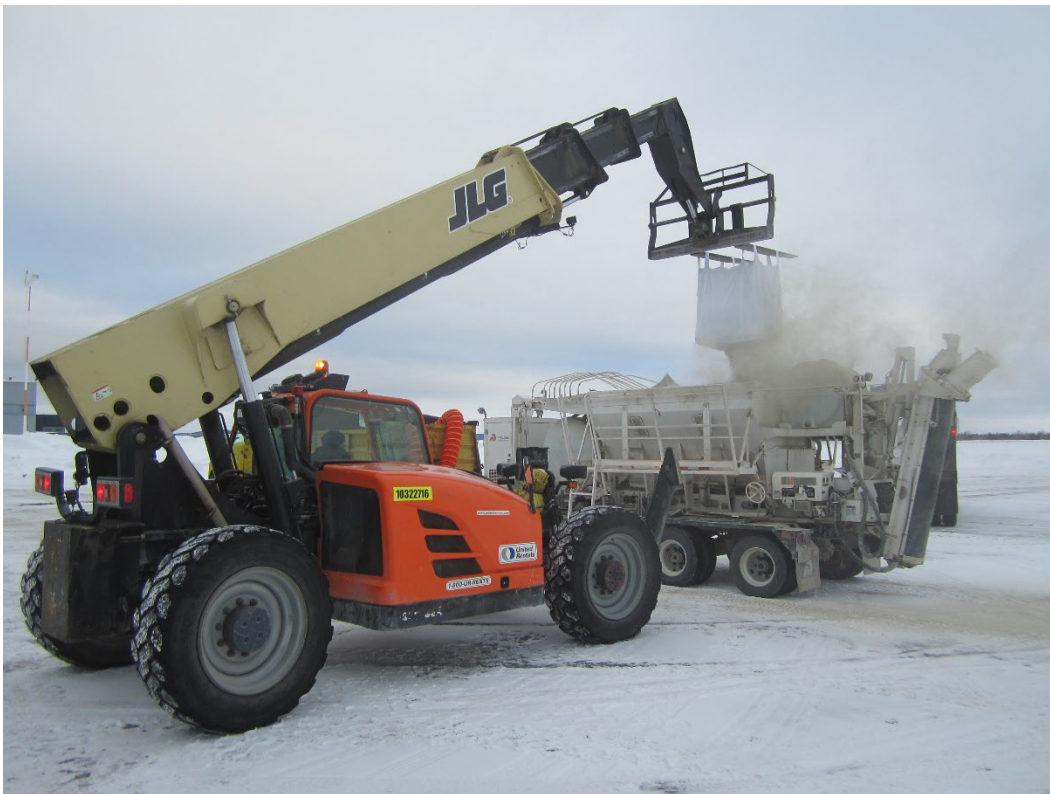
Figure 56. Loading super sacks into dry material bin.
