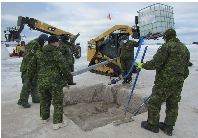
Figure 51. Dispensing water over dry RSFF.
