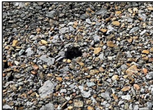
(b) Typical 1/4 to 3/4 in. surface void
