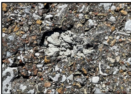
(e) Deteriorating soft aggregate particle
