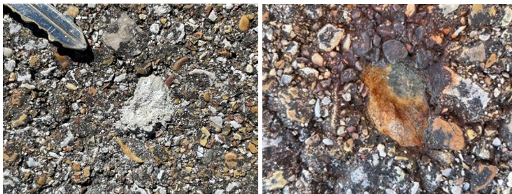
(a) Intrusion of low-quality aggregate
