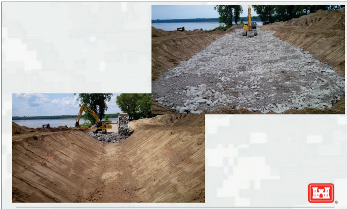
Figure 21. Example revetment key on the Mississippi River. Images reproduced from USACE Vicksburg District (n.d.).
