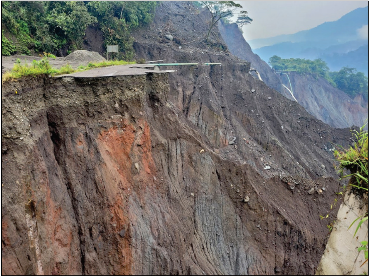
Figure 3. Regressive erosion on the Rio Coca at a tributary bridge on C. Teniente Hugo Ortiz, approximately 550 m northwest of San Luis, Ecuador.
