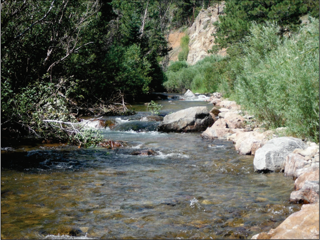
Figure 19. The Boulder Creek, Colorado, stabilization project was completed using onsite large boulders and well-graded finer materials to reestablish cascades, falls, pools, and revegetation.
