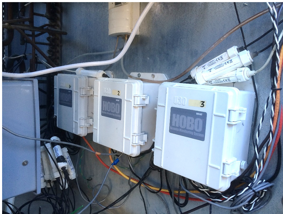
Figure 30. HOBO Dataloggers Installed in Baseline Unit at Fort Irwin OSJA.
