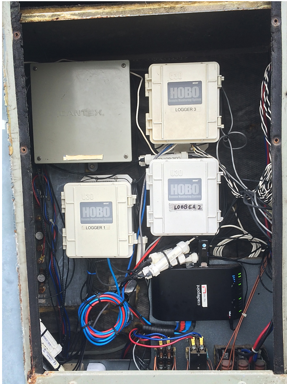
Figure 12. HOBO Dataloggers Installed in Baseline Unit at CCSFS-NOTU.
