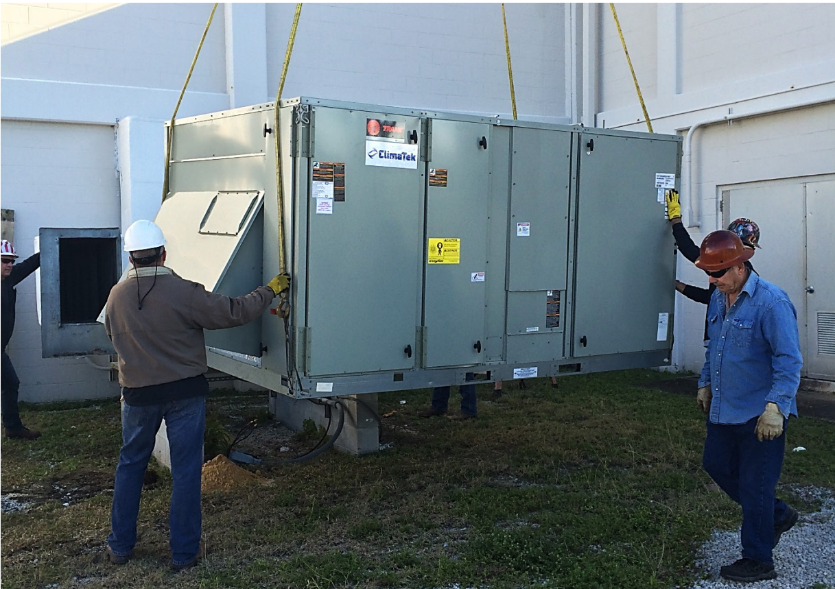
Figure 10. Advanced NexGen Cooling Package Unit Being Installed at CCSFS NOTU Support Building.
