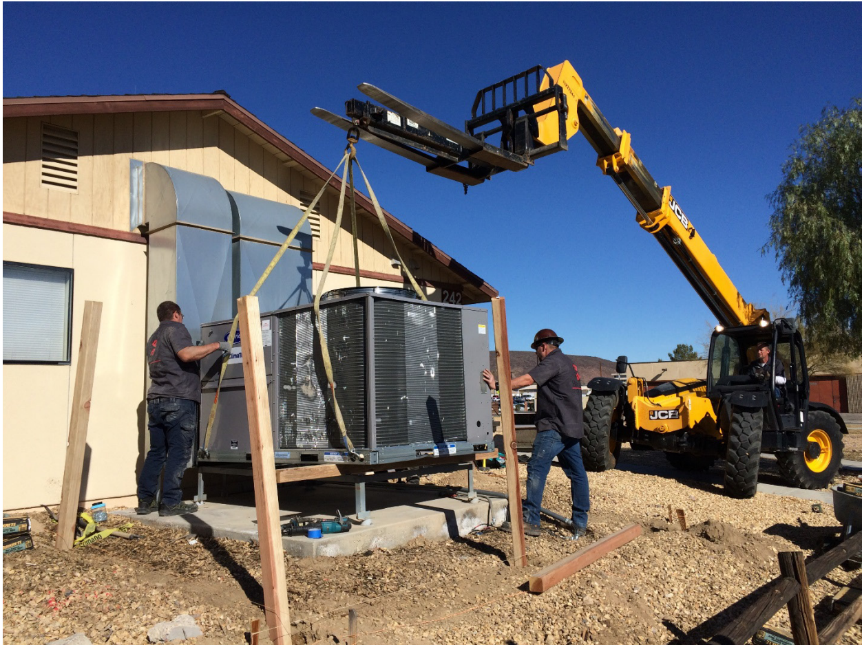
Figure 9. Advanced NexGen Heat-pump Package Unit Being Installed at Fort Irwin OSJA Building.
