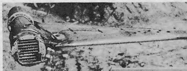
Figure 3 - Engine mounted on rotor tip
