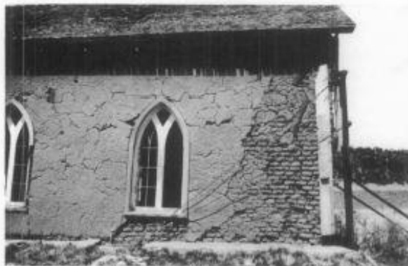
Deteriorated Adobe Building. By virtue of its fragile nature, the adobe building must be restored by thorough, systematic, and professional measures that will insure its future survival. (Technical Preservation Services Division)
