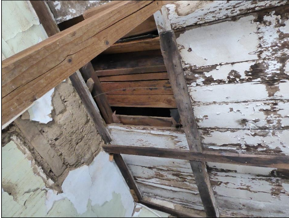
Figure 108. Multisized and multiaged wooden members supporting the ceiling within the José María Gil Adobe, 2021. (ERDC-CERL.)
