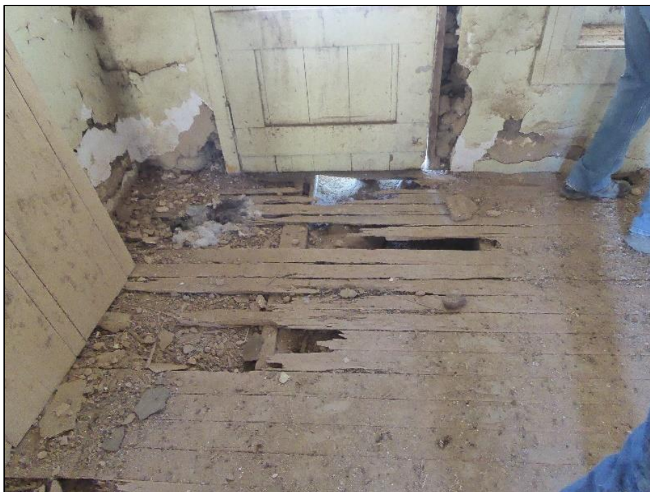
Figure 112. Wood strip flooring with breakthrough areas near an exterior door of the José María Gil Adobe, 2021. (ERDC-CERL.)
