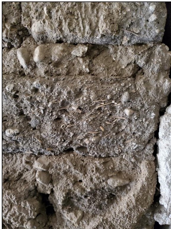
Figure 196. Bricks having dark gray color with rounded aggregates and a high fraction of straw reinforcement.
