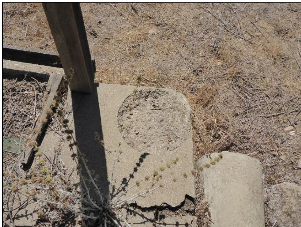
Figure 138. Concrete base with separated concrete column on the south corner of the José María Gil Adobe, 2021. (ERDC-CERL.)
