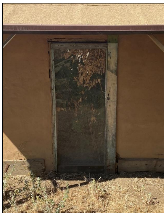
Figure 40. Plexiglass in the door opening on the northeast side of the cold storage building, 2021. (ERDC-CERL.)
