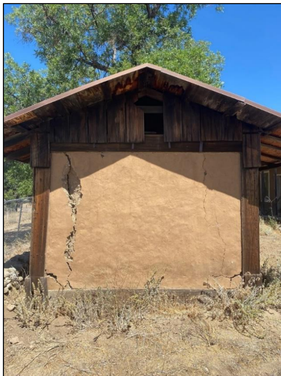
Figure 48. Wooden trim boards along base and corners of the cold storage building, 2021. (ERDC-CERL.)
