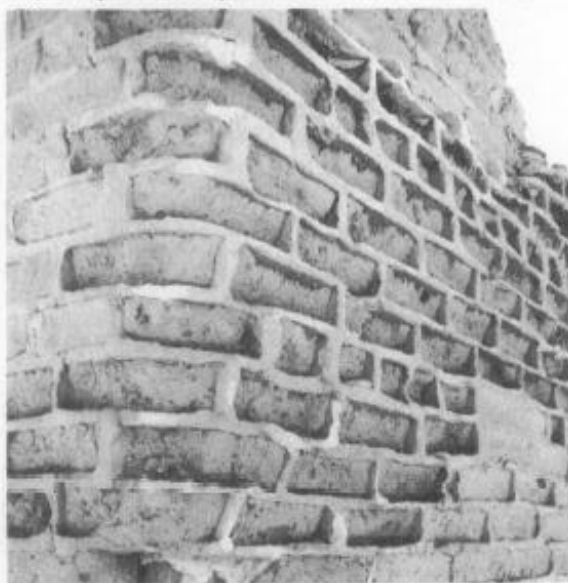
Cement Mortar Incompatibility. The stronger and less flexible cement mortar has caused the softer adobe bricks to crumble thus leaving a "honeycomb" of cement mortar joints. (National Park Service)
