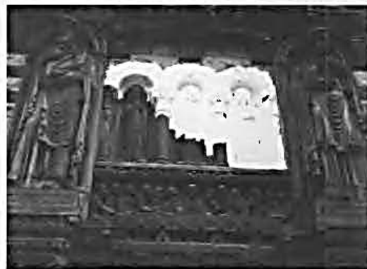
Figure 17. A poultice is being used to remove salts from the brownstone statuary on the facade of this late-19th century stone church. Photo: National Park Service Files.
