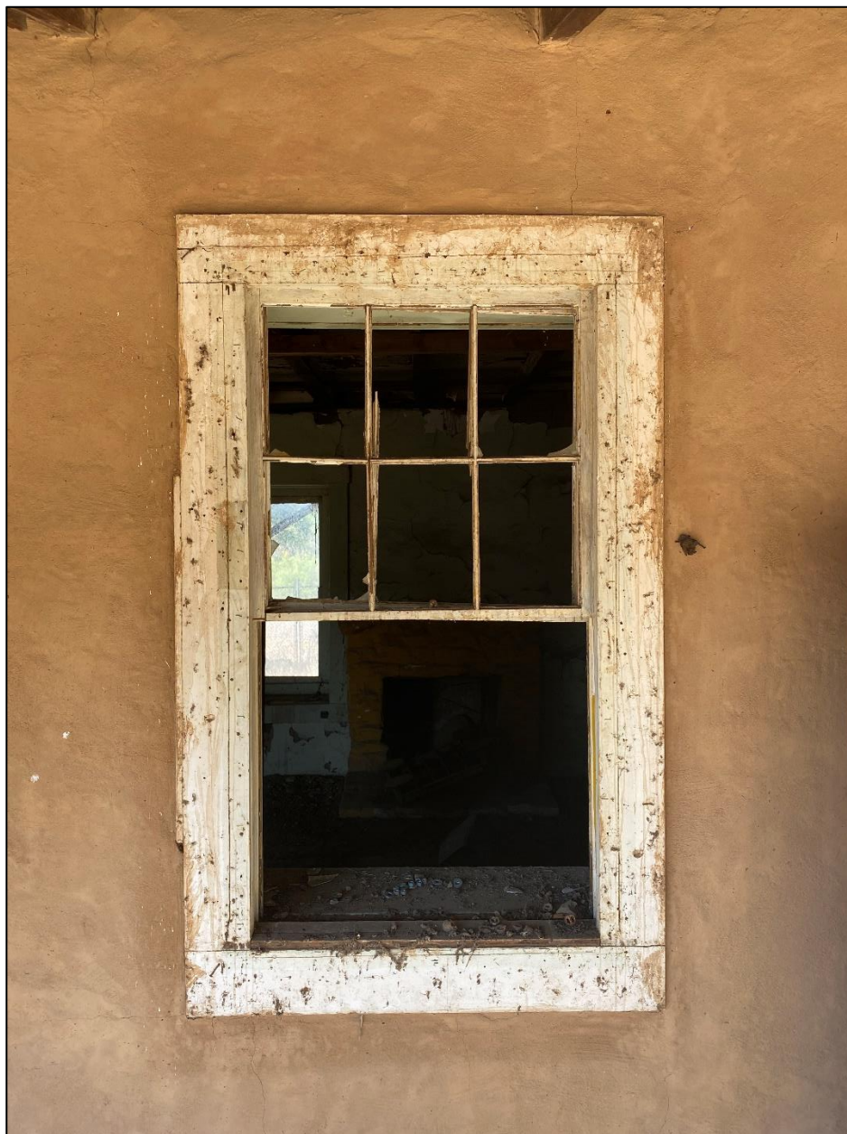
Figure 62. Example of a six-over-six, wood-sash, double-hung wood window that is missing muntins on the east side of the José María Gil Adobe, 2021. (ERDC-CERL.)
