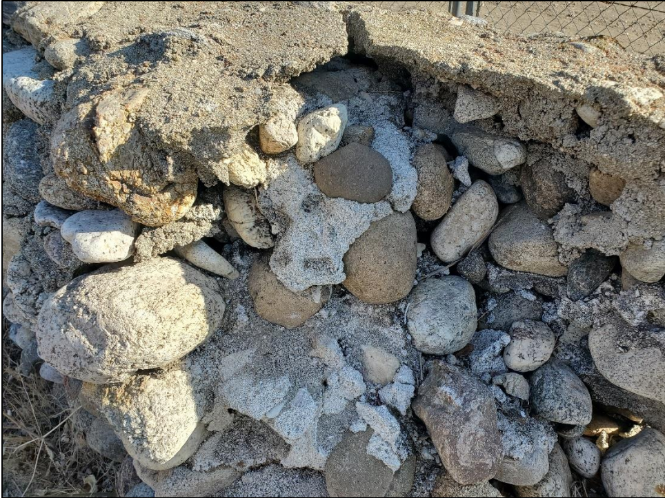
Figure 184. Inner mortar within stone wall (sample 2).
