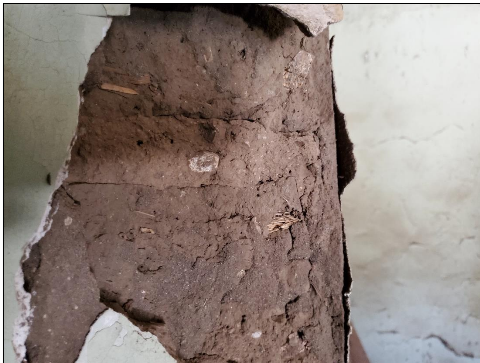
Figure 197. Bricks (sample 16a) in the east room having brown color and a low fraction of straw reinforcement.
