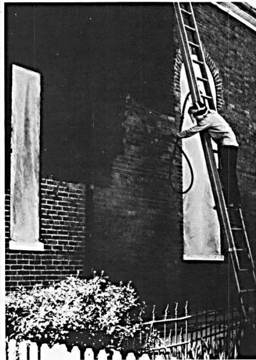
"Line Drop." Even though the operator of the sandblasting equipment is standing on a ladder to reach the higher sections of the wall, it is still almost impossible to have total control over the pressure. The pressure of the sand hitting the lower portion of the wall will still be greater than that above, because of the "line drop" in the distance from the pressure source to the nozzle. (Hugh Miller)
