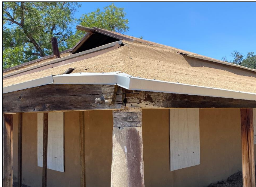
Figure 156. Aluminum drip edge that lines the edge of the roof of the José María Gil Adobe, 2021. (ERDC-CERL.)
