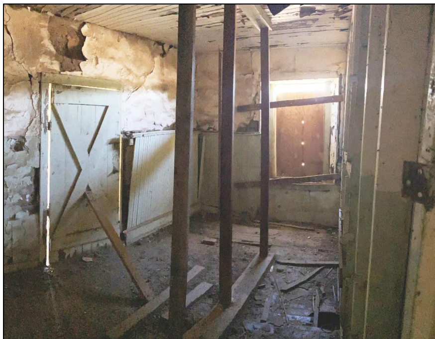
Figure 126. Beadboard wainscoting in the north wing of the José María Gil Adobe, 2021. (ERDC-CERL.)
