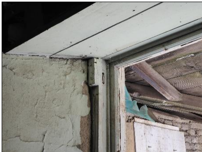
Figure 123. Wooden door header in the south wing of the José María Gil Adobe, 2021. (ERDC-CERL.)
