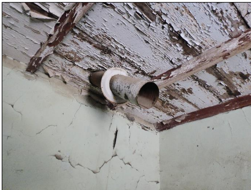
Figure 176. Metal stovepipe connection remaining in the south wing of the José María Gil Adobe, 2021. (ERDC-CERL.)
