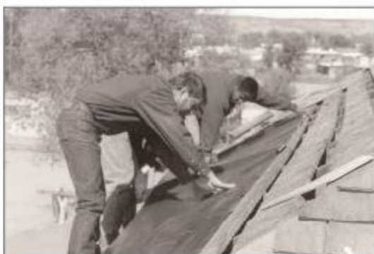
5. Carefully remove kraft paper from underside of the shield. Work from one end to the other. Carefully place the shield on roof surface.
