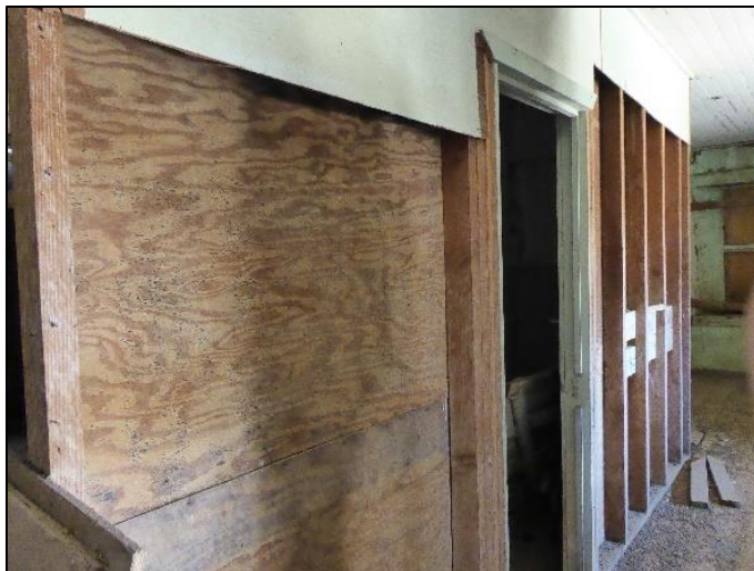
Figure 129. Wooden partition wall using plywood and studs, framing the bathroom space in the north wing of the José María Gil Adobe, 2021. (ERDC-CERL.)
