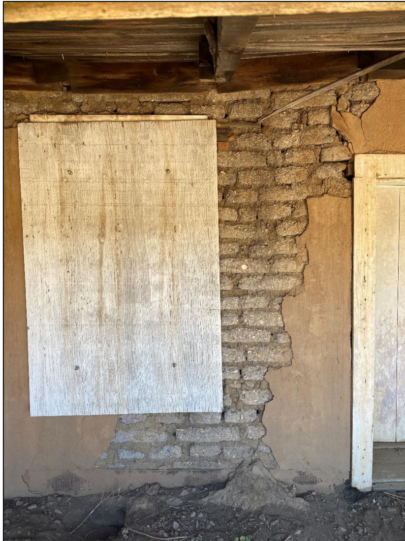
Figure 60. Plaster coating and exposed adobe brick on the north wing of the José María Gil Adobe, 2021. (ERDC-CERL.)
