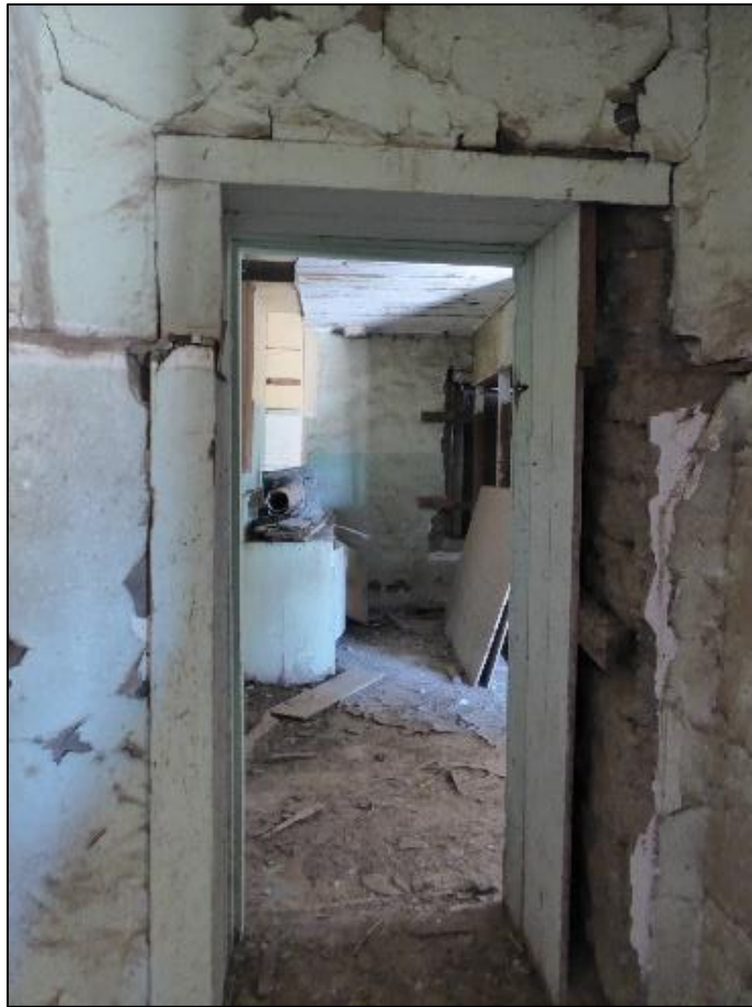
Figure 119. Interior wooden door trim with a missing board on the right side in the José María Gil Adobe, 2021. (ERDC-CERL.)
