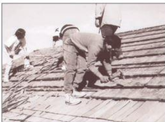
3. Drive in or pull out existing nails and repair or replace damaged purlins.
