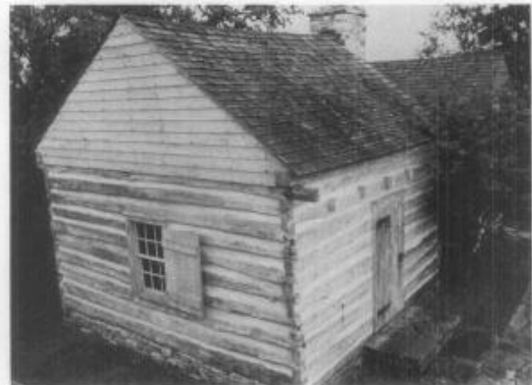
2. Handsplit and dressed shingles were also used on less elaborate buildings as seen in the restoration of the circa 1840 kitchen at the Winedale Inn, Texas. The uneven surfaces of the handsplit shingles were generally dressed or smoothed with a draw-knife to keep the rainwater from collecting in the wood grain and to ensure that the shingles lay flat on the sub-roof. Photo: Thomas Taylor.
