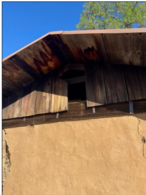
Figure 45. Vertically placed boards cladding the gable opening on the north and south sides of the cold storage building, 2021. (ERDC-CERL.)
