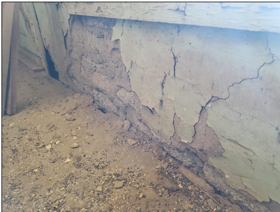
Figure 202. Coating, stucco (sample 11), and bricks in the west rooms.
