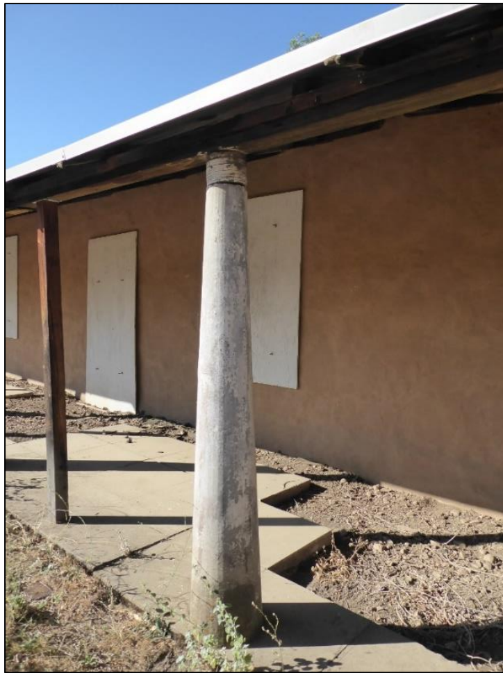
Figure 136. Intact concrete column on the northeast side of the José María Gil Adobe, 2021. (ERDC-CERL.)
