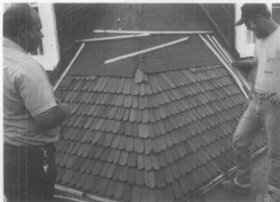
D. The fanned hips (seen here), swept valleys, and projecting ridge combs were installed as part of the re-roofing project. Special features, when documented, should be reproduced when re-shingling historic roofs.
