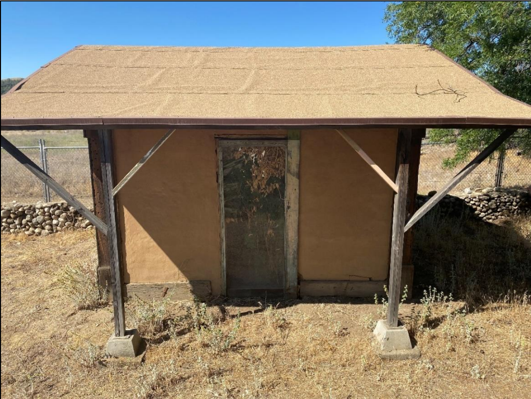
Figure 47. Wooden posts supporting front veranda of the cold storage building, 2021. (ERDC-CERL.)
