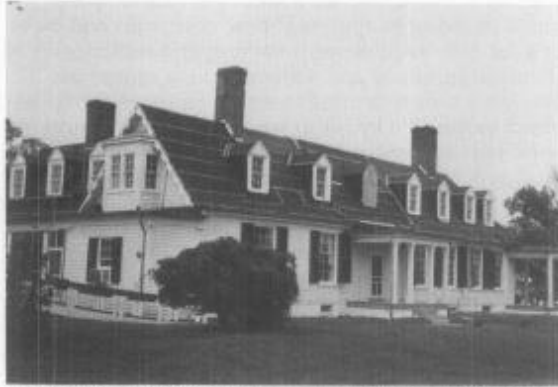
A. The later non-historic shingles were removed from Appomattox Manor (circa 1840 with later additions) and roofing paper was installed for temporary protection during the re-shingling.
