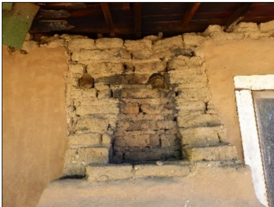
Figure 107. Circular posts imbedded into the south chimney of the José María Gil Adobe, 2021. (ERDC-CERL.)
