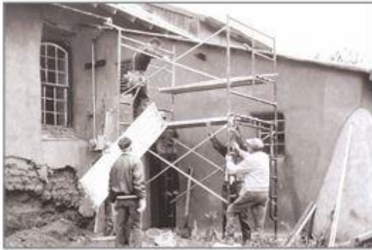
1. Set up scaffolding and equipment.
