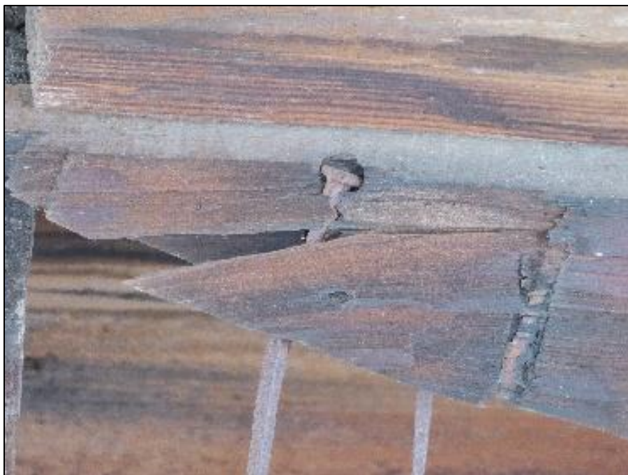
Figure 161. Rusted square nails on an exterior support frame of the José María Gil Adobe, 2021. (ERDC-CERL.)
