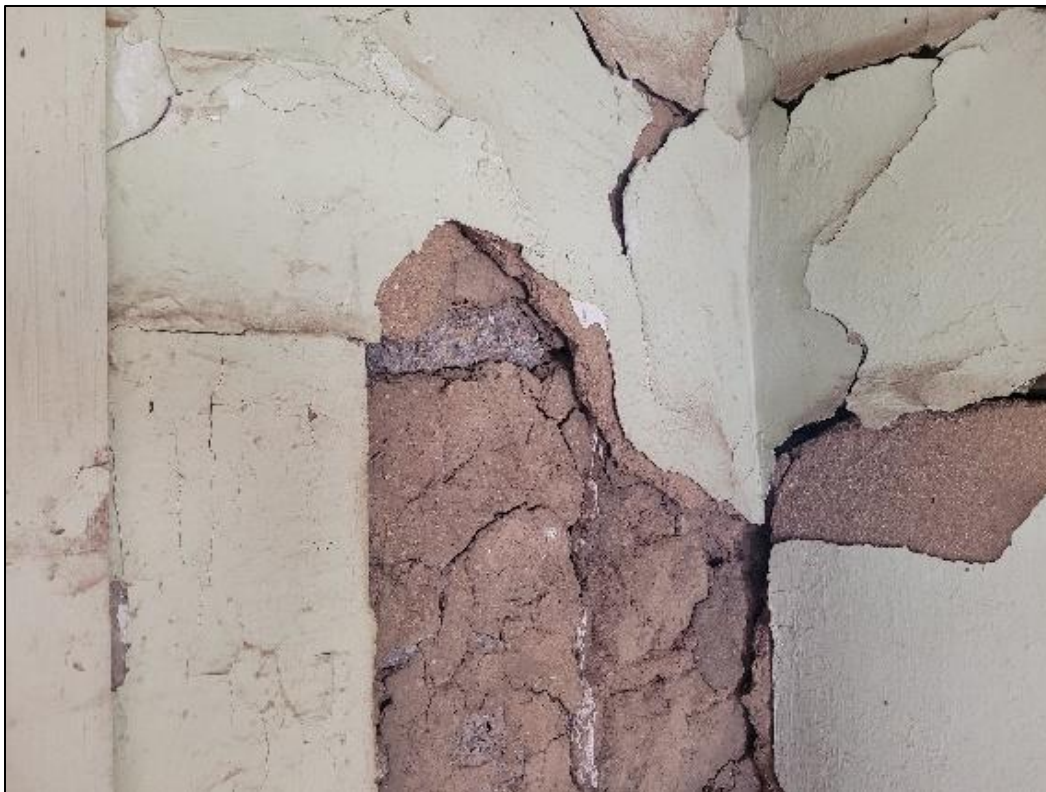
Figure 89. Cracked plaster and paint exposing adobe brick in the south wing of the José María Gil Adobe, 2021. (ERDC-CERL.)
