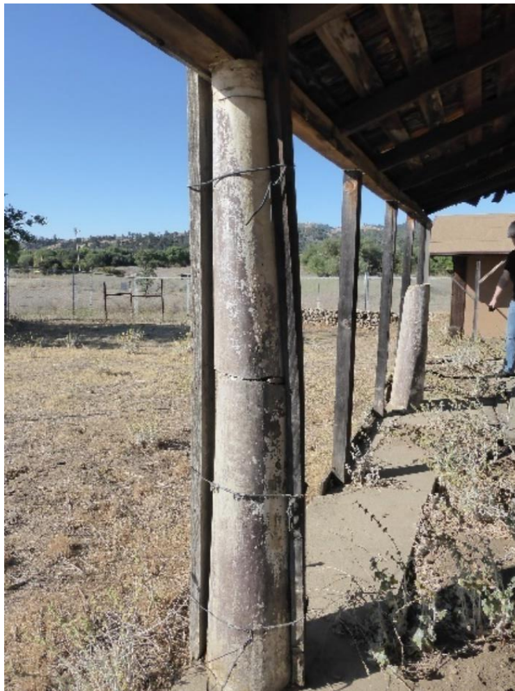
Figure 106. Two wooden 2 × 4 in. boards supporting a concrete column that is cracked in multiple places, 2021. (ERDC-CERL.)
