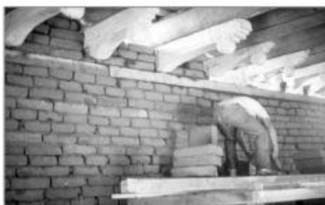
13. Infill between the corbels and vigas with adobe bricks and mud mortar.
