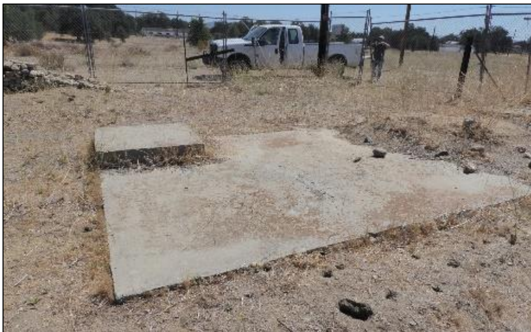
Figure 140. Concrete slab with raised square corners on the northeast side, approximately 25 ft east of the José María Gil Adobe, 2021. (ERDC-CERL.)
