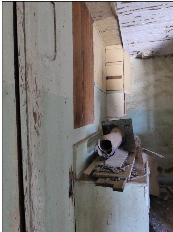
Figure 128. Wooden kitchen elements in the north wing of the José María Gil Adobe, 2021. (ERDC-CERL.)
