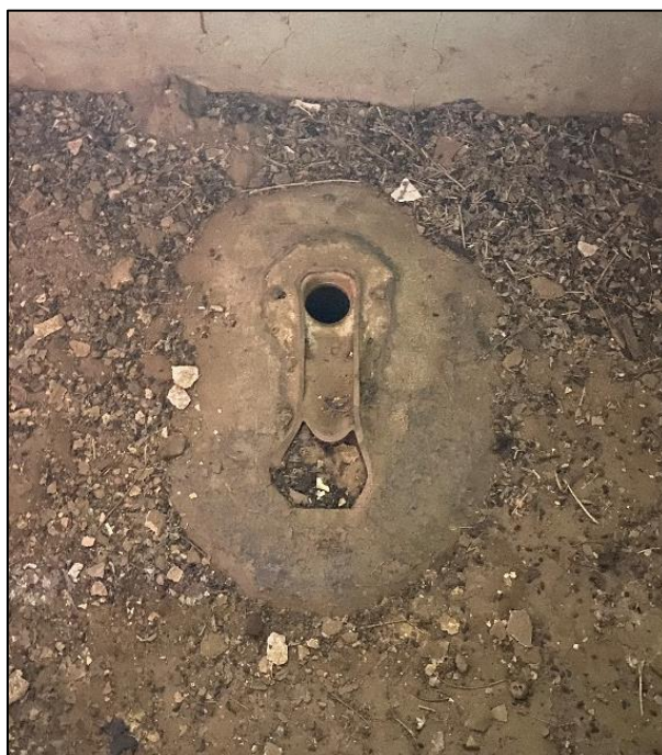
Figure 171. Metal toilet plumbing connection near the shower floors in the north wing of the José María Gil Adobe, 2021. (ERDC-CERL.)
