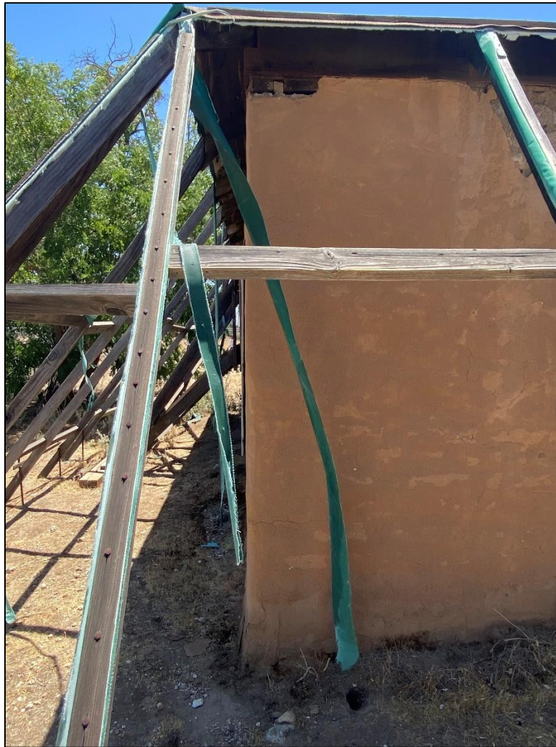
Figure 61. Uneven surface and flare of adobe wall at the base on the north corner of the José María Gil Adobe, 2021. (ERDC-CERL.)
