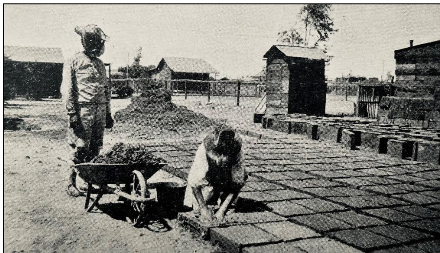
Figure 6. Making adobe brick and setting it in rows to bake in the sun, no date (Image reproduced from Long 1929. Public domain.)
