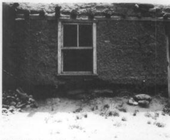
Coving. Salts deposited by rising ground water can evaporate and cause spalling of the adobe bricks at the base of the wall, a serious condition called "coving." Coving can also be caused and/or exacerbated by the erosion of rain splash. (National Park Service)
