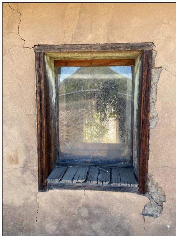
Figure 49. Wooden window trim and sill boards on the cold storage building, 2021. (ERDC-CERL.)
