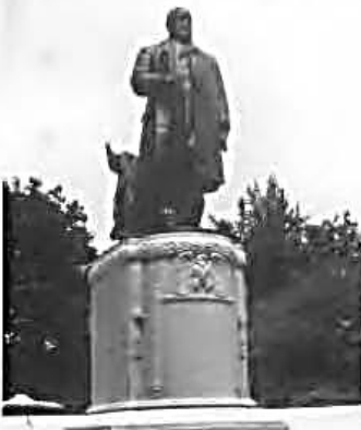
Figure 16. (a) The limestone base was heavily stained by runoff from the bronze statue above. (b) A poultice consisting of copper stain remover and ammonia mixed with fuller's earth was applied to the stone base and covered with plastic sheeting to keep it from drying out too quickly. (c) As the poultice dried, it pulled the stain out of the stone. (d) The poultice residue was removed carefully from the stone surface with wooden scrapers and the stone was rinsed with water. Photos: John Dwyer.
