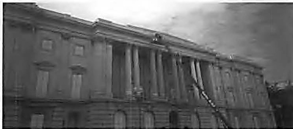
Figure 1. Low-to medium-pressure steam (hot-pressurized water washing), is being used to clean the exterior of the U.S. Tariff Commission Building, the first marble building constructed in Washington, D.C., in 1839. This method was selected by an architectural conservator as the "gentlest means possible" to clean the marble. Steam can soften heavy soiling deposits such as those on the cornice and column capitals, and facilitate easy removal. Note how these deposits have been removed from the right side of the cornice which has already been cleaned.
