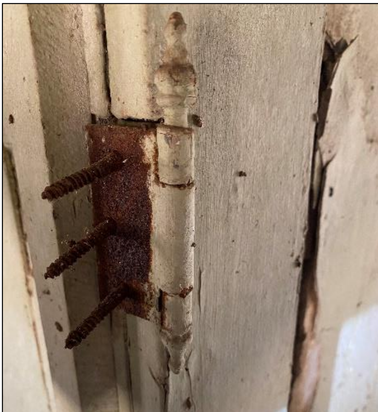
Figure 173. Stylistic metal door hinges that remain on interior doors of the José María Gil Adobe, 2021. (ERDC-CERL.)
