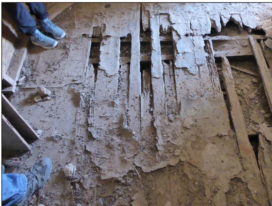
Figure 113. Wood strip flooring with breakthrough areas in a central location of a floor in the José María Gil Adobe, 2021. (ERDC-CERL.)
