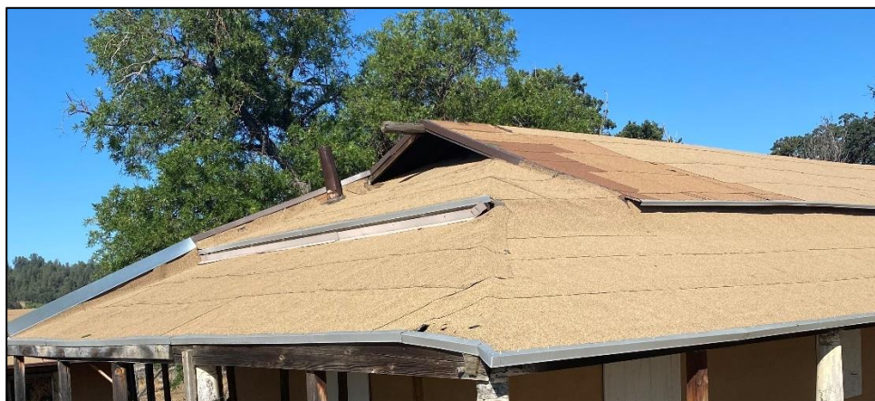
Figure 56. Multiple layers of roofs on the south end of the José María Gil Adobe, 2021. (ERDC-CERL.)
