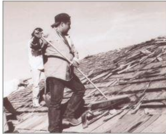
2. Sweep and clean the roof surface.
