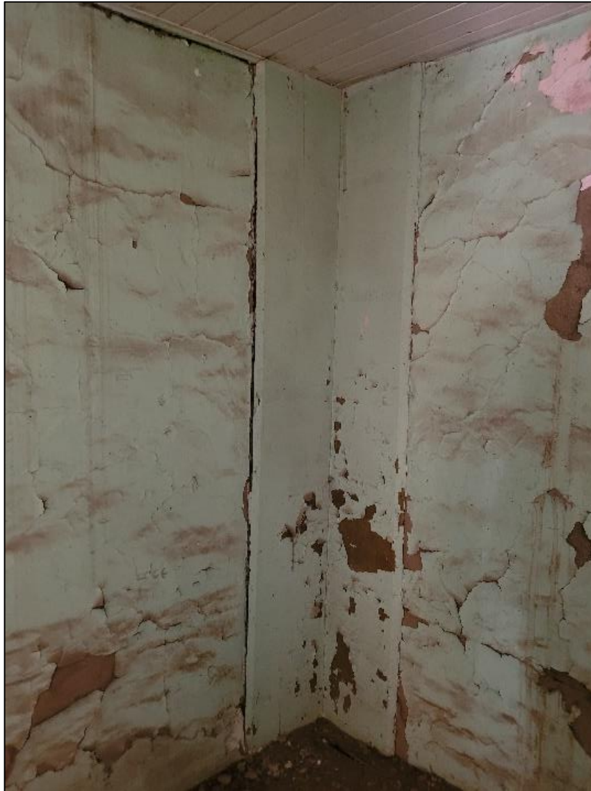
Figure 131. Floor to ceiling wooden element in the northmost corner of the José María Gil Adobe, 2021. (ERDC-CERL.)
