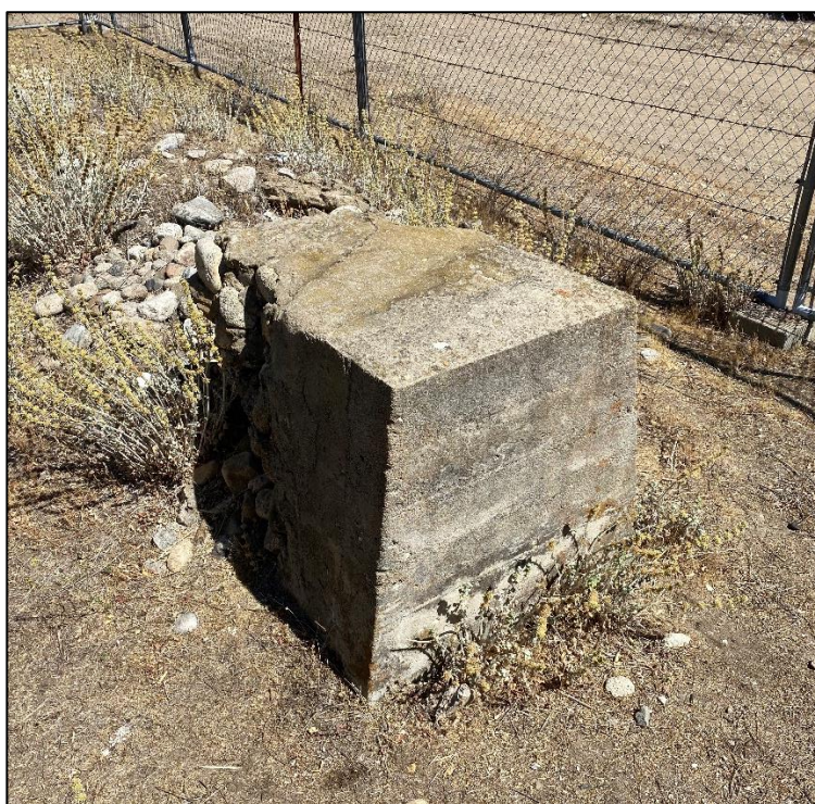
Figure 141. Cast-concrete entrance pillars attached to cobblestone wall near the north corner of the site of the José María Gil Adobe, 2021. (ERDC-CERL.)
