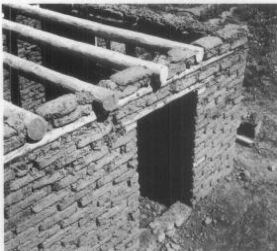
Roof Bearing. A roof bearing timber placed within the adobe walls provides even support for the weight of the roof. (Farm Security Administration Collection, Library of Congress)
