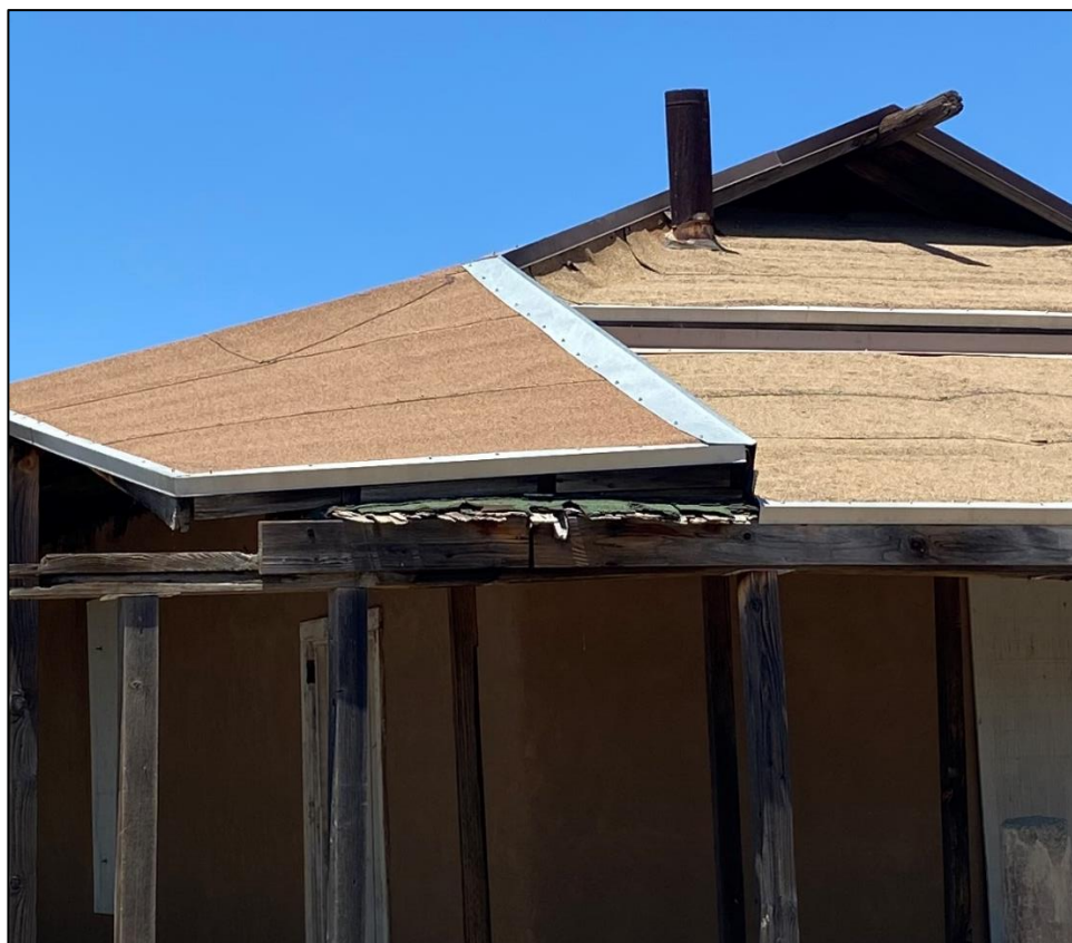
Figure 55. Multiple roof layers showing green asphalt shingles and brown asphalt paper on the south corner of the José María Gil Adobe, 2021. (ERDC-CERL.)
