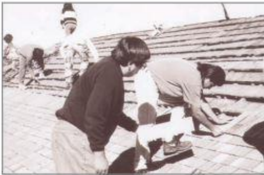
13. Continue the process of placing shingles.
