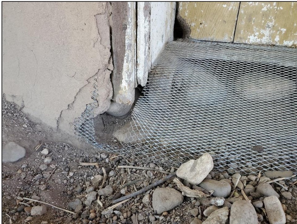
Figure 192. Stucco on wire lath (sample 17b) over different color stucco having better edge quality (sample 18.)
