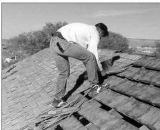
1. Remove existing shingles if any.
