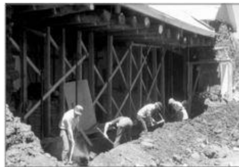
2. Remove fallen wall material.
