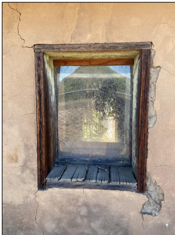
Figure 41. Plexiglass in the window opening on the southwest side of the cold storage building, 2021. (ERDC-CERL.)
