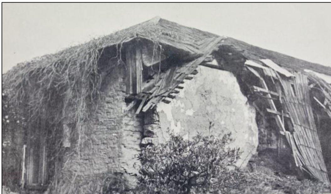
Figure 17. Roofing material crumbling at the corner of the Ignacio Palomares Adobe and plants growing into the wooden roof, no date. (Image reproduced from Giffen 1955, 84. Public domain.)
