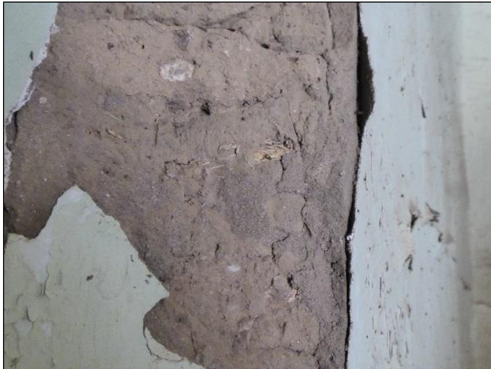
Figure 91. Intact plaster with peeling paint in the south wing of the José María Gil Adobe, 2021. (ERDC-CERL.)
