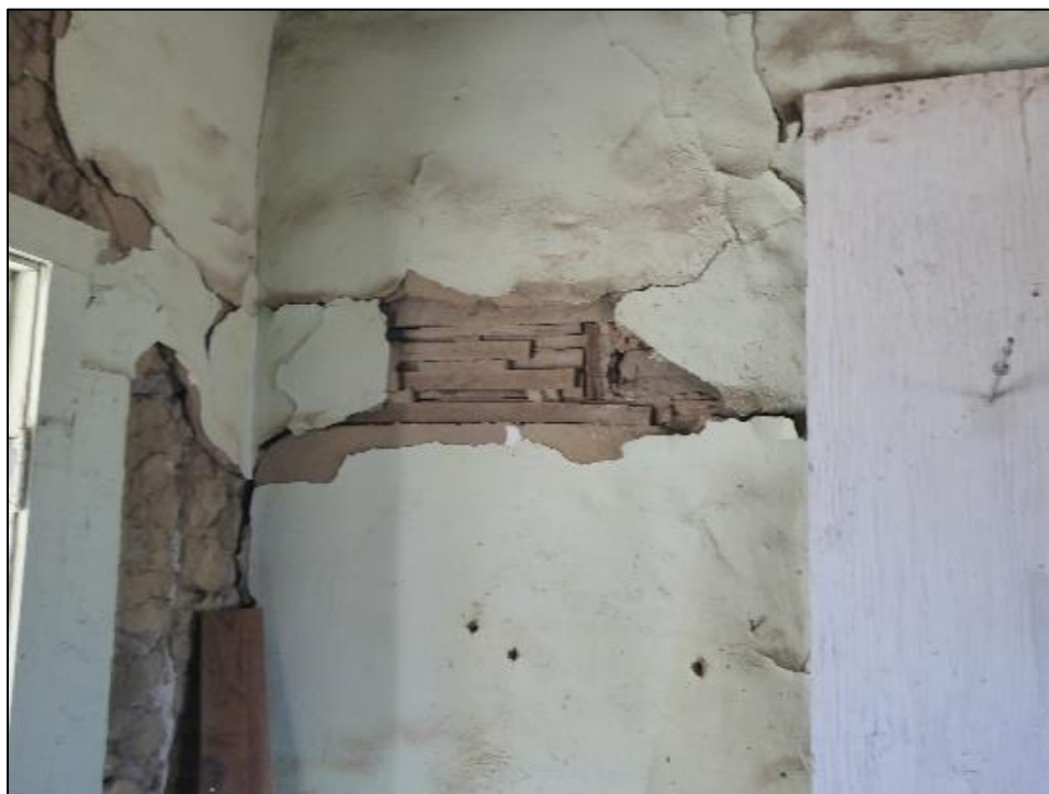
Figure 90. Cracked plaster and paint exposing wooden elements in the south wing of the José María Gil Adobe, 2021. (ERDC-CERL.)
