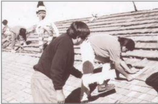
13. Continue the process of placing shingles.
