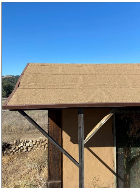
Figure 42. Brown asphalt paper on the roof of the cold storage building, 2021. (ERDC-CERL.)
