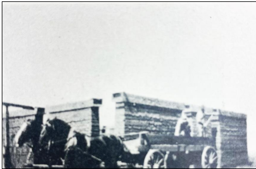
Figure 4. An adobe wall with 1 × 10 in. wooden forms on a high layer, showing the poured adobe construction method, no date (Image reproduced from Long 1929. Public domain.)
