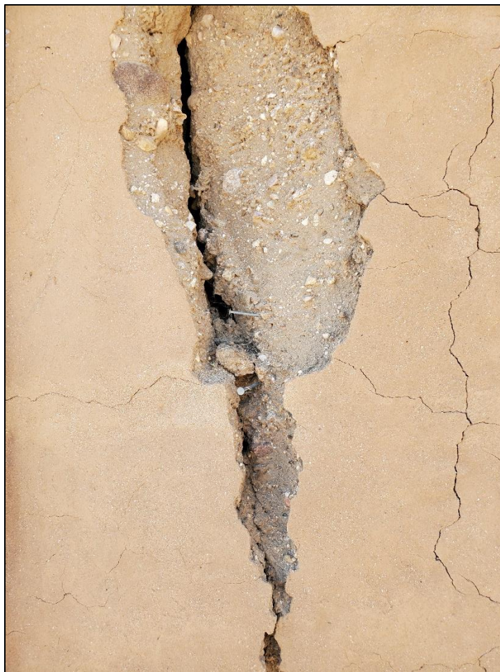
Figure 205. Outbuilding earthen wall and stucco with reinforcing nails.
