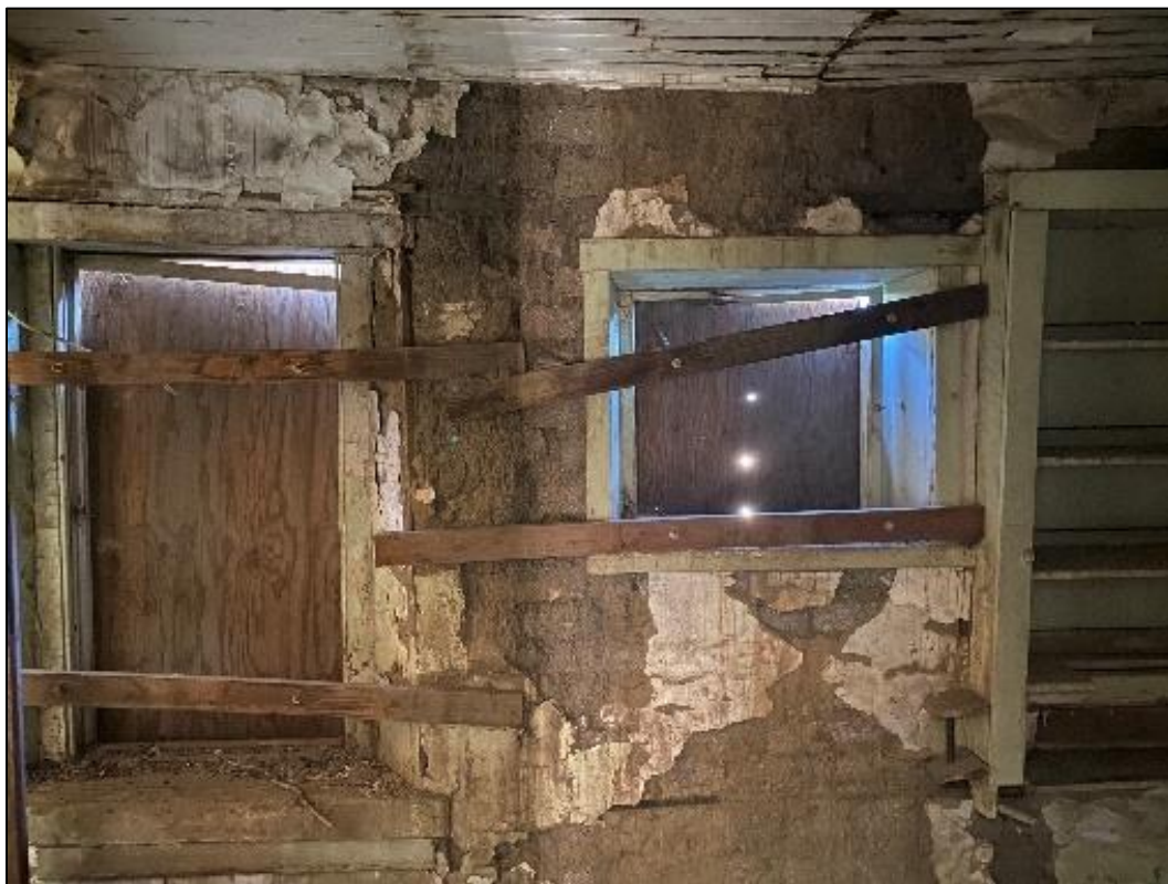
Figure 118. Crooked and various-sized window trim in the north wing of the José María Gil Adobe, 2021. (ERDC-CERL.)
