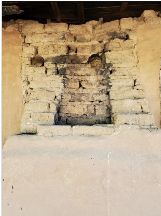
Figure 191. Two stuccos ( top and bottom ) (samples 17b and 18) of different color and edge quality on the south exterior wall, indicating different time periods of application.
