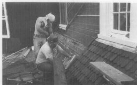
E. In order to achieve a "Class B" fire-rating, the shingles were dipped in fire-retardant chemicals and allowed to dry prior to installation. Iron oxide was added to this chemical dip to stain the shingles to match the historic red color. These coatings will need periodic reapplication.
