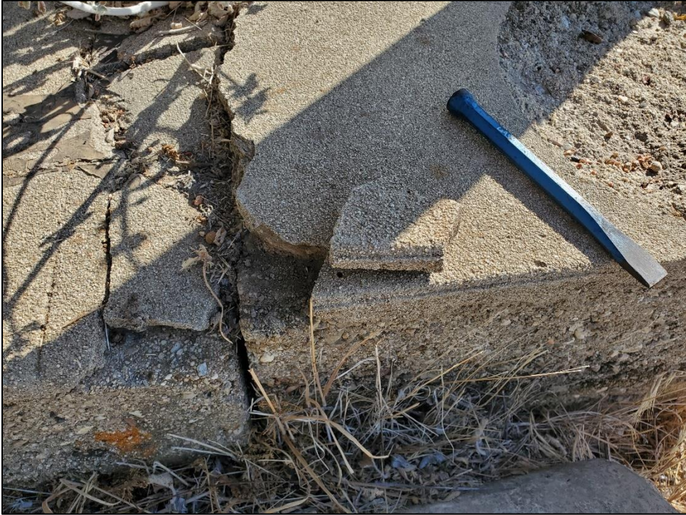
Figure 185. Tile surrounding main structure (sample 3).
