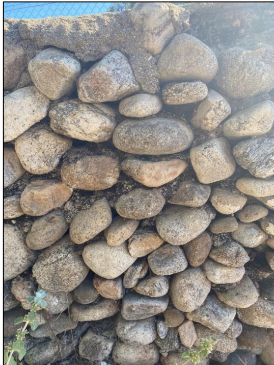
Figure 149. Various sizes of cobblestone making up the perimeter wall of the site of the José María Gil Adobe, 2021. (ERDC-CERL.)
