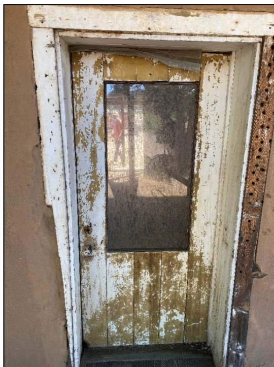
Figure 64. Exterior door type with vertical boards and a window on the northwest side of the José María Gil Adobe, 2021. (ERDC-CERL.)
