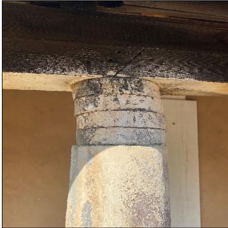
Figure 105. Wooden disks on top of the concrete columns supporting the veranda roof, possibly for leveling purposes, on the José María Gil Adobe, 2021. (ERDC-CERL.)
