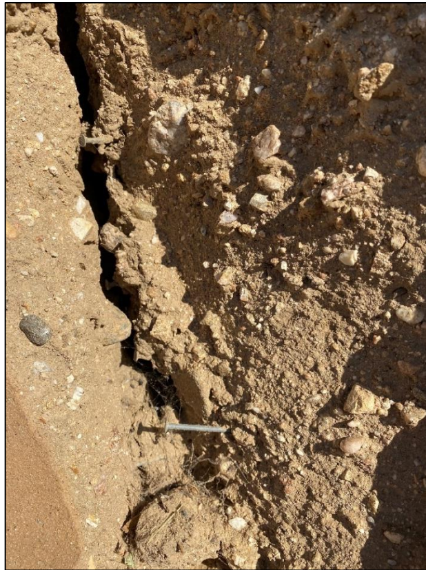
Figure 43. Rammed earth material exposed in crack on the southeast side of the cold storage building, 2021. (ERDC-CERL.)
