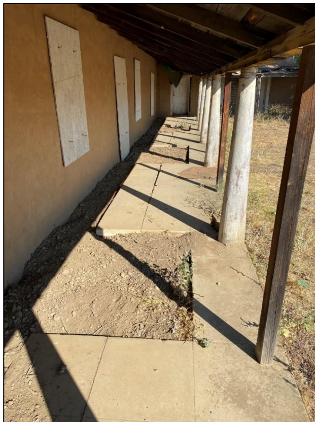
Figure 132. Concrete pavers lining the northeast side of the José María Gil Adobe, 2021. (ERDC-CERL.)
