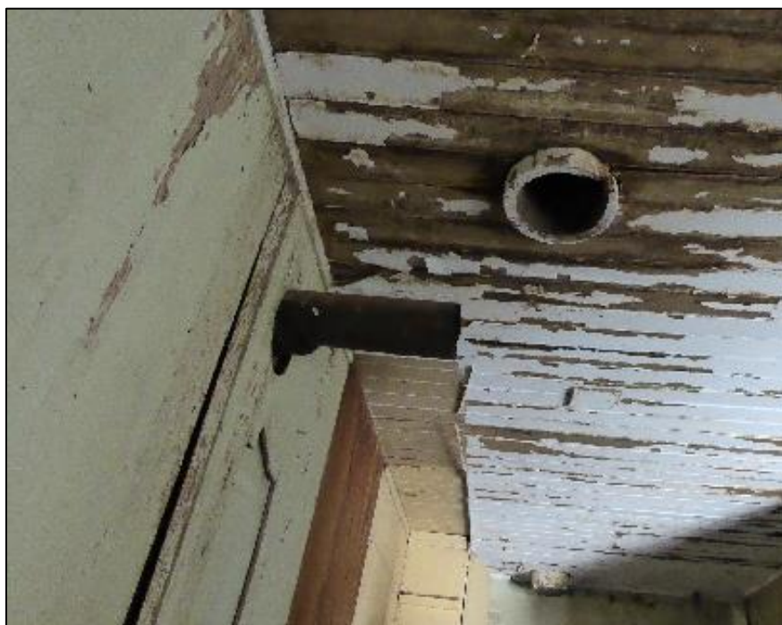
Figure 177. Metal stovepipe connection remaining on a wall and a chimney pipe remaining in the ceiling in the north wing of the José María Gil Adobe, 2021. (ERDC-CERL.)
