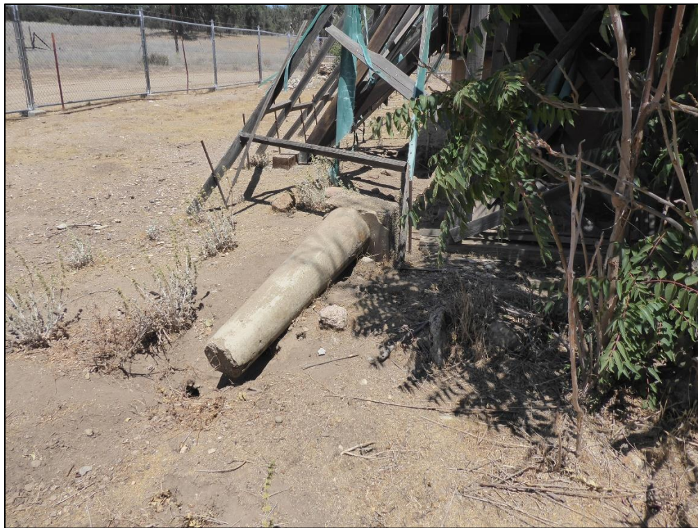
Figure 139. Concrete column tipped over with base still attached on the northwest corner of the José María Gil Adobe, 2021. (ERDC-CERL.)
