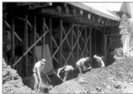
2. Remove fallen wall material.
