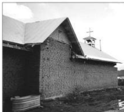
14. Apply a mud plaster when the wall has been completed (see Mud Plastering below).
