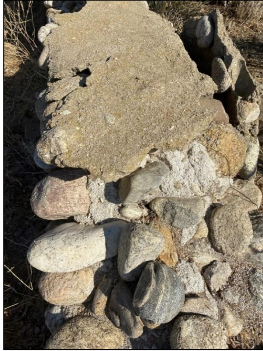
Figure 148. Smeared concrete surface on top of the cobblestone wall along the perimeter of the site of the José María Gil Adobe, 2021. (ERDC-CERL.)
