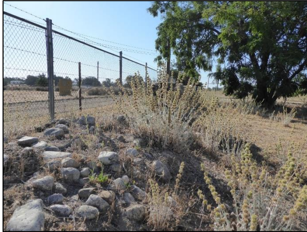
Figure 150. Crumbled and scattered cobblestone wall on the east side of the site of the José María Gil Adobe, 2021. (ERDC-CERL.)
