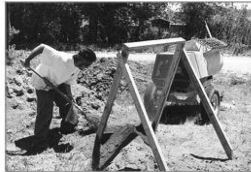
2. Screen the soil. Do not screen the soil if wet. (See Building a Screen at the end of this section.)
