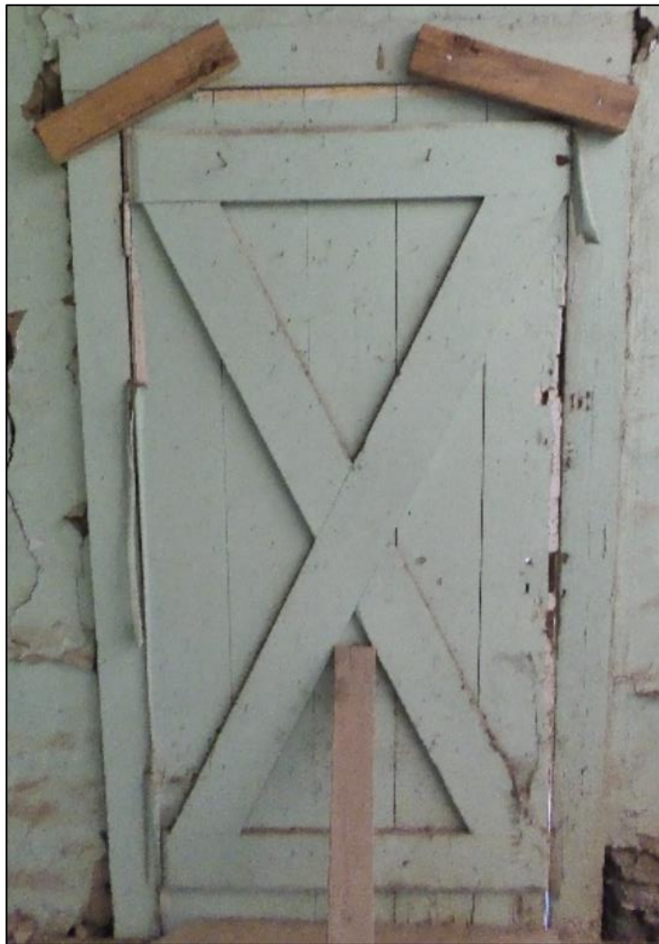
Figure 101. X-brace pattern on the inside of the main exterior door type on the José María Gil Adobe, 2021. (ERDC-CERL.)
