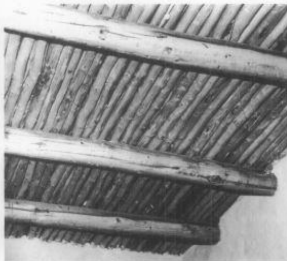
Roof Framing. Viga logs and savinos are seen in the interior of the adobe building. Often the wooden materials that compose the traditional flat adobe roof create interesting and pleasing patterns on the ceilings of the interior rooms. (Photo by Russell Lee, Farm Security Administration Collection, Library of Congress)
