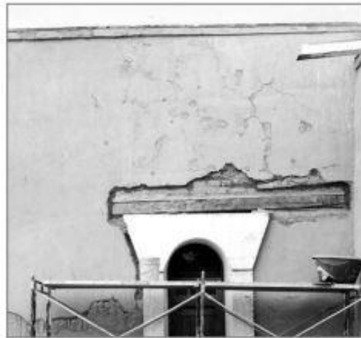
Lintel repair and replacement was an important part of the preservation project completed in 2005 at the mid-19th century mission at Socorro, Texas. (Pat Taylor, 2004)
