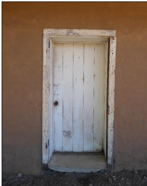
Figure 63. Exterior door type with vertical boards on the southwest side of the José María Gil Adobe, 2021. (ERDC-CERL.)
