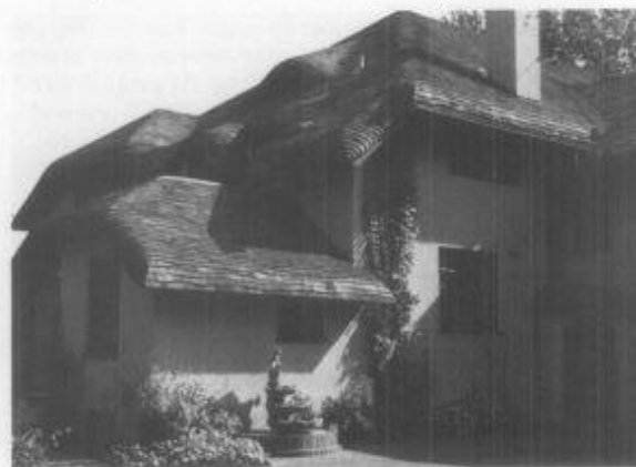
4. With the popularity of the revival of historic styles in the late 19th and early 20th centuries, a new technique was developed to imitate English thatch roofs. For the Tudor Revival thatch cottages, steaming and curving of sawn shingles provided an undulating pattern to this picturesque roof shape. Photo: Courtesy of C.H. Roofing.
