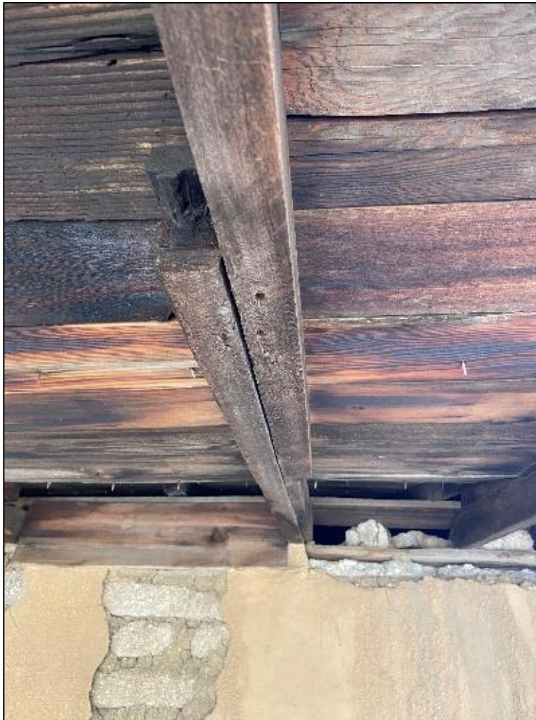
Figure 95. Looking at the connection between the veranda roof to the roof of the José María Gil Adobe, 2021. (ERDC-CERL.)
