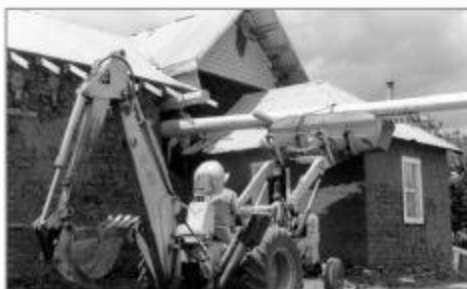
12. Replace vigas that cannot be spliced or repaired with new ones to match the existing. Slide the viga through one side of the building to the other then set the viga on the corbel (see Part Three, Repairing Vigas and Corbels ).
