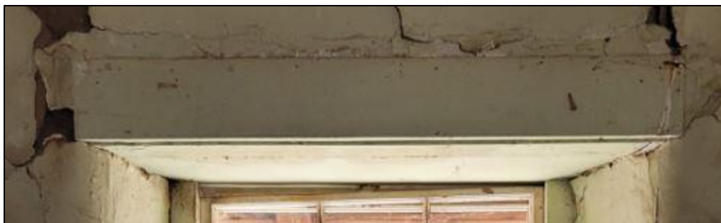
Figure 121. Wooden window header covered with wooden trim in the south wing in the José María Gil Adobe, 2021. (ERDC-CERL.)
