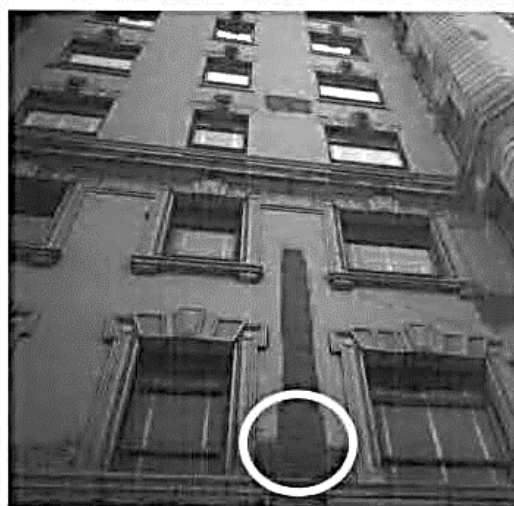
Figure 3. This small test area has revealed a red brick patch that does not match the original beige brick. This may explain why the building was painted, and may suggest to the owner that it may be preferable to keep it painted.
