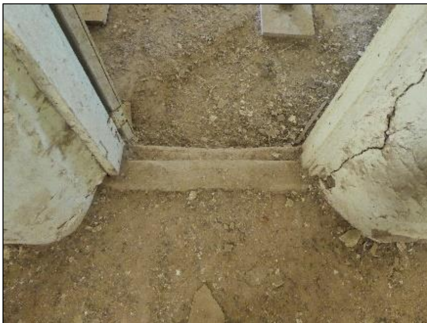
Figure 124. Wooden threshold transition between two rooms in the south wing of the José María Gil Adobe, 2021. (ERDC-CERL.)
