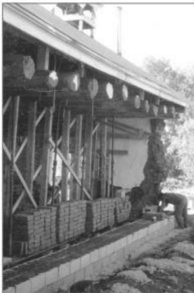
1. Shore up roof prior to work (see Part One, Emergency Shoring ).
