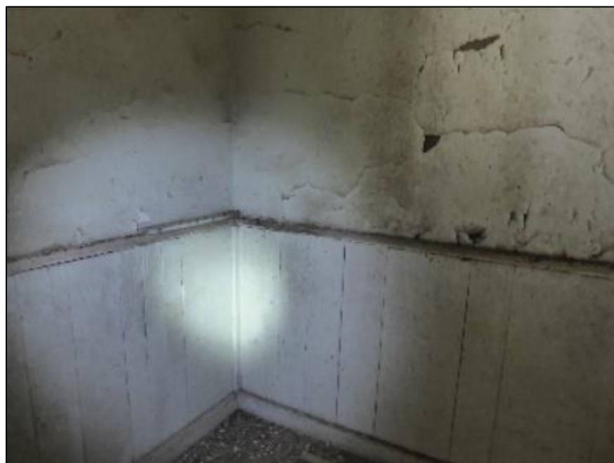
Figure 127. Various-sized plank wainscoting with a chair rail in the south wing of the José María Gil Adobe, 2021. (ERDC-CERL.)
