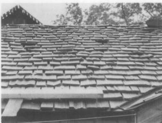
15. These commercially available roofing products with rustic split faces are not appropriate for historic preservation projects. In addition to the inaccurate appearance, the irregular surfaces and often wide spaces between shingles will allow wind-driven moisture to penetrate up and under them. The excessively wide boards will tend to cup, curl and crack. Moss, lichens and debris will have a tendency to collect on these irregular surfaces, further deteriorating the roofing. Photo: Sharon C. Park.
