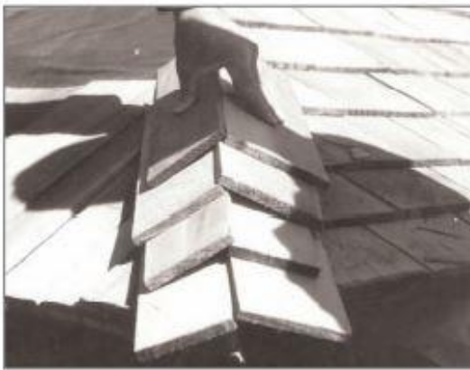
15. At the hip each side of the shingle overlaps in an alternating fashion.
