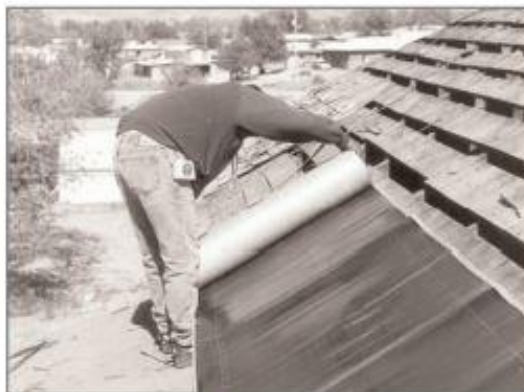
4. Ice and water shield should be installed on all overhangs. Roll out shield, cut to a workable length, and cut to fit at the hip if a hip exists.
