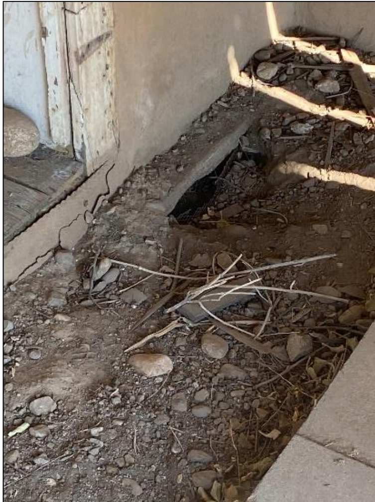
Figure 103. Wooden sill supporting the base of the adobe wall at grade level of the José María Gil Adobe, 2021. (ERDC-CERL.)
