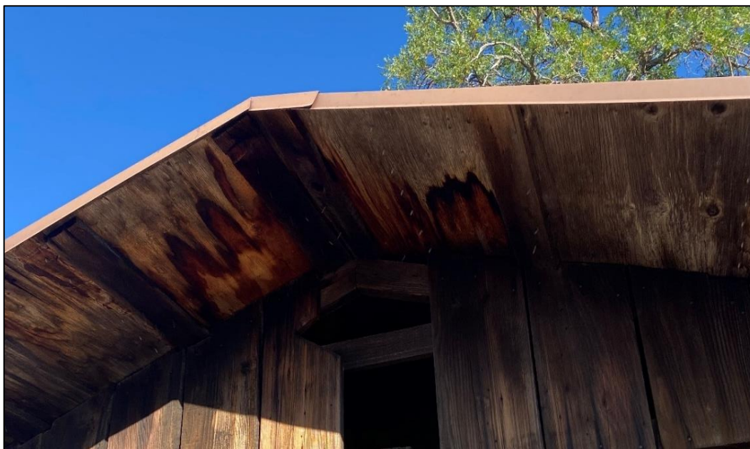
Figure 46. Wooden soffits under the roof overhang of the cold storage building, 2021. (ERDC-CERL.)
