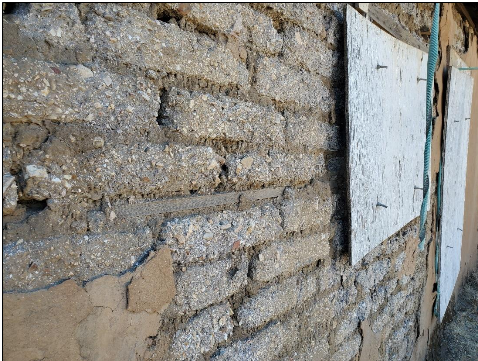
Figure 186. West exterior wall bricks (sample 15) and mortar (sample 13.)
