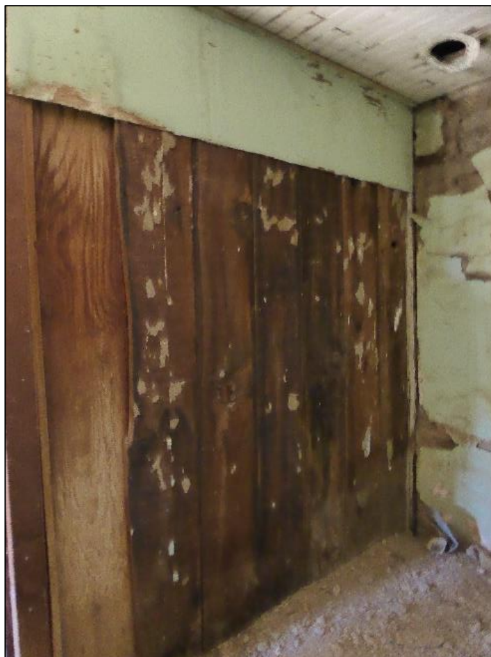
Figure 130. Wood plank portion of the partition wall in the north wing of the José María Gil Adobe, 2021. (ERDC-CERL.)
