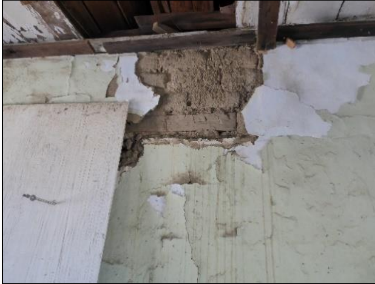
Figure 125. Wooden element embedded within the adobe wall in the south wing of the José María Gil Adobe, 2021. (ERDC-CERL.)
