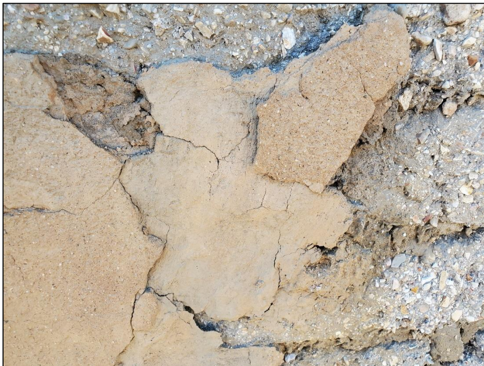
Figure 190. West exterior wall stucco (sample 14.)
