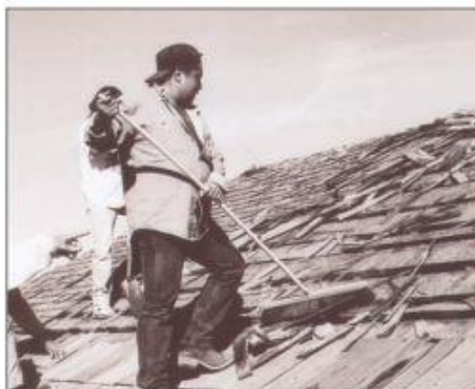
2. Sweep and clean the roof surface.
