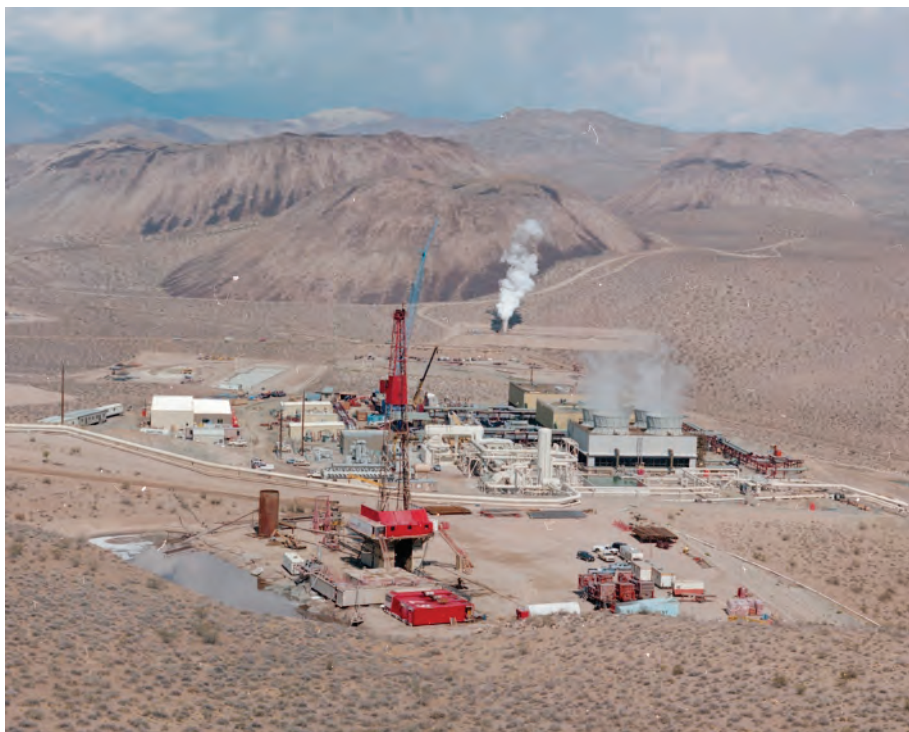
Navy Geothermal Plant One.
