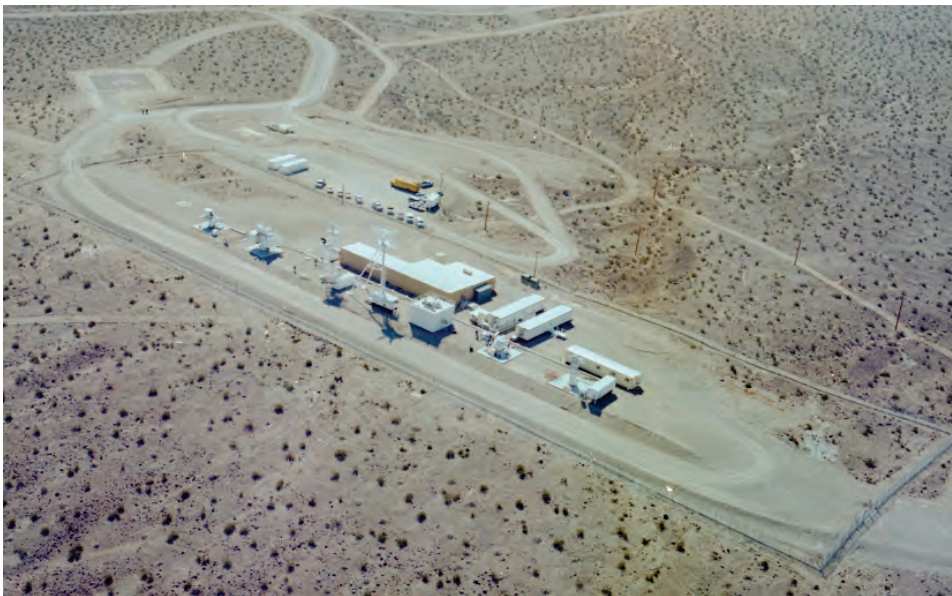
Aerial view of Sea Site, Echo Range.
