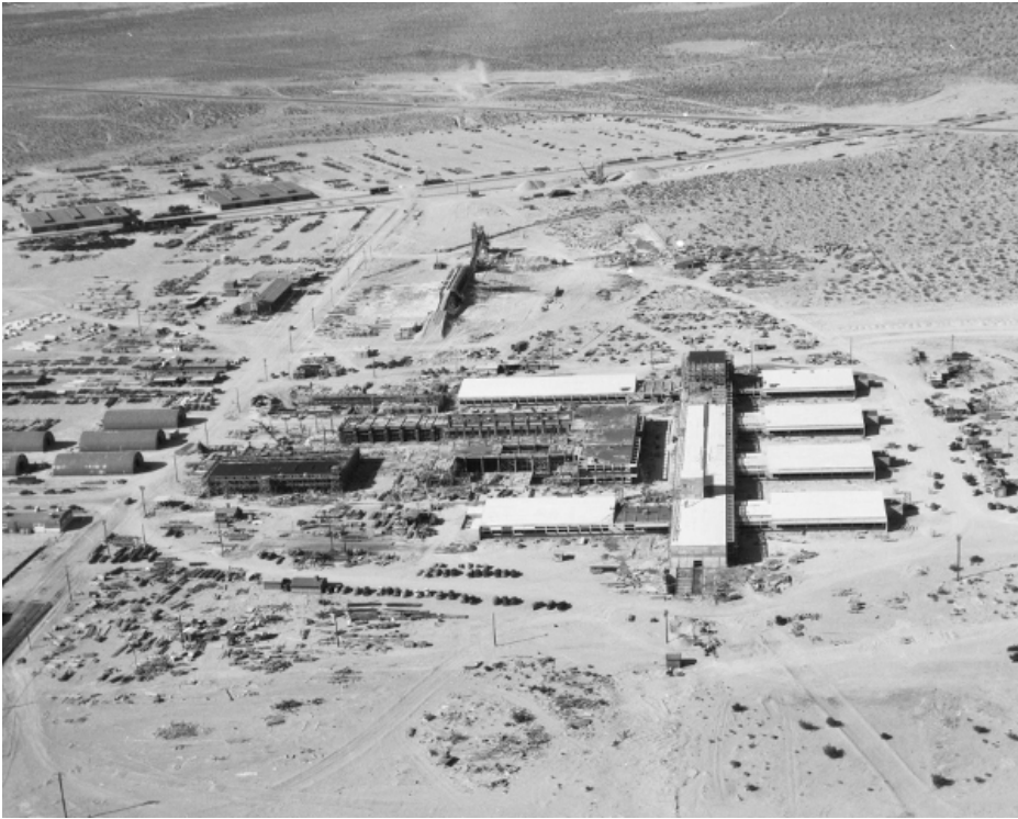
Michelson Laboratory under construction, 1946.
