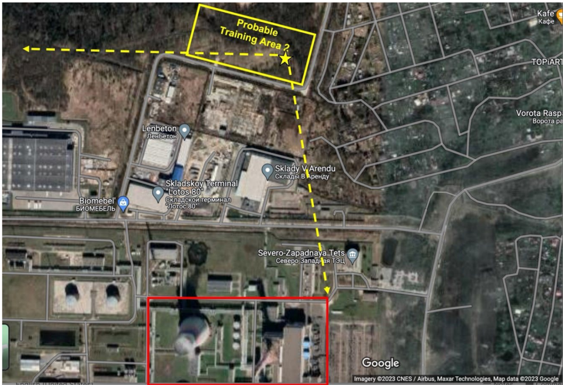
Figure 11. Overhead Perspective of Olgino Power Plant from the North in Training Area 2. 414
