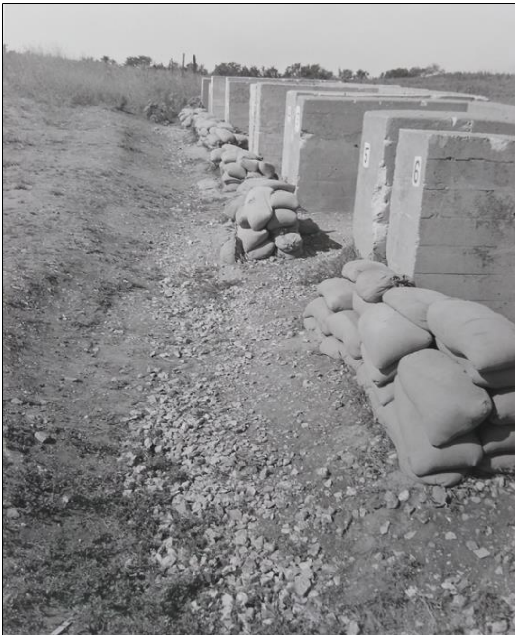
Figure 55. Protective trench on hand grenade range (range 25) and board-formed concrete pits, 13 July 1966. (RG 111-SCA Album 528D, 631509, Riley—Views, Signal Corps Photographs between 1941 and 1954, RG 111, NARA, College Park, MD. Public domain.)
