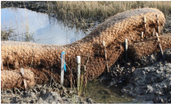
c. Coir logs, Avalon, New Jersey Source: Timothy Welp, ERDC
