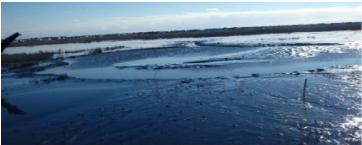
Figure 5.5. Scour Hole at the Base of a Dredge Pipeline Discharge
