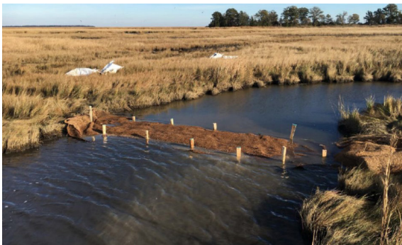
a. Coir mat filled with sand, Blackwater NWR Source: Albert McCollough, Sustainable Science
