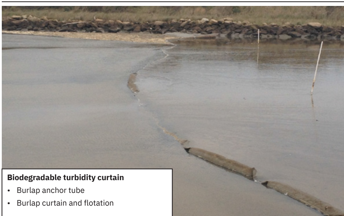
Figure 4.14. Biodegradable Burlap Silt Curtain at the Gaillard Island Disposal Facility
