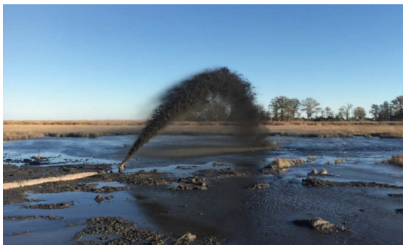
c. Blackwater NWR, Maryland high-pressure (ground-mounted nozzle) discharge Source: Albert McCollough, Sustainable Science
