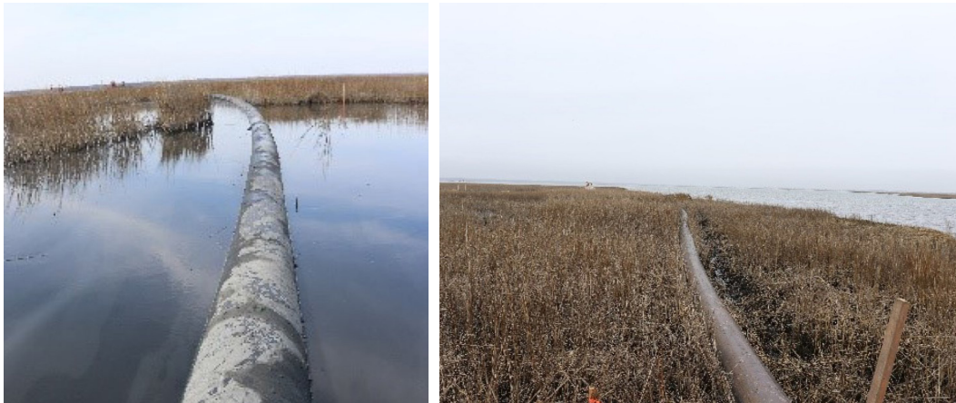
a. Use of dredge's HDPE active discharge pipeline
