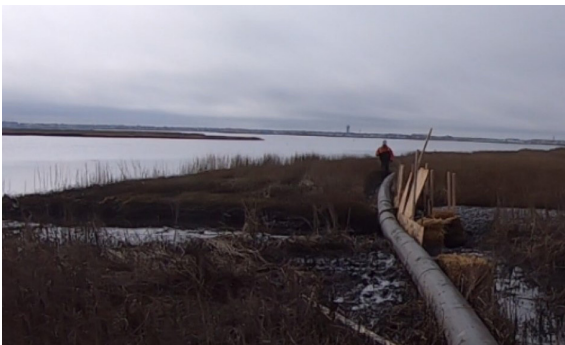
b. Dredge pipeline, Sturgeon Island, New Jersey Source: Timothy Welp, ERDC
