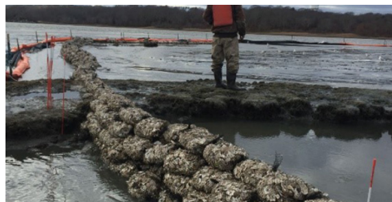
d. Clam and oyster shell bags, John H. Chafee NWR Source: TNC
