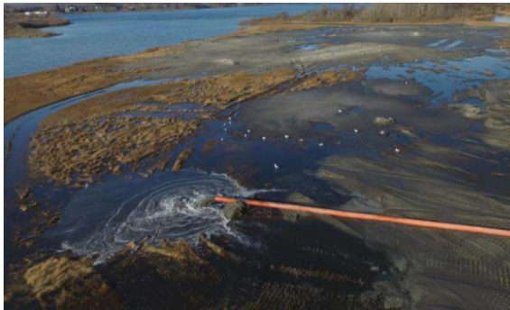
a. John H. Chafee NWR, Rhode Island low-pressure (naked) discharge Source: USFWS
