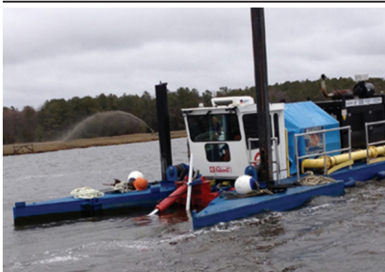
a. Pepper Creek, Delaware 10-in (25.4 cm) swinging ladder cutterhead dredge
