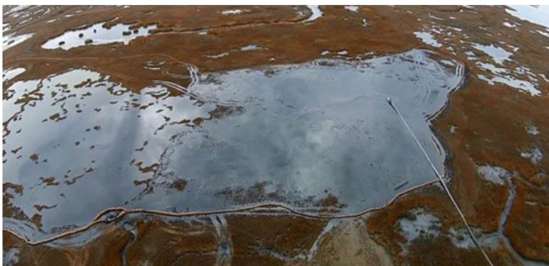
Figure 5.4. Avalon (New Jersey) Phase II DM Placement with a Low-Pressure (Spreader Plate) Discharge
