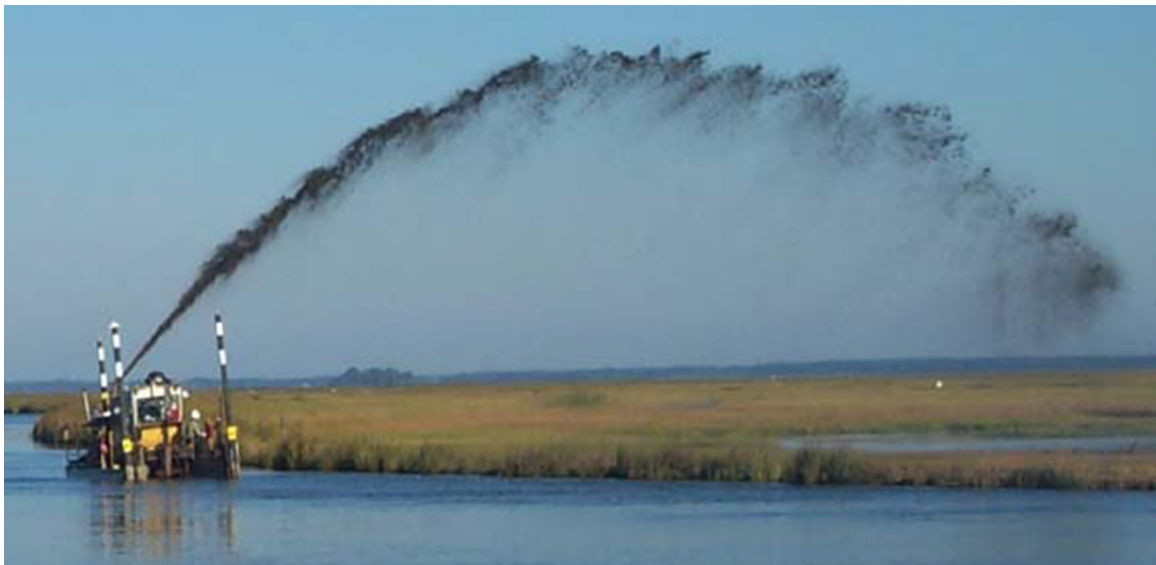
Figure 1.1. High-Pressure TLP of DM on Wetlands
