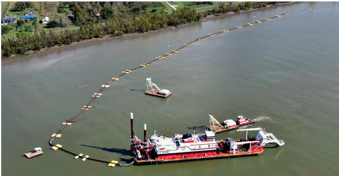
Figure 5.12. Cutterhead Dredge and Tailpipe for Open-Water TLP
