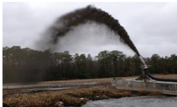
d. Pepper Creek, Delaware high-pressure (barge-mounted nozzle) discharge Source: DNREC
