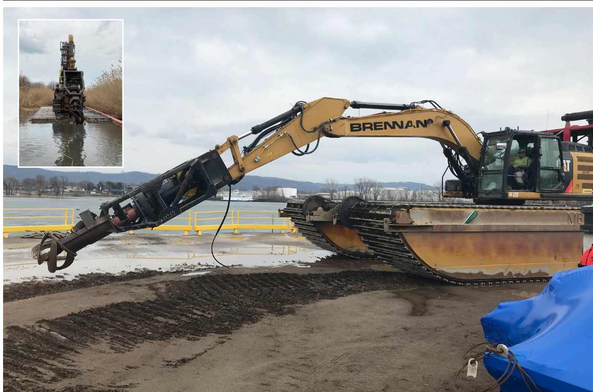
Figure 5.2. Submersible Pump with Cutterhead Attached to a Hydraulic Excavator
