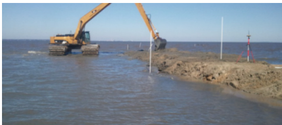
e. Earthen containment dike, Gaillard Island, Alabama Source: Nate Lovelace
