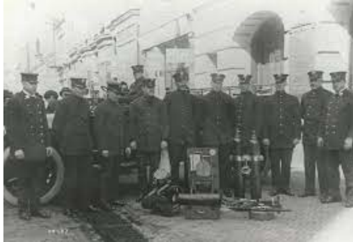
Figure 1. Original Fire Equipment and Apparatus. 96
