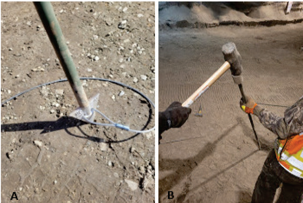
Figure 4-6. Arrowhead anchor installation. (A) Drive rod nested against arrowhead. (B) Two operators needed to install.
