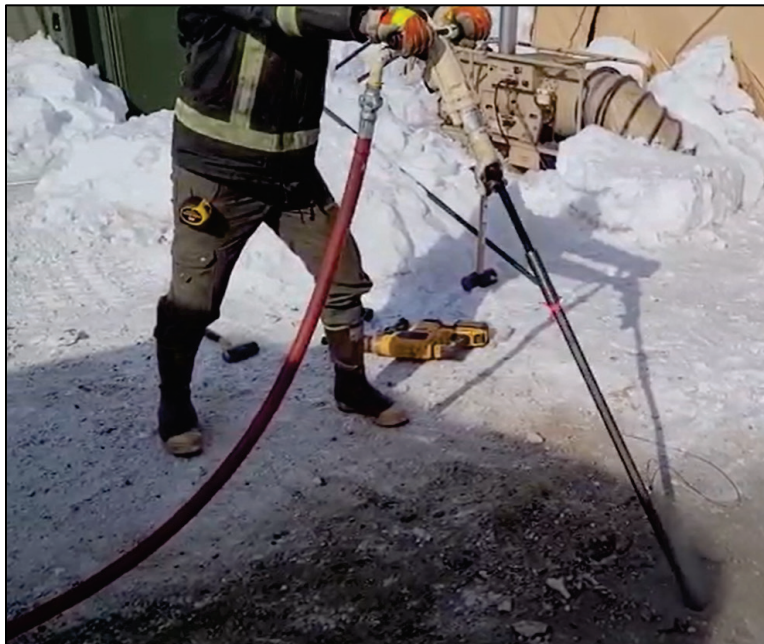
Figure 4-4. Drilling in frozen gravels.
