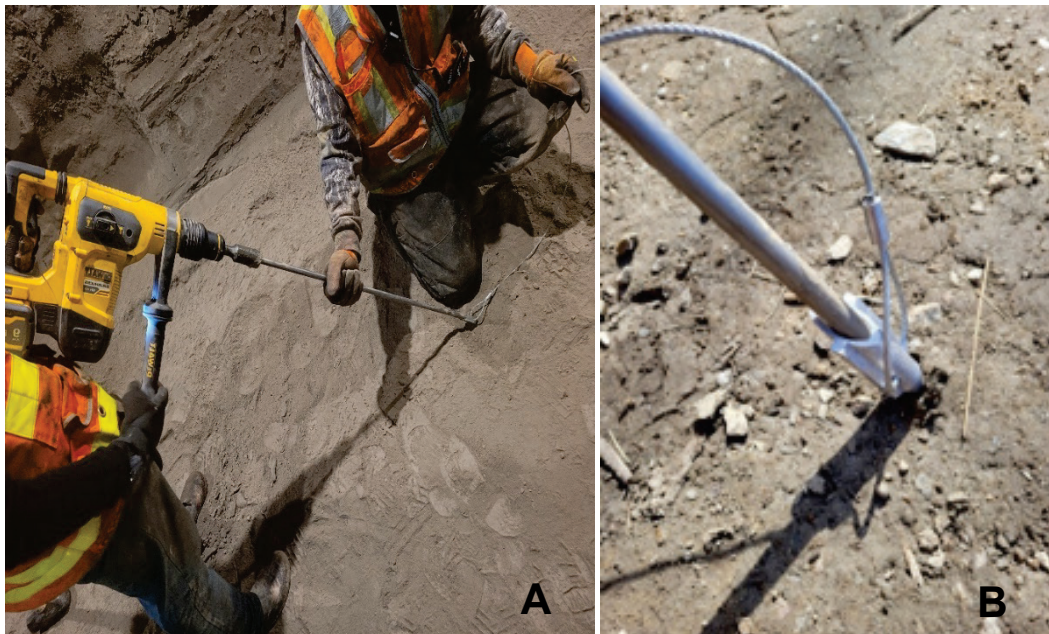
Figure 4-5. Bullet style anchor installation.
