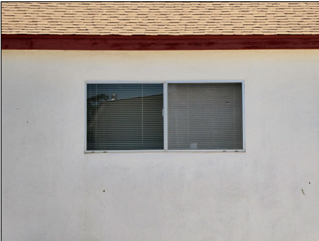
Figure 75. Close-up of replacement slider window, asphalt-shingled roof, and stucco panels used on the exterior of the building. (ERDC-CERL, 2021. Public domain.)
