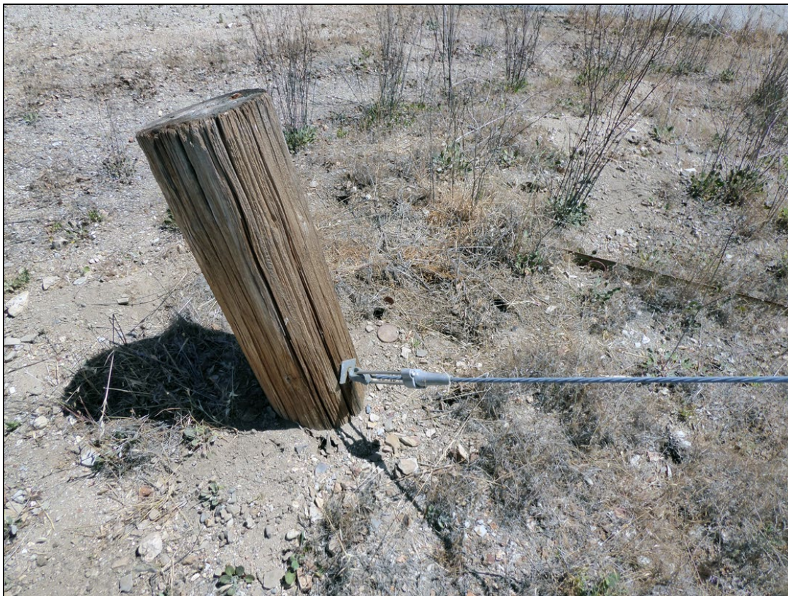
Figure 147. Buried post and guidewire supporting Structure 0301BS. (ERDC-CERL, 2021. Public domain.)
