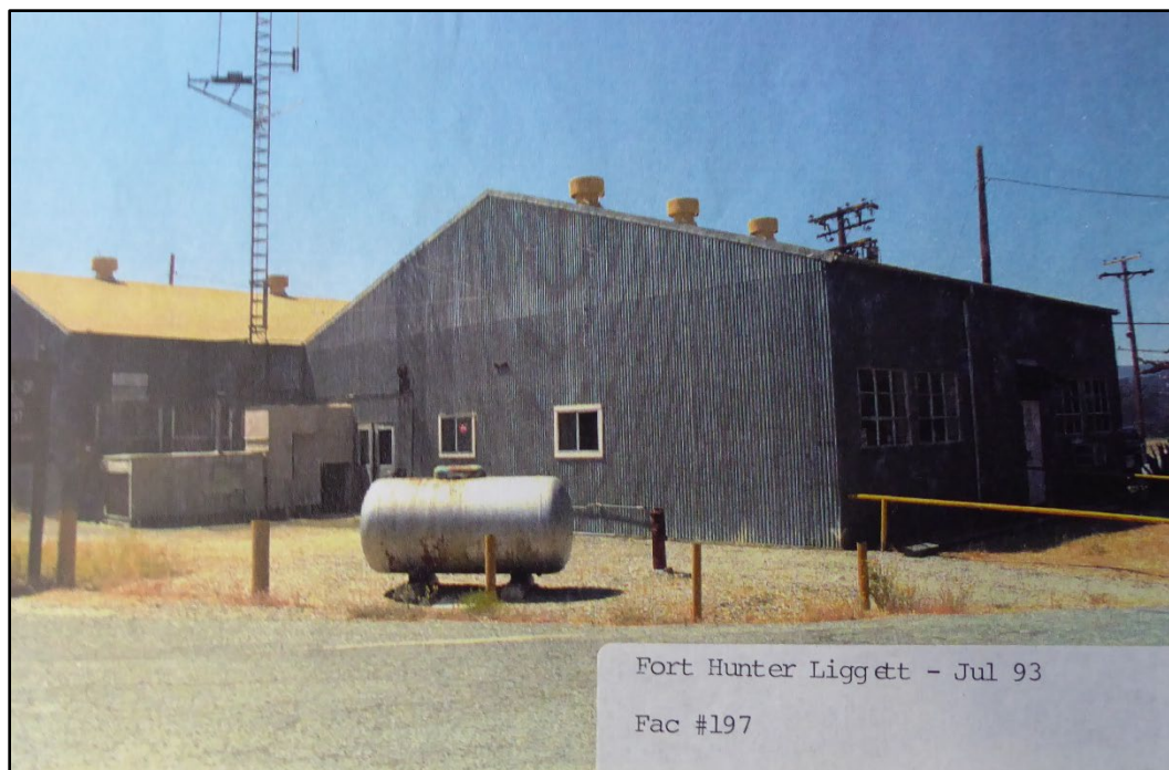
Figure 77. North oblique of Building 197 in 1993 showing the original corrugated metal clad exterior walls. (Fort Hunter Liggett Real Property Office. Public domain.)
