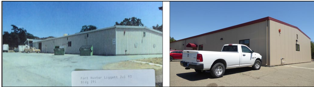
Figure 164. Comparison image of Building 291 in 1993 with the original metal siding to the current condition with addition of the Kingspan insulated panels (Fort Hunter Liggett Real Property Office and ERDC-CERL).
