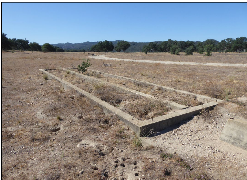
Figure 158. Board-formed concrete foundation remnants adjacent to the concrete circle. (ERDC-CERL, 2021. Public domain.)
