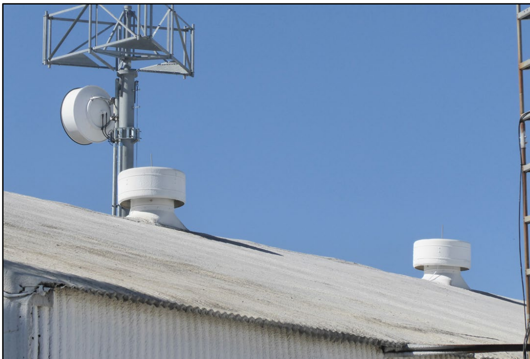
Figure 98. Close-up of the corrugated metal roofing covered with spray-on insulation foam on Building 197. (ERDC-CERL, 2021. Public domain.)
