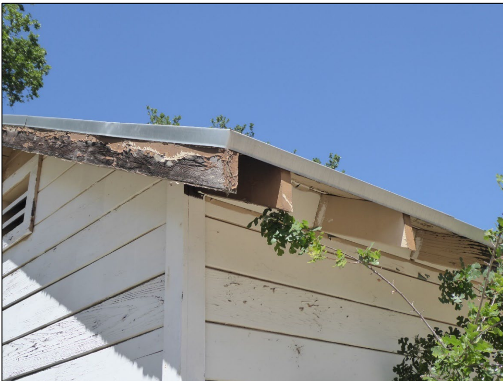
Figure 137. Detail of the southwest corner of Building 914 showing the corner board, rake board, and rafters. (ERDC-CERL, 2021. Public domain.)
