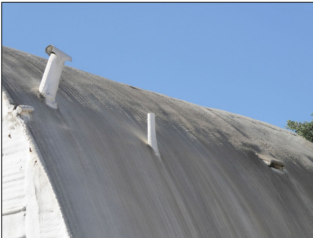
Figure 62. View of barrel roof of Building 179 with spray-foam insulation addition. (ERDC-CERL, 2021. Public domain.)
