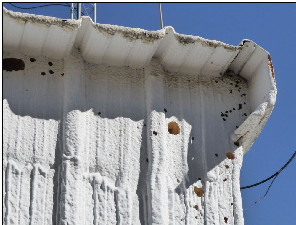
Figure 95. Close-up of the metal siding and metal roofing material covered with spray-on insulation on Building 197. (ERDC-CERL, 2021. Public domain.)
