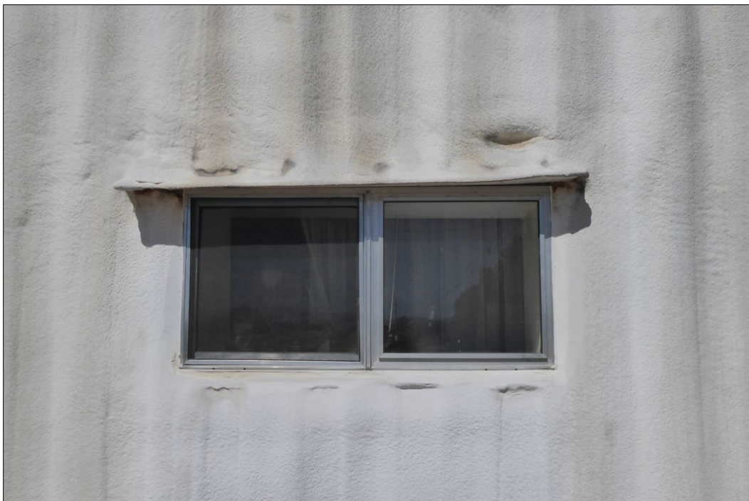
Figure 126. Close-up of a two-pane, bright aluminum slider window on Building 723. (ERDC-CERL, 2021. Public domain.)
