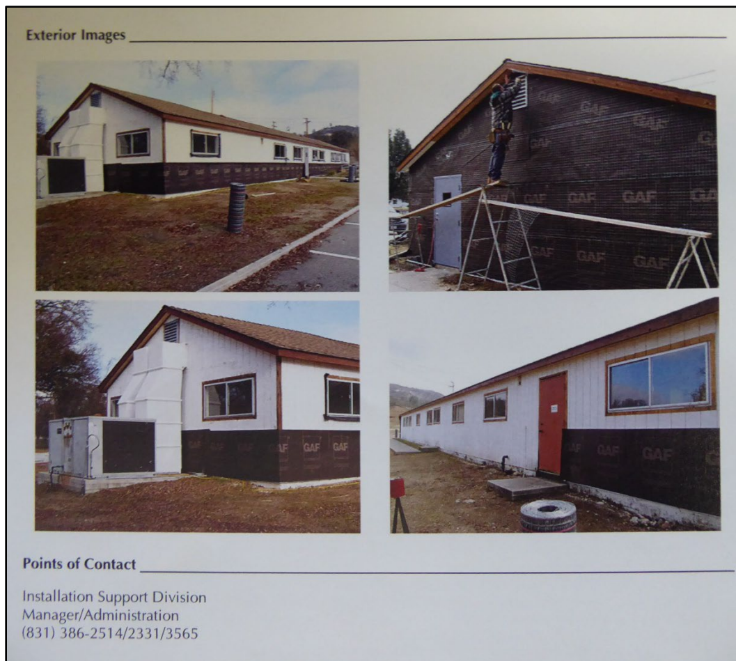
Figure 65. Documentation from the Real Property Master Plan for Fort Hunter Liggett showing the modifications to Building 196, including new windows, roof, and stucco panels covering existing exterior walls, 2006. (Fort Hunter Liggett Real Property Office. Public domain.)
