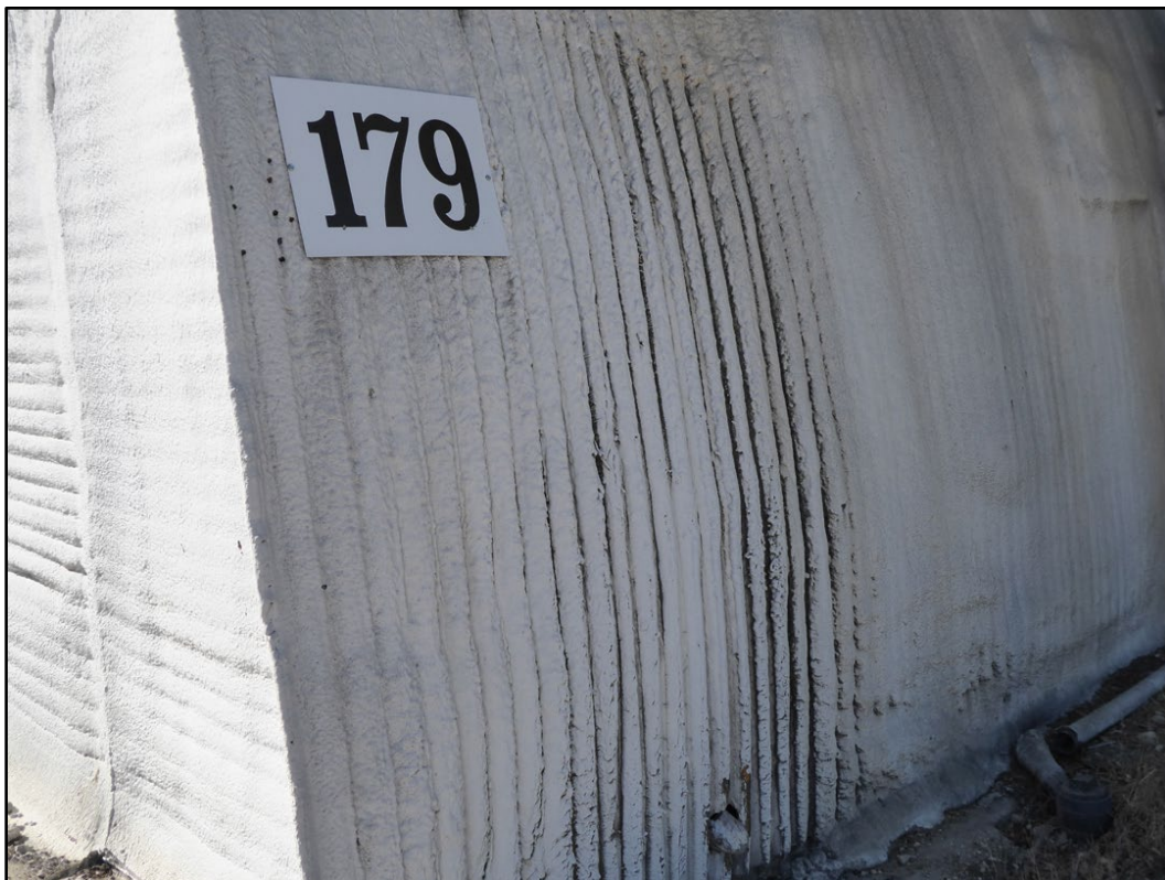
Figure 61. North corner of Building 179 and the close-up of the spray-foam insulation. (ERDC-CERL, 2021. Public domain.)
