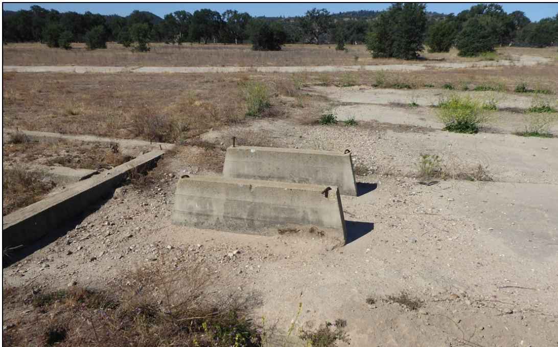
Figure 159. Close-up of the board-formed concrete foundations. (ERDC-CERL, 2021. Public domain.)
