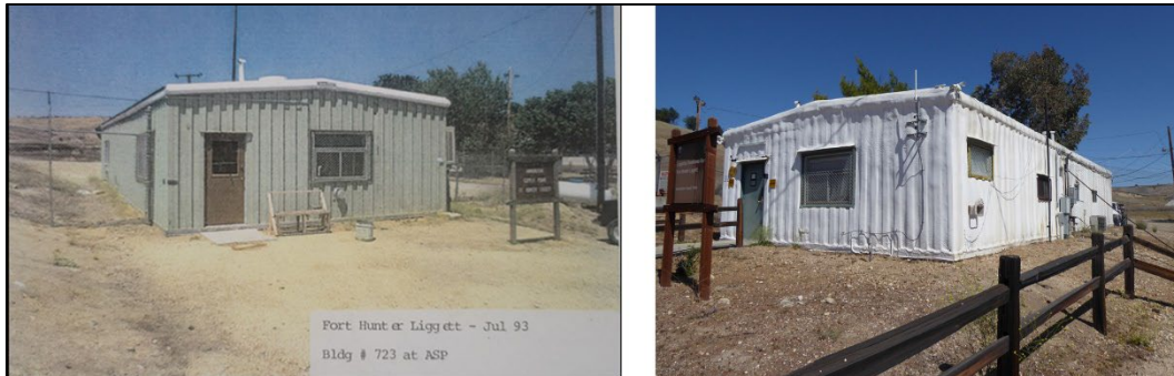
Figure 165. Comparison image of Building 723 in 1987 metal, prefabricated Butler building to the current condition with the addition of the spray-on insulation foam (Fort Hunter Liggett Real Property Office and ERDC-CERL).
