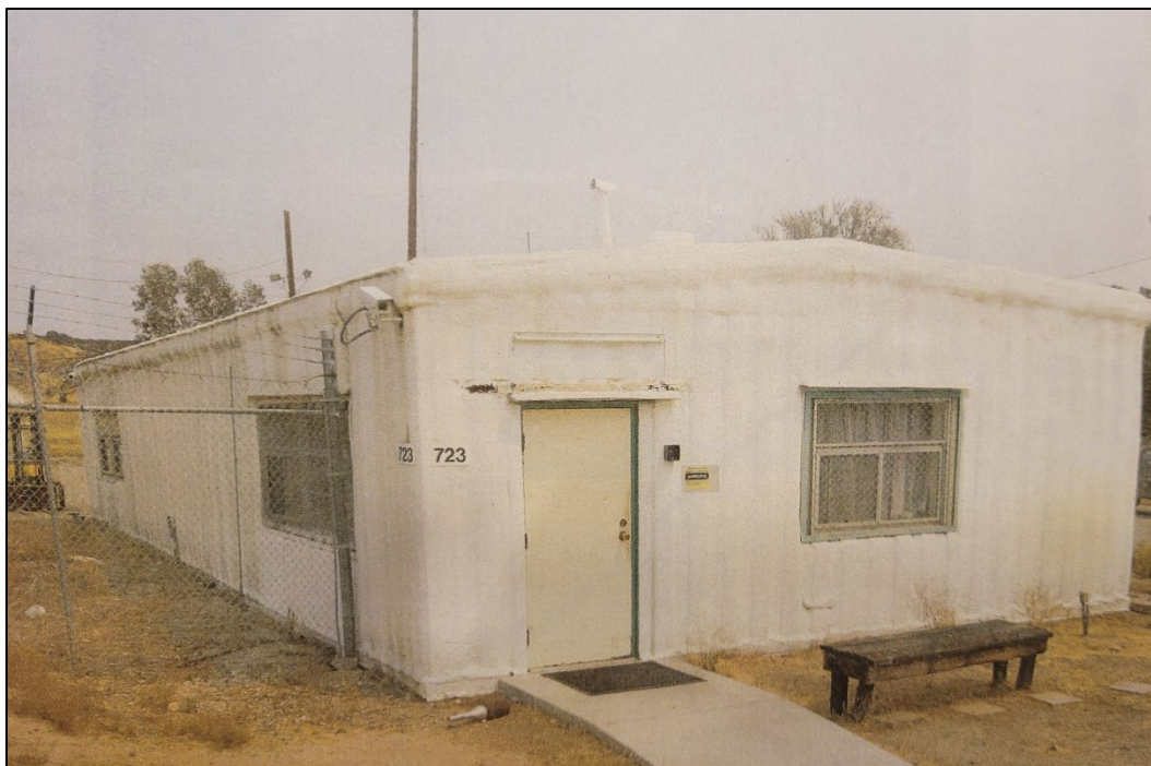
Figure 119. Building 723 exterior modifications with the addition of the spray-on insulation foam in 1999. (Fort Hunter Liggett Real Property Office. Public domain.)
