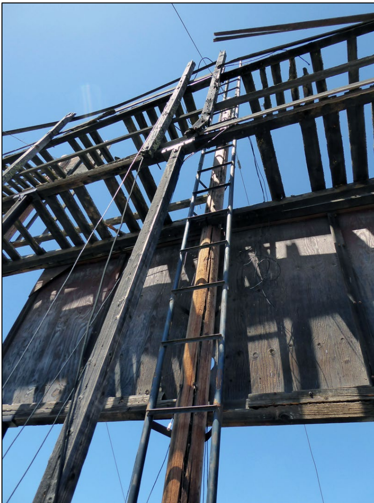
Figure 146. Looking up at the wooden column posts, access ladder, and remnants of the wooden platforms of Structure 0301BS. (ERDC-CERL, 2021. Public domain.)
