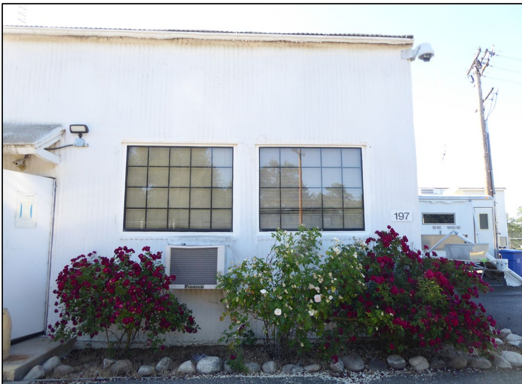
Figure 83. Replacement windows on the west elevation of Building 197. (ERDC-CERL, 2021. Public domain.)
