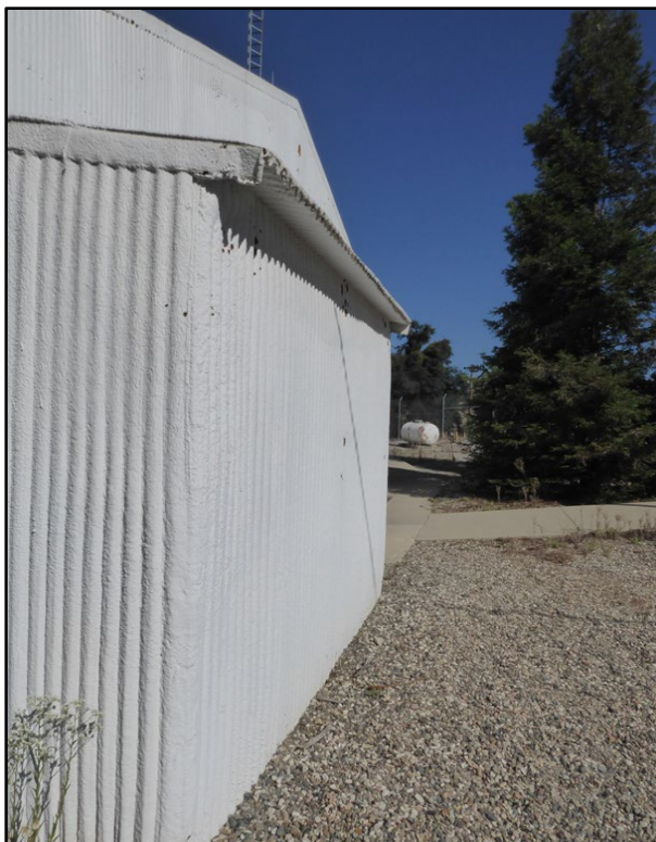
Figure 94. Close-up of the spray-on insulation foam used on Building 197. (ERDC-CERL, 2021. Public domain.)
