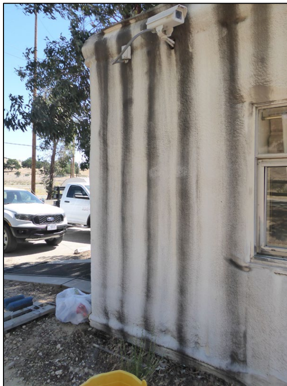
Figure 129. Close-up of the spray-on insulation foam that covers the original metal exterior siding on Building 723. (ERDC-CERL, 2021. Public domain.)
