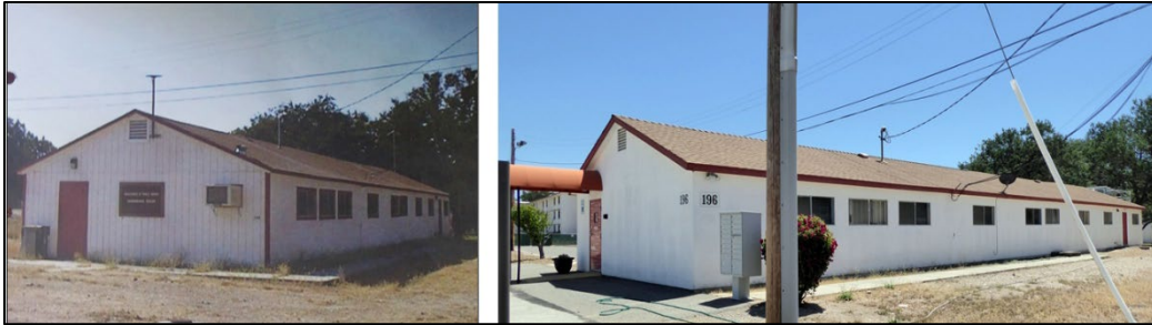
Figure 162. Comparison image of Building 196 with the original wood panel exterior walls (no date), to the current condition with the addition of the insulated panels used on the exterior of the building. (Real Property Office, Fort Hunter Liggett, California and ERDC-CERL.)
