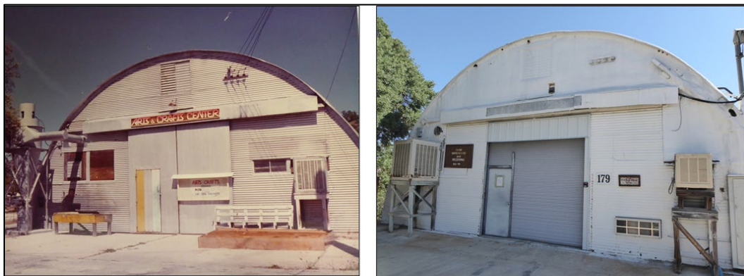
Figure 161. Comparison image of Building 179 in 1993 with original corrugated metal exterior to the condition in 2021 with the addition of the spray-on insulation foam. (Fort Hunter Liggett Real Property Office and ERDC-CERL.)
