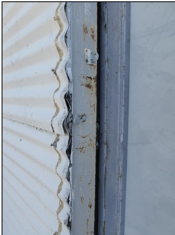
Figure 56. Close-up of the corrugated metal siding covered with spray-foam insulation on Building 179. (ERDC-CERL, 2021. Public domain.)
