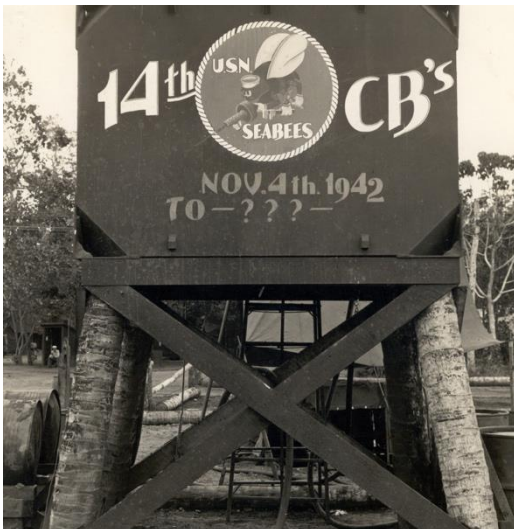
Elevated gas station built with a pontoon and palm tree trunks, WWII.
