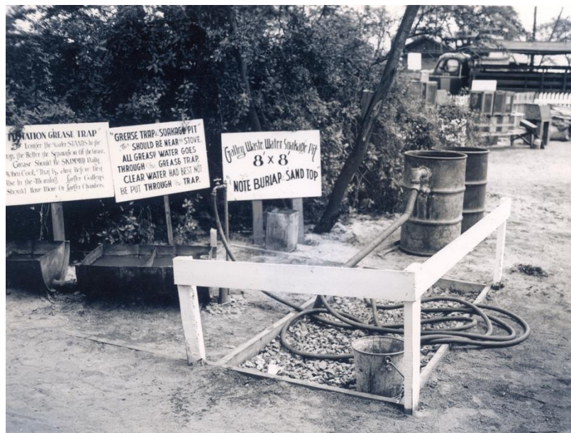
Galley waste water soakage pit and grease trap created by Seabees with the 81st NCB on Okinawa.
