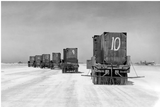
Water trucks made with pontoons rumble down airstrip at Eniwetok to aid in packing the coral on the strip, Marshall Islands.
