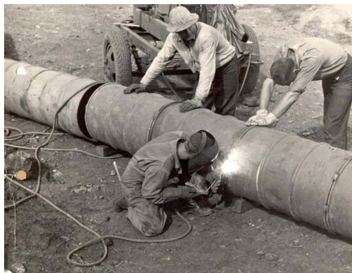
Seabees from the 75th Construction Battalion constructing a sewage pipeline from gasoline
