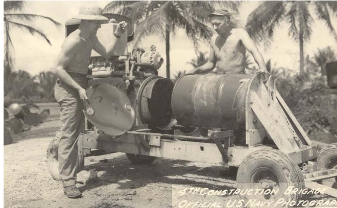
Seabees from the 71st Construction Battalion improvising a hydraulic barrel-end remover from a 55-gallon drum. The Seabees have a long history of creating need-based inventions with the 55-gallon drum.
