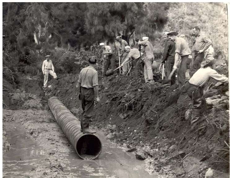
Seabees from the 75th Construction Battalion laying a sewage pipeline made entirely from 55-gallon drums. The Seabees have a long history of creating need-based inventions with the 55-gallon drum.
