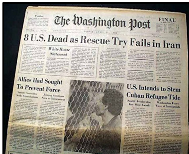
Figure 106. Newspaper Depicting the Failure of Operation EAGLE CLAW 925
