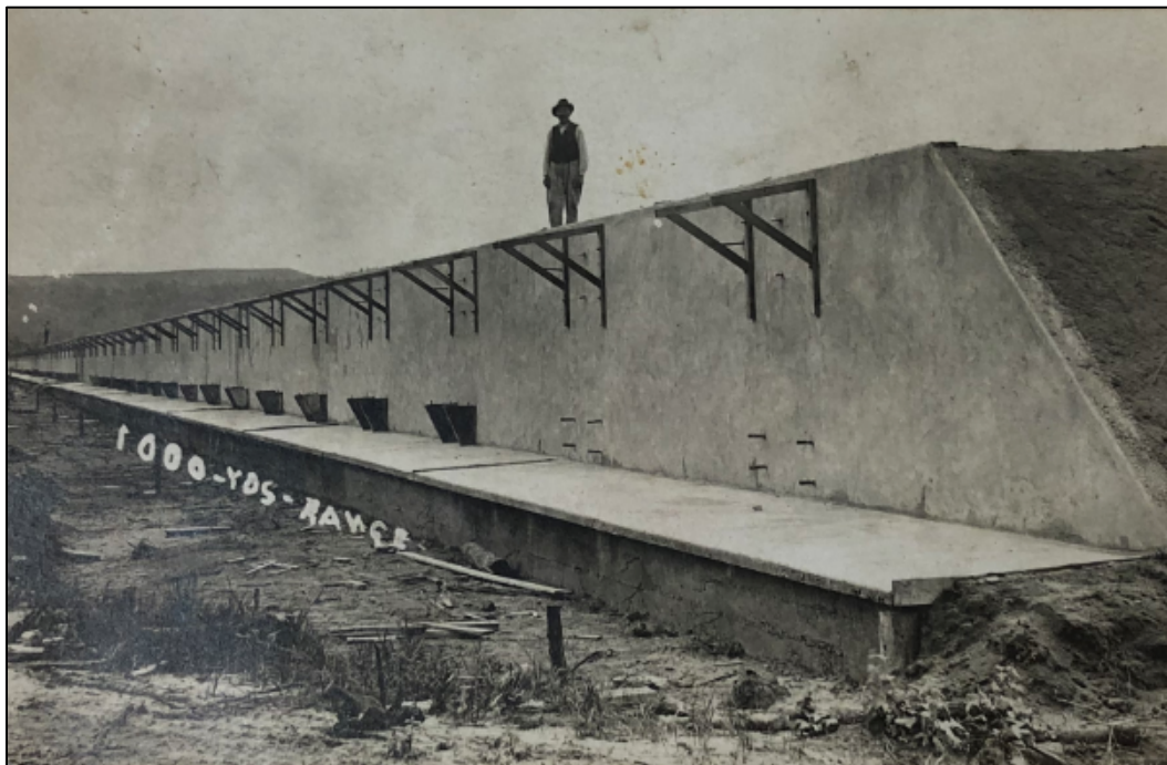
Figure 16. Concrete target butt of 1,000-yard range, n.d. (Image from Fort McCoy Historical Center. Public Domain).
