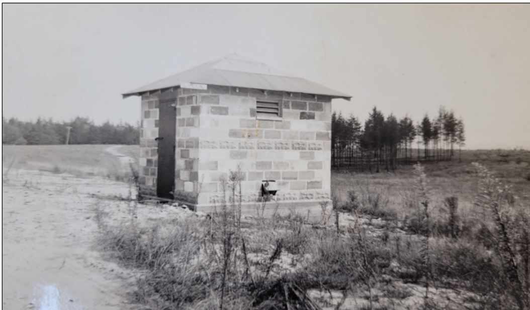
Figure 39. 10 ft by 10 ft ordnance magazine completed on 1 August 1940, n.d. (Image from Fort McCoy Historical Center. Public Domain).
