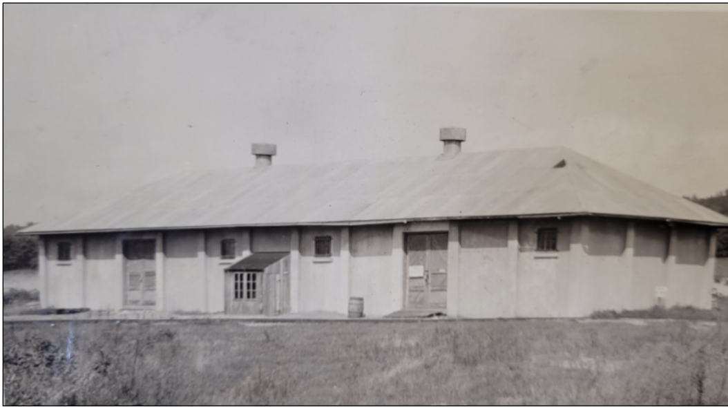
Figure 9. Concrete ordnance magazine constructed in 1909, 1940 (Image from Fort McCoy Historical Center. Public Domain).
