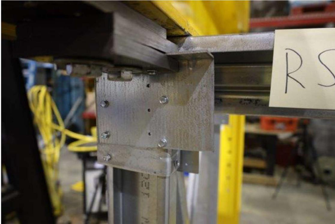
Figure 20: Typical End Bearing Connection
