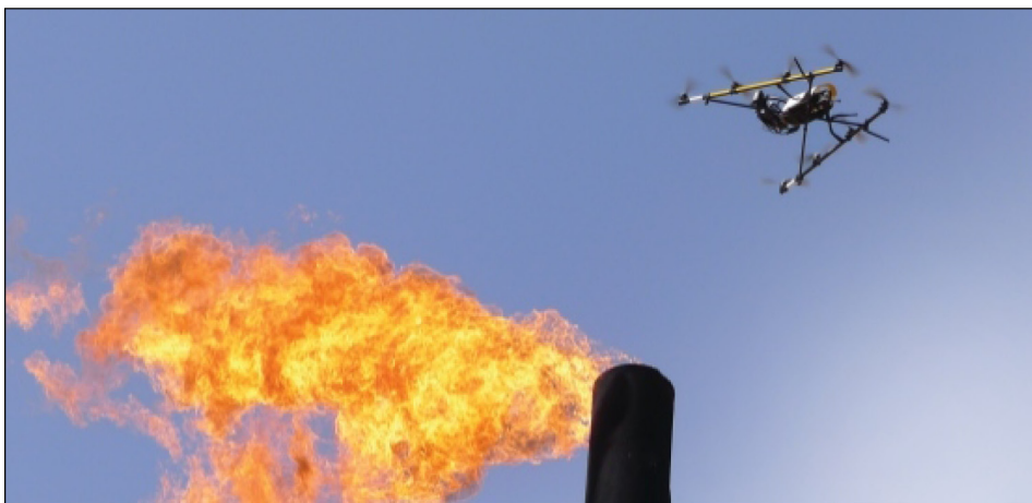
Flare stack inspection
