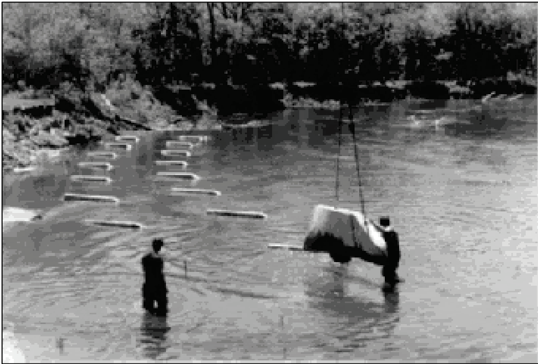
Figure 9. Installation of concrete Iowa vanes at low flow.
