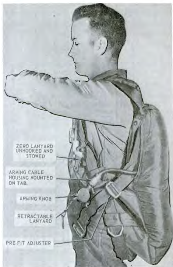
Figure 16-5. Arrangement of Arming Accessories, Automatic Back Parachute.
