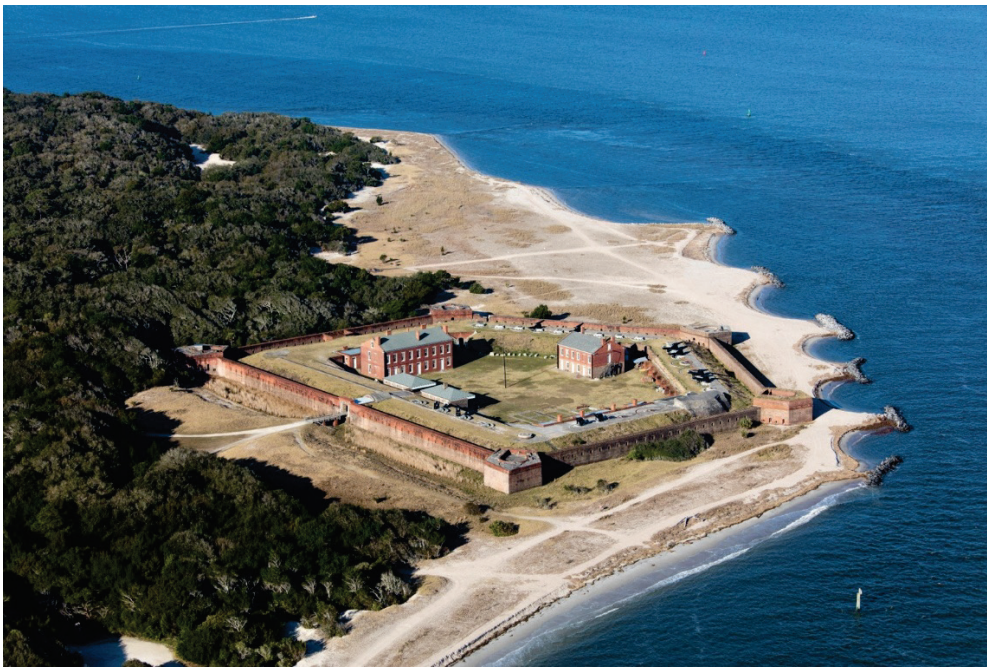
Figure 2-7. A series of T-Shaped groins, man-made structures designed to trap sand as it is moved down the beach by longshore drift. Photo Credit: USACE: Jacksonville District.
