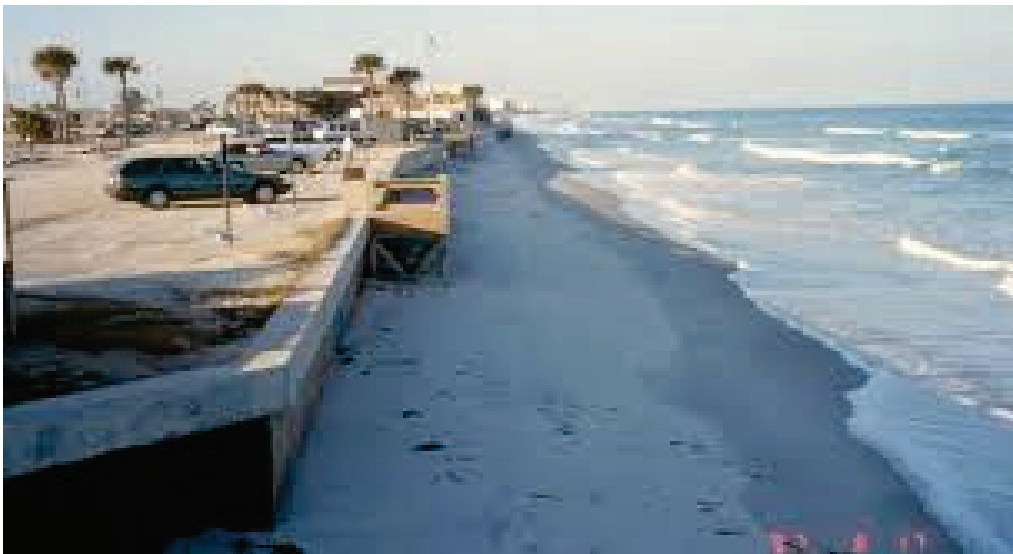
Figure 2-6. An example of a hard structure (e.g., seawall) used to protect property from erosion. Photo Credit: USACE: Jacksonville District.
