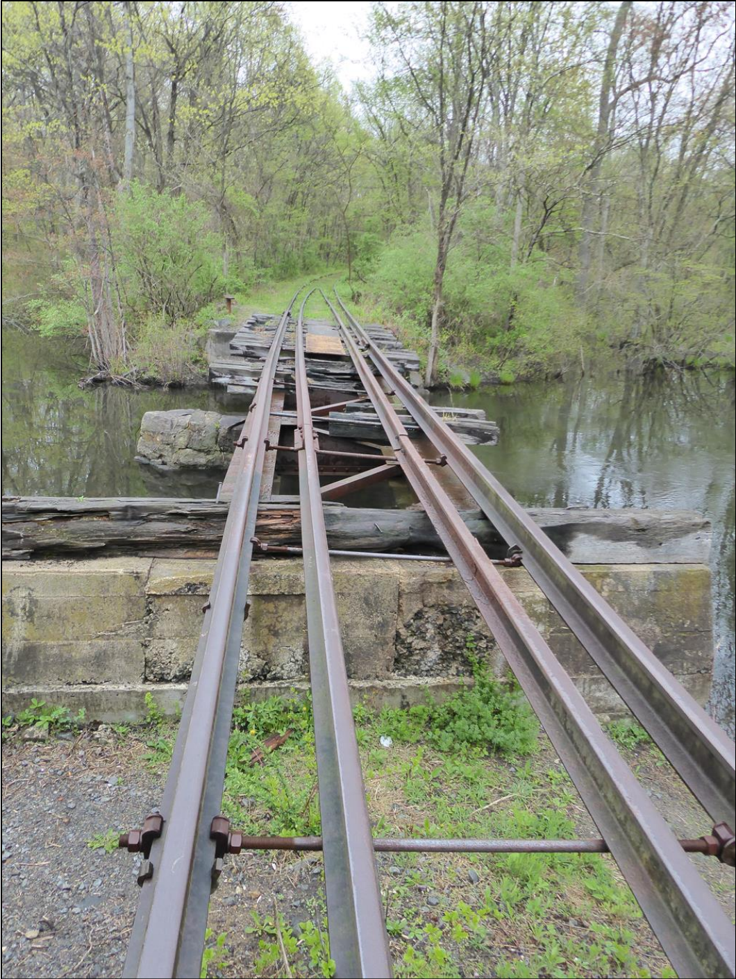
Figure 50. Looking east across the Rockaway River bridge.
