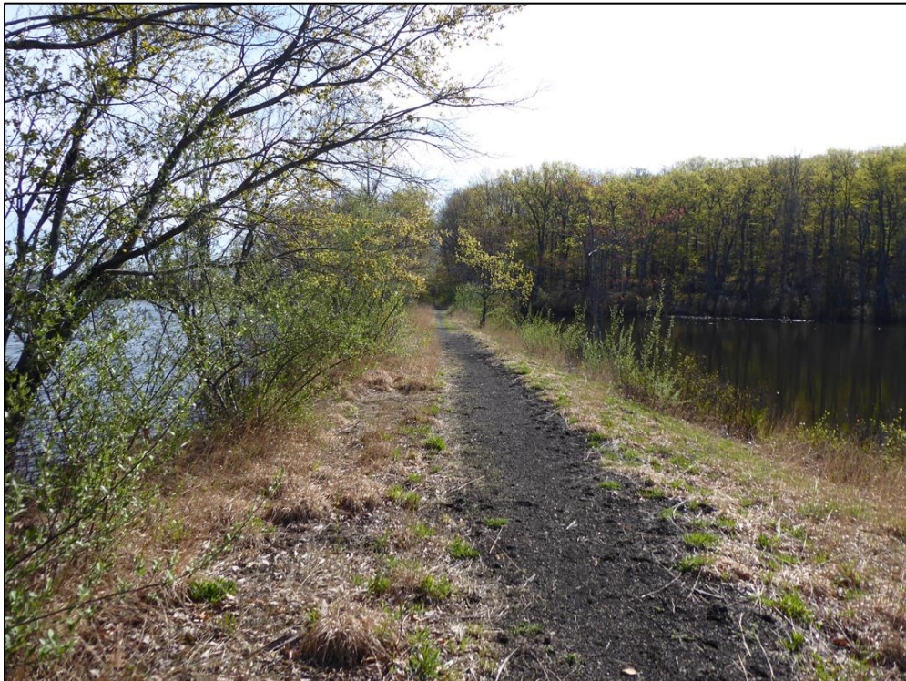
Figure 88. Looking north along the ROW at Lake Denmark.
