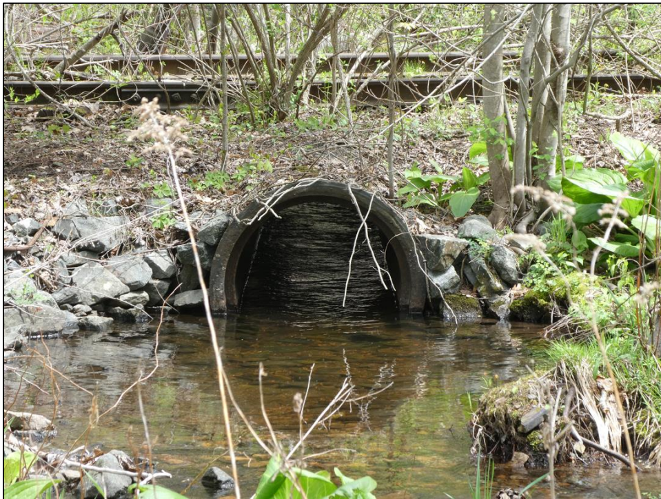
Figure 63. Looking at a concrete pipe culvert under the tracks.
