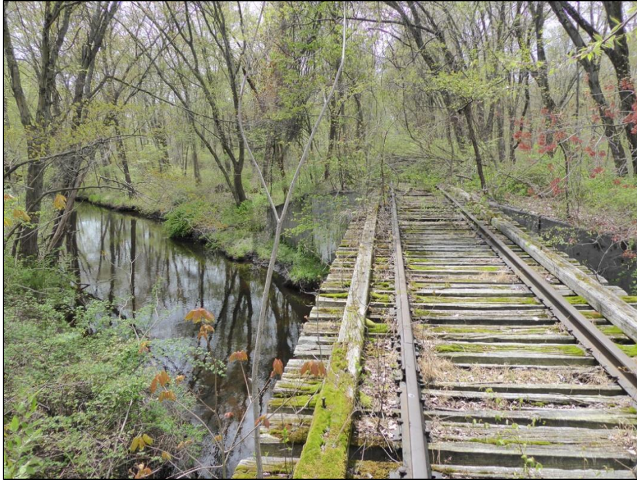
Figure 58. Looking west at a bridge over Green Pond Brook.
