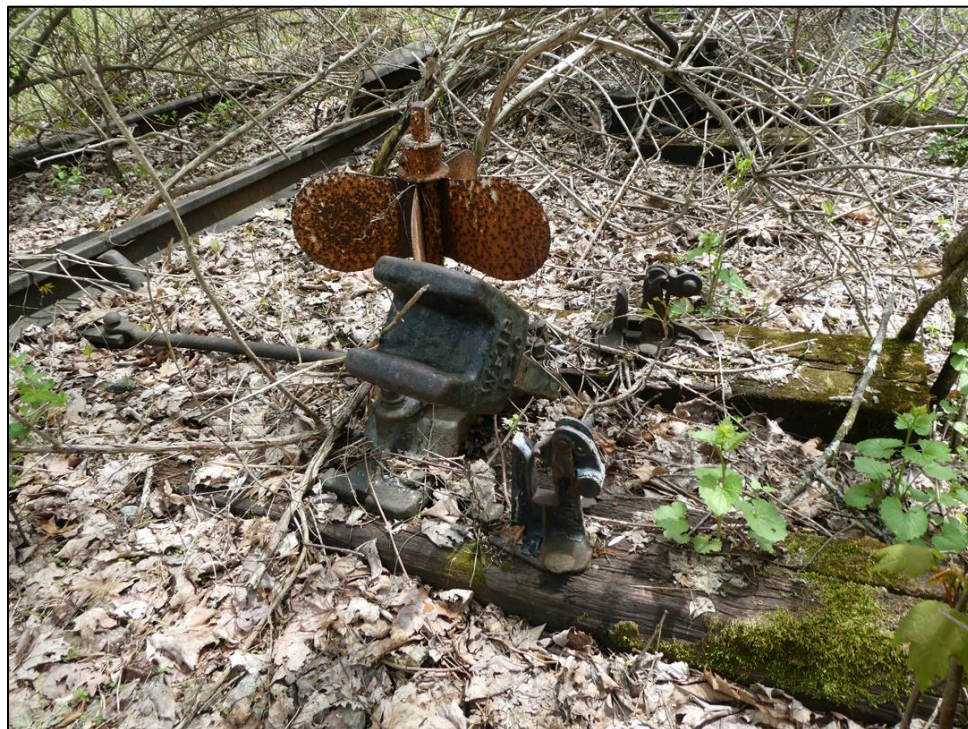
Figure 65. Detail of a switch.
