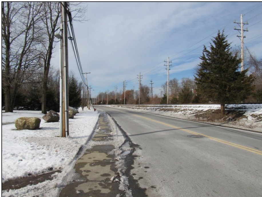
Figure 101. Looking west along West Dewey Avenue at the former location of Wharton branch viaduct.
