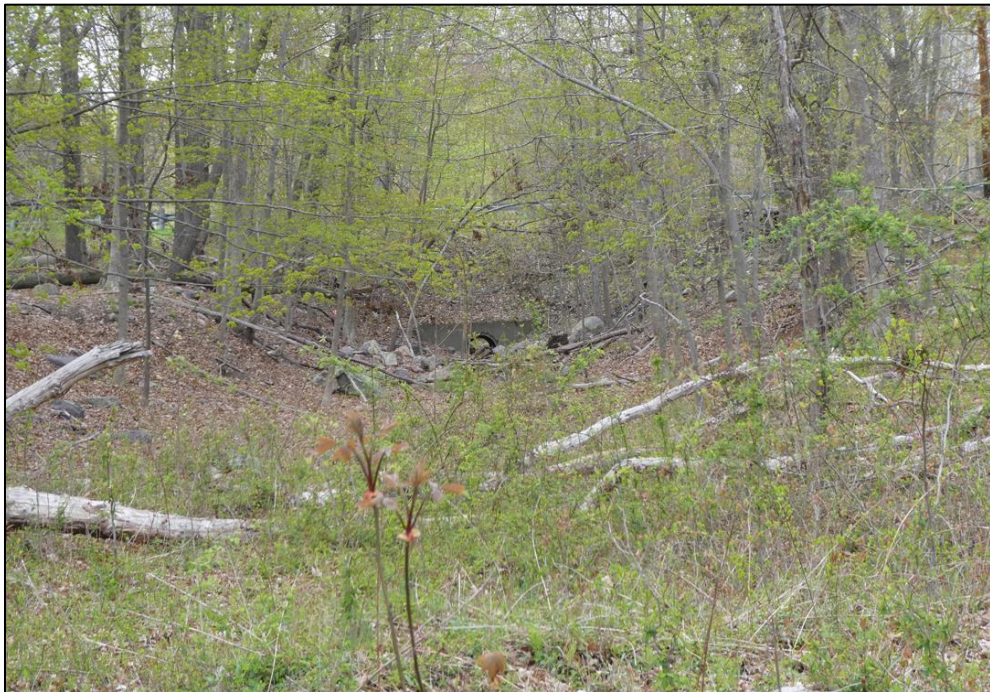
Figure 96. Looking north to culvert under Green Pond Road (location of original Hump Back Bridge on ROW).
