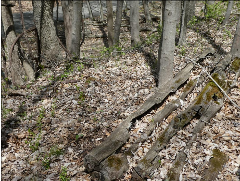
Figure 82. Decaying railroad tie along the ROW by the former Lake Denmark boundary.
