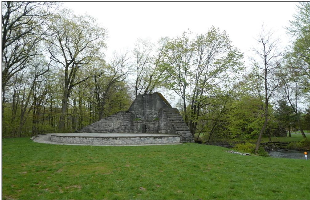
Figure 102. Looking east at the stone support for the former Wharton branch of the Wharton & Northern bridge over the Rockaway River.
