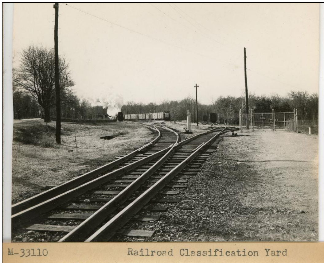
Figure 28. Looking southwest from Cannon Gate with the Wharton & Northern ROW on the left and the Army-owned classification yard on the right.
