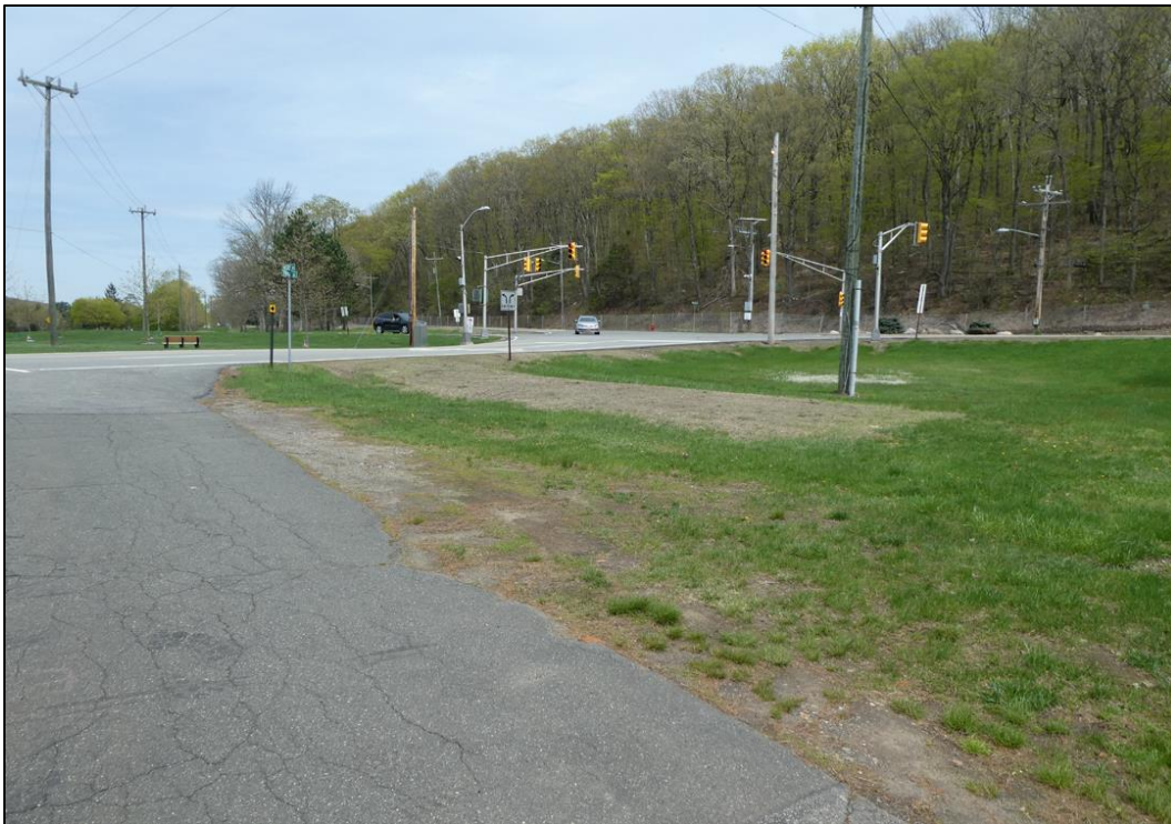
Figure 68. Looking north along ROW towards First Street.
