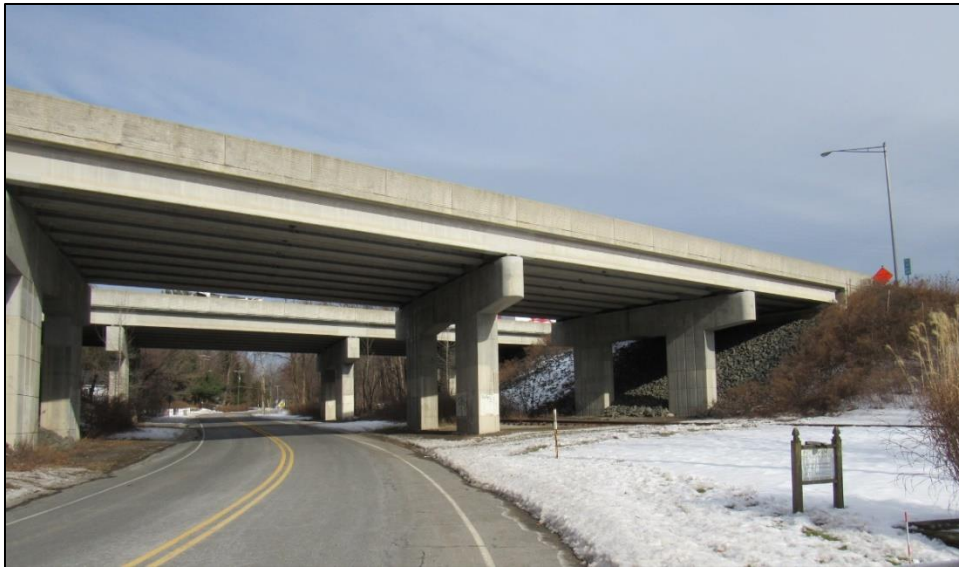
Figure 46. Looking north along Berkshire Valley Road at I-80 showing the separate area for the Wharton & Northern ROW on the east.
