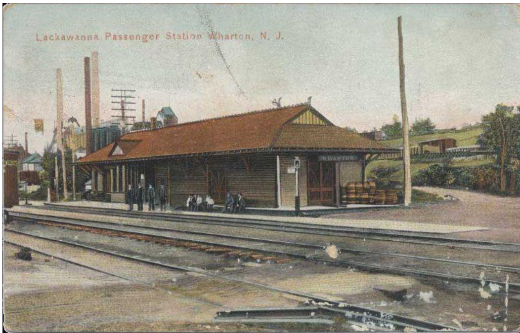
Figure 18. Wharton depot on the Lackawanna railroad (note Wharton Iron Furnace in background), no date.
