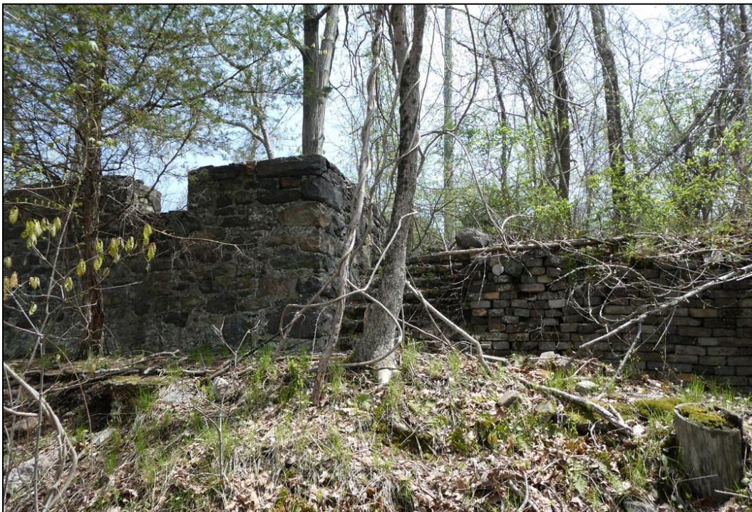
Figure 77. Looking up at the steps to the Factory Railroad Station (Site number: 28-Mr-345).
