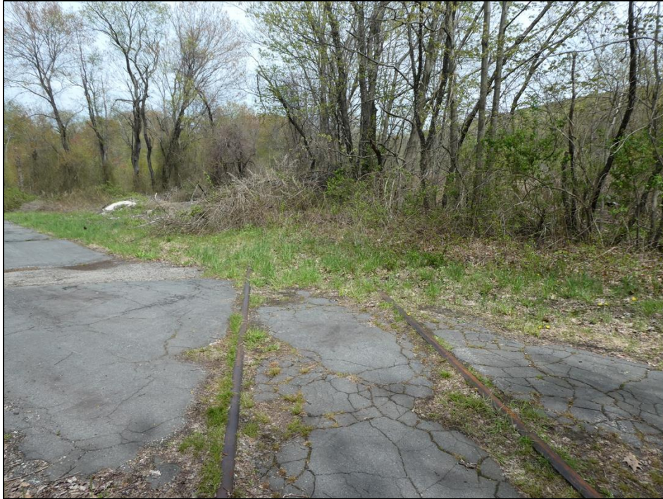
Figure 60. Looking east at ROW past Brook Road.
