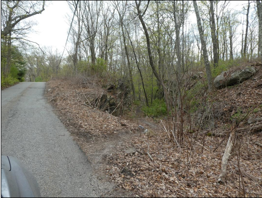
Figure 99. Looking north at Oreland Branch ROW as it crosses Upper Hibernia Road.
