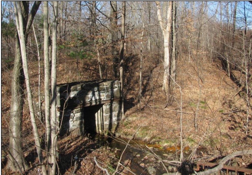
Figure 74. Looking south at a stone culvert adjacent to Bott Road.
