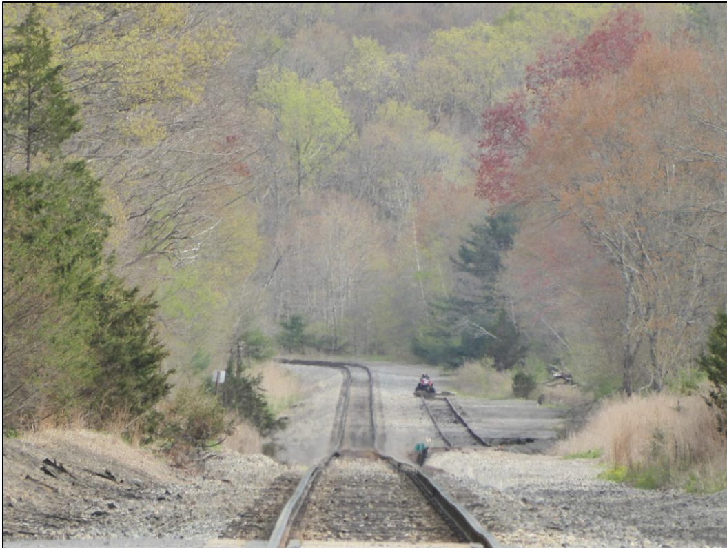
Figure 97. Looking east along the Susquehanna Railroad at the former Charlotteburg Junction to the Wharton & Northern.
