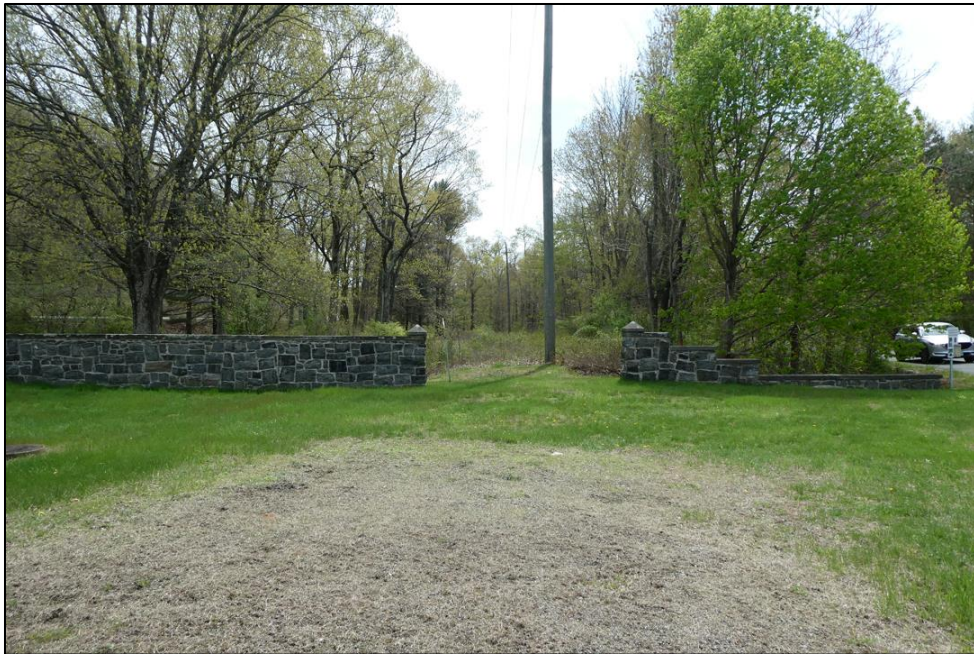
Figure 66. Looking south at the stone wall abutting the Picatinny Arsenal Cannon Gate for the ROW of the Wharton & Northern.
