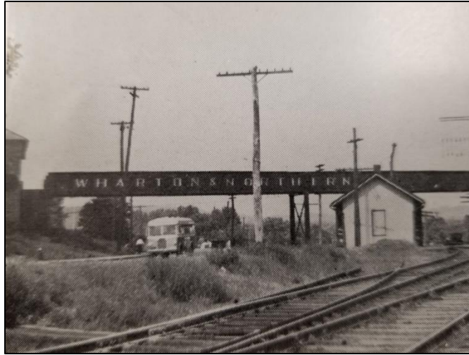
Figure 13. Trestle over the Lackawanna and Dewey Avenue, no date.
