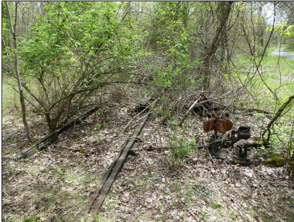
Figure 64. Looking south along the ROW east of Moody Road.
