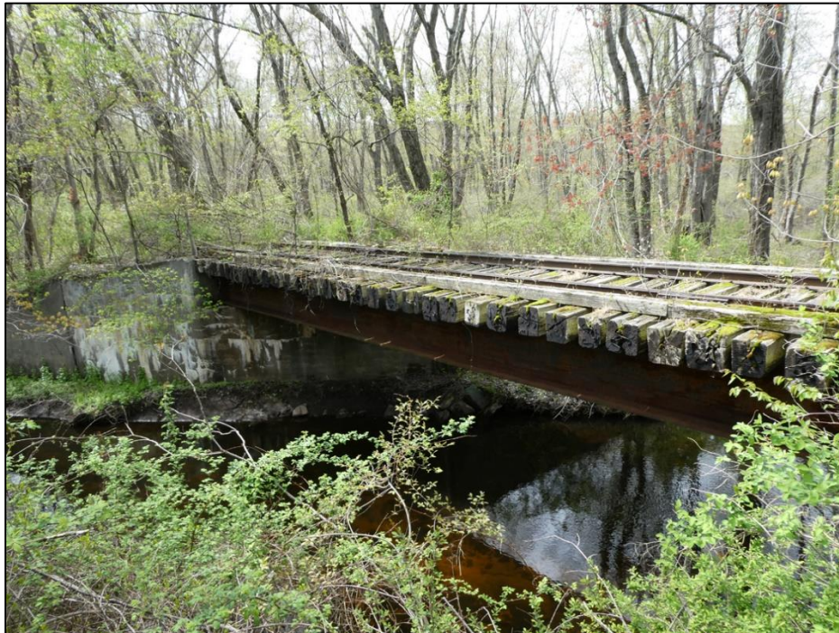
Figure 59. Bridge over Green Pond Creek.
