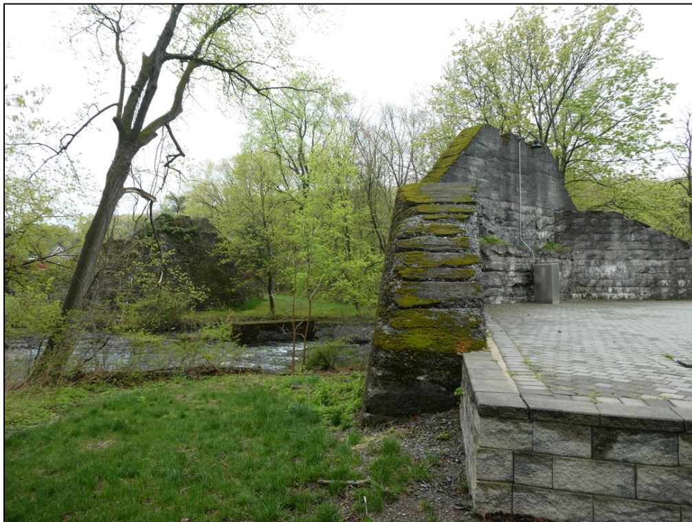
Figure 103. Looking south at the two stone supports for the former Wharton branch of the Wharton & Northern bridge over the Rockaway River.
