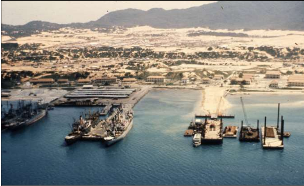
Figure 1. DeLong Piers in Vietnam. This photograph is oriented toward the east and shows DeLong pier number one on the left and DeLong pier number three being constructed on the right at Cam Ranh Bay. USACE LNO trip slides Vietnam 5.182 . Photograph by United States Army Corps of Engineers, November 7, 1966. Vietnam Trip Briefings by OCE Liaison Officer, Office of History, Headquarters, US Army Corps of Engineers, Alexandria, VA.
