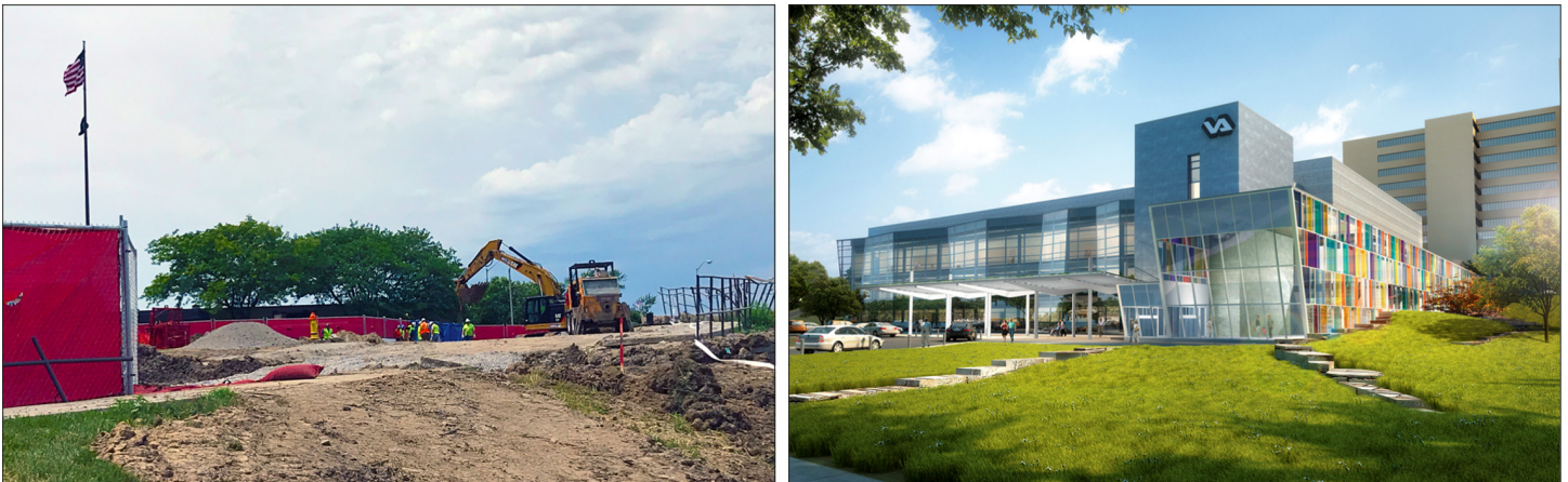
Figure 1: Department of Veterans Affairs’ Ambulatory Care Center in Omaha, NE—Construction Site and Rendering of Completed Facility
