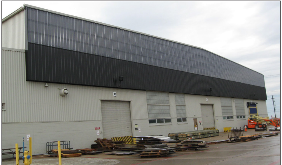
Figure 5: Solar Wall at Letterkenny Army Depot
