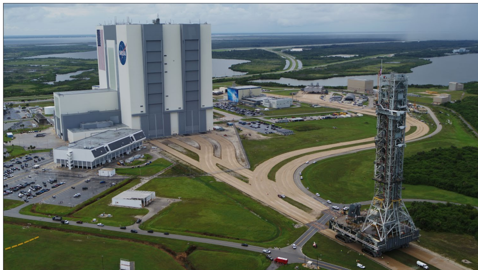
Figure 2: Mobile Launcher on the Crawler-Transporter outside the Vehicle Assembly Building at Kennedy Space Center
