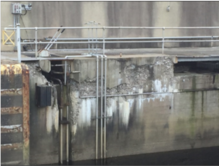
Crumbling concrete wall of lock chamber at Allegheny River Lock and Dam 2 in Pittsburgh, Pennsylvania, (left) and recently rehabilitated lock chamber wall at Emsworth Locks and Dams in Pittsburgh, Pennsylvania (right). Crumbling concrete walls may present safety risks associated with falling and unstable walls.
