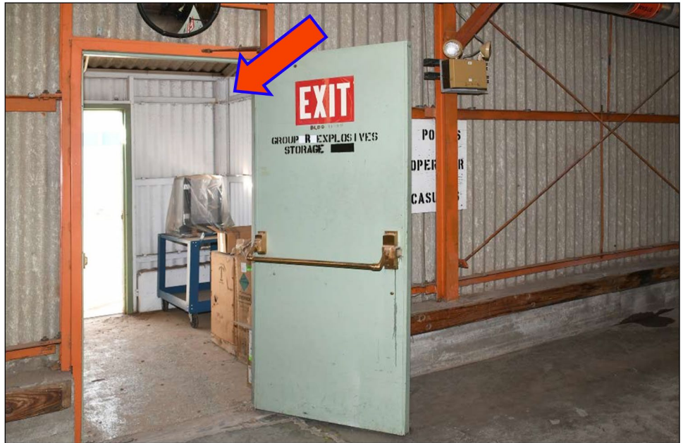
Figure 6: Inert (Non-explosives) Storage Closet at Pantex Plant that Is Characterized as an Explosives-Related Asset
