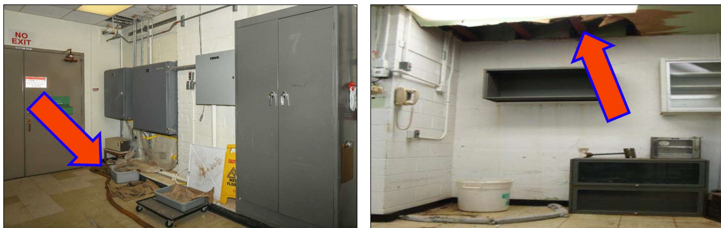
Figure 4: Weather Damage in the Analytics and Chemistry Laboratory at the Pantex Plant
