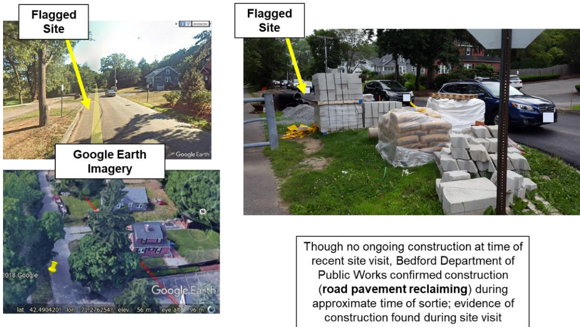
Figure 29. Road construction detected by algorithm.
