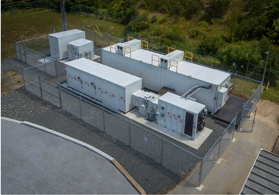
Figure 6. 800kW UltraBattery® ESS at Aqua (King of Prussia, PA)
