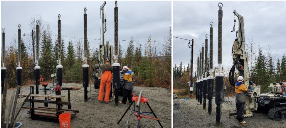
Figure 10. Installation of thermistor string casings (R1-R3) with a Geoprobe 7822.
