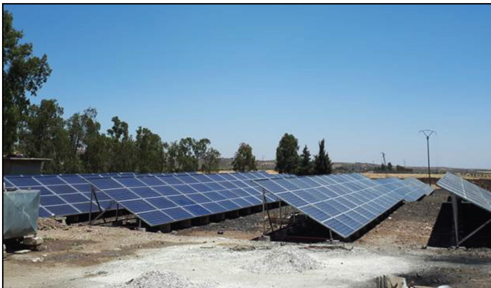
Figure 5: USAID-Supported Solar Array Installation Providing Renewable Energy for a Drinking Water Pumping Station in Dar'a Province, Syria
