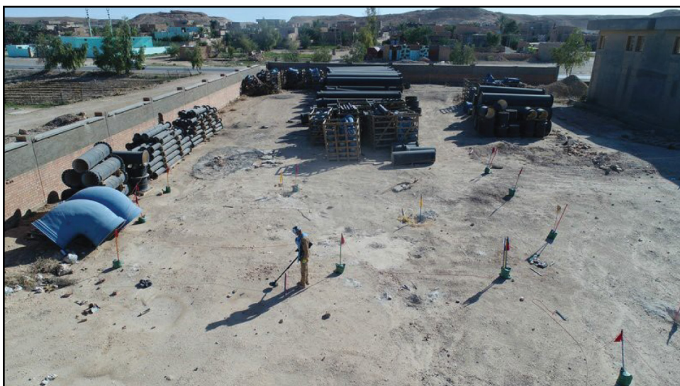
Figure 4: State-Supported Explosive Remnants of War Clearance Operations at a Water Treatment Facility in Iraq
