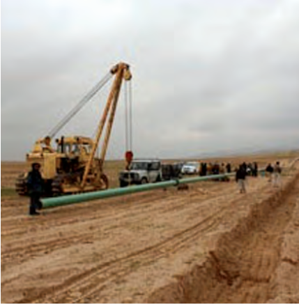
The Mazar-Sheberghahn pipeline was rehabilitated with the assistance of TFBSO. (GIROA photo)
