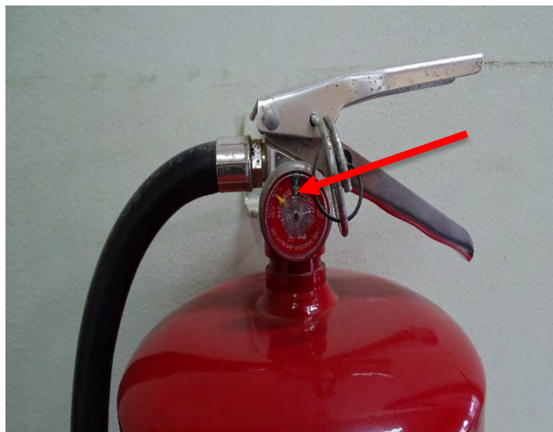
Photo 7 - Empty Fire Extinguisher
