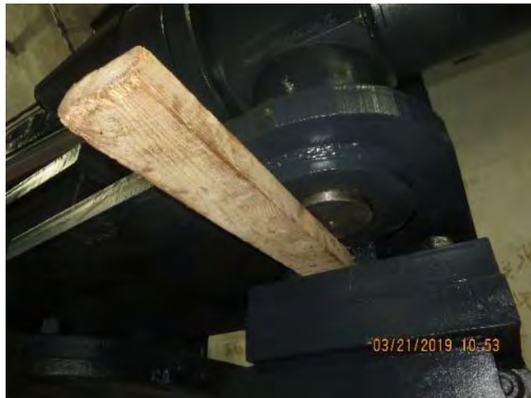
Photo 2 - Lumber Supporting the Emergency Closure Valve Pins
