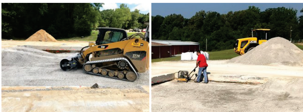
Figure 12. Compaction of crushed limestone base with the roller attachment (left) and plate compactor (right).
