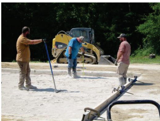
(e) Spot checking flowable fill depth
