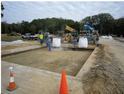
(a) Mobilizing super sacks of flowable fill
