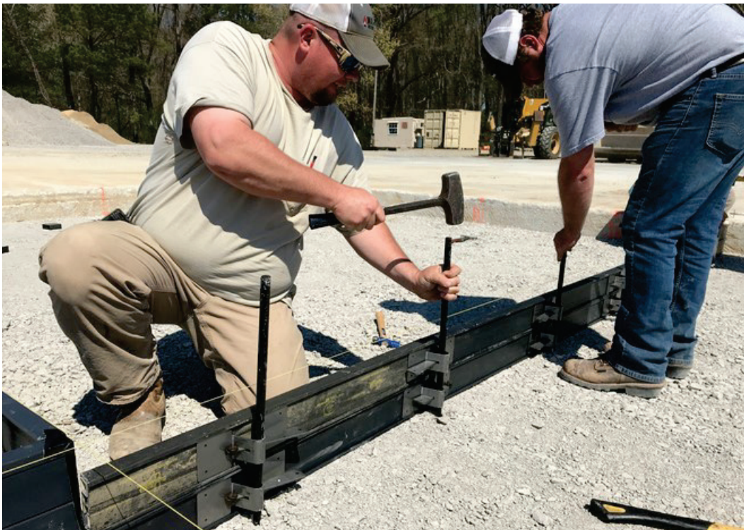
Figure 19. Staking forms.
