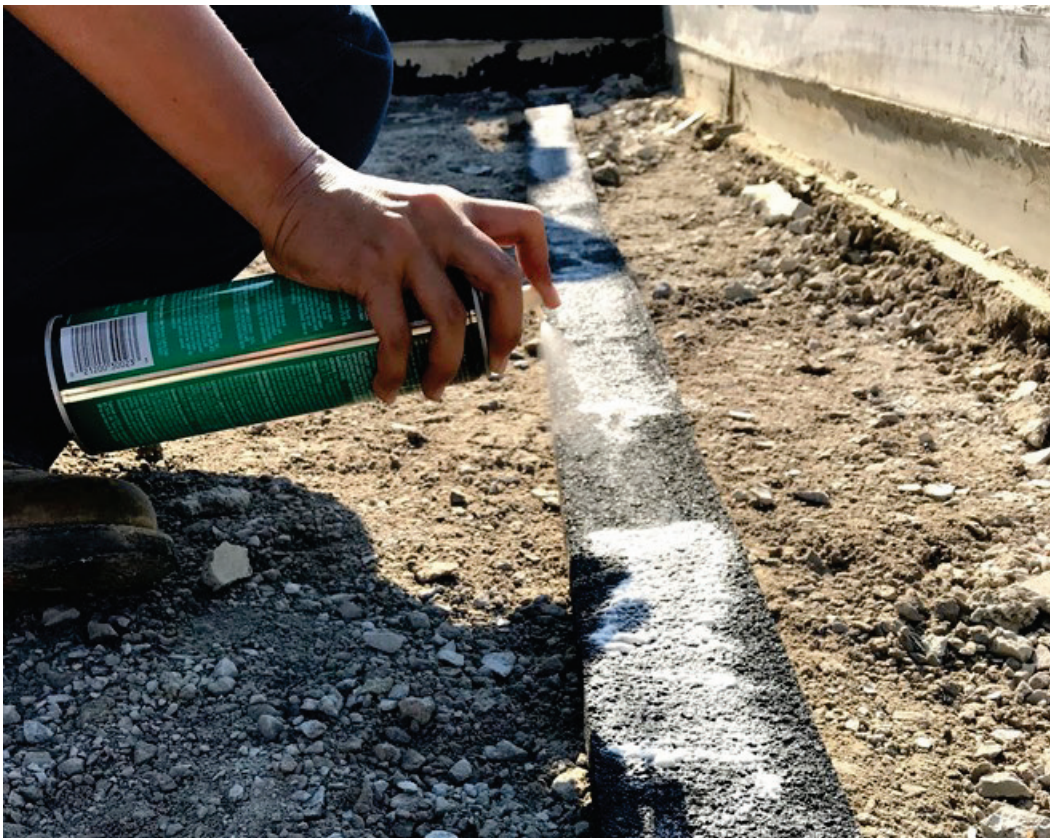
Figure 24. Spray adhesive on expansion board.
