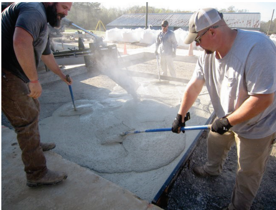
Figure 26. Close-up of placing rapid-setting concrete.
