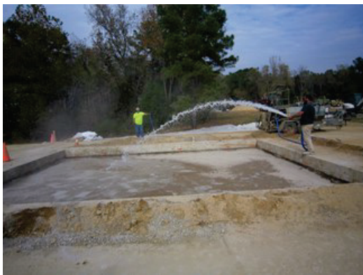
(c) Adding water to dry flowable fill
