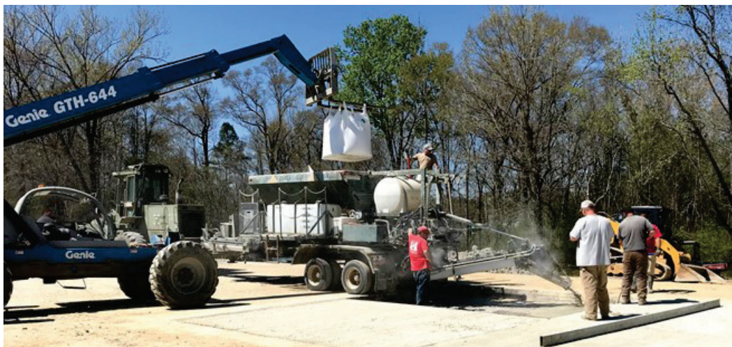
Figure 26. Close-up of placing rapid-setting concrete.
