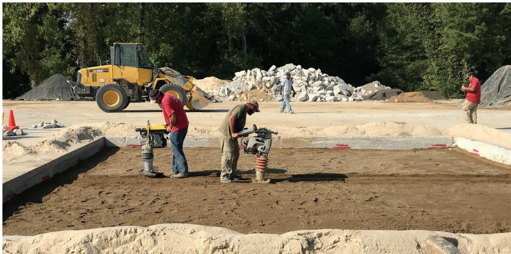
Figure 18. Jumping jack compaction.
