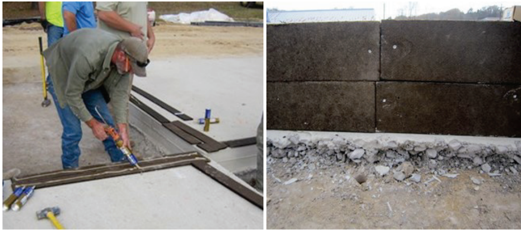
Figure 21. Installation of expansion board that included a combination of applying Liquid Nails and masonry nails in the curing rapid-setting concrete (Repair 1).
