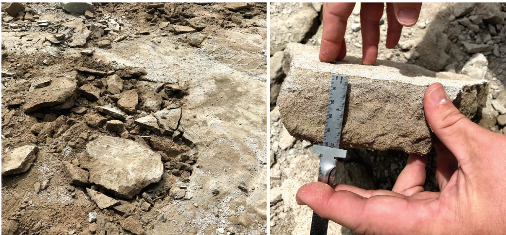
Figure 45. Close-up of flowable fill layers during removal.
