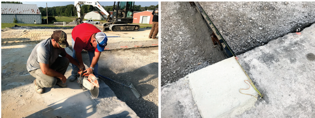
Figure 34. Patching high-severity joint spalls on the parent slabs adjacent to the repair area.
