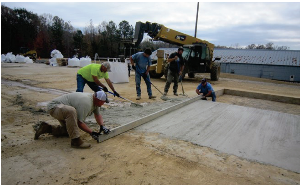
Figure 28. Screeding with 20-ft-long magnesium bar.
