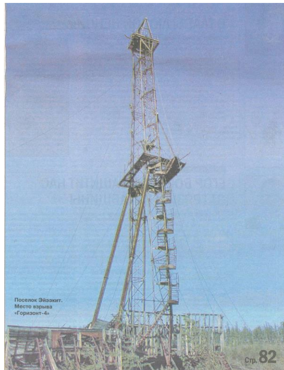
Figure 95. The emplacement tower for the Horizon-4 PNE.
