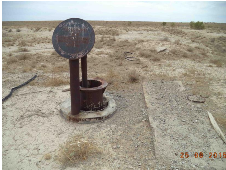
Figure 69. Borehole of Meridian-3.
