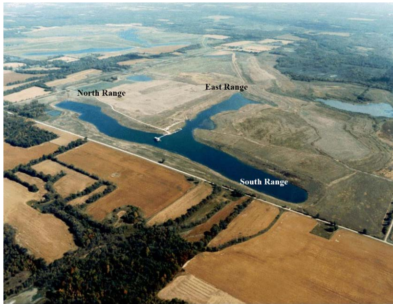
Figure 2. Lake Glendora Test Facility
