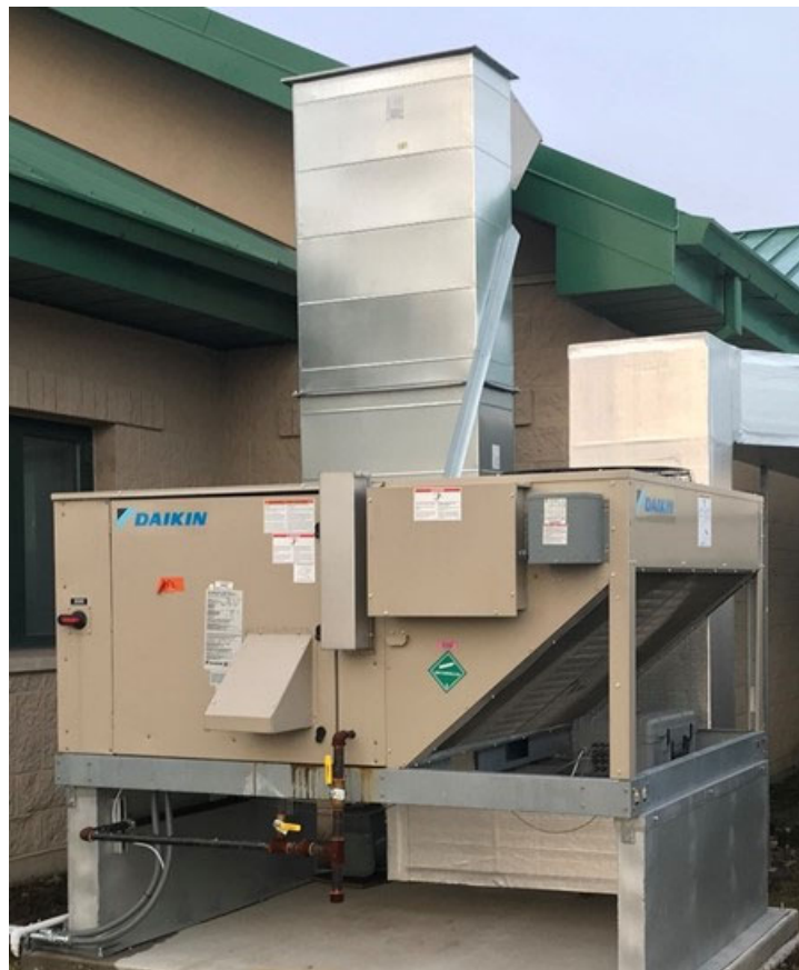
Figure 5 A DOAS conditioned ventilation air (100%OA) for the demonstration site
