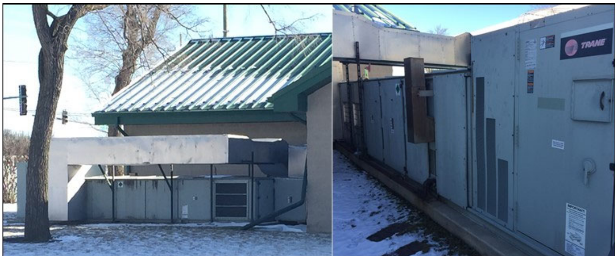
Figure 2 Example of a ground-mounted VAV system
