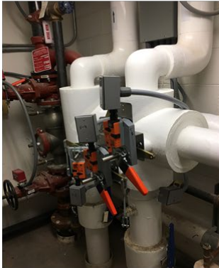
Installation of bypass valves
