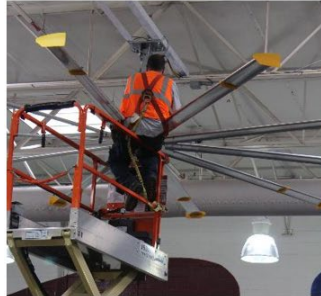
Installing 18' dia. DC ceiling fans
