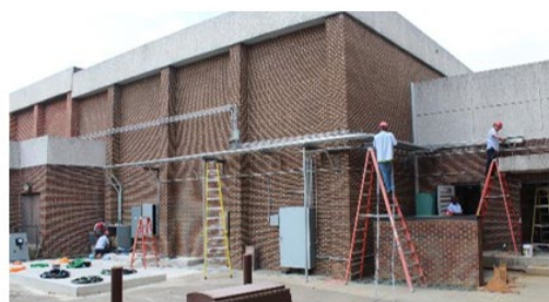
Installing outdoor conduit
