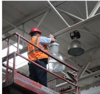
Replacing AC HID Lights
