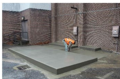
Finished slabs for outdoor equipment
