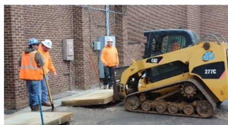
Removal of unused concrete slabs
