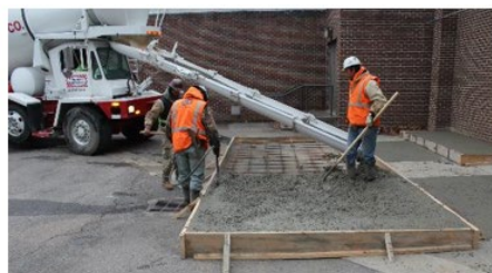
Pouring new slab for battery storage container
