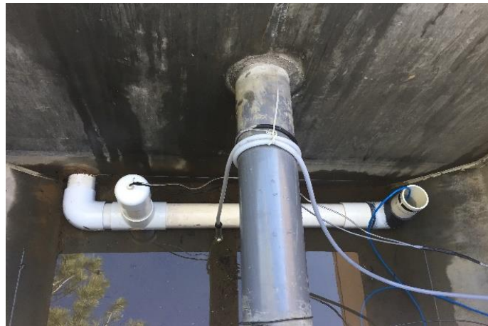
Figure 5-2. Corrected Effluent Flow Monitoring Sensor with Integrated Air Stone
