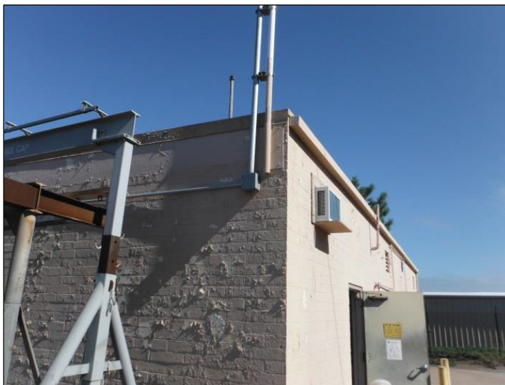
Figure 4-3. Hazardous Storage Building at FRC MFC NBPL San Diego
