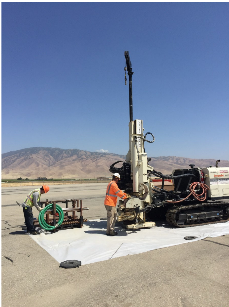
Photo 1 Drilling crew setting up at a soil boring location.
