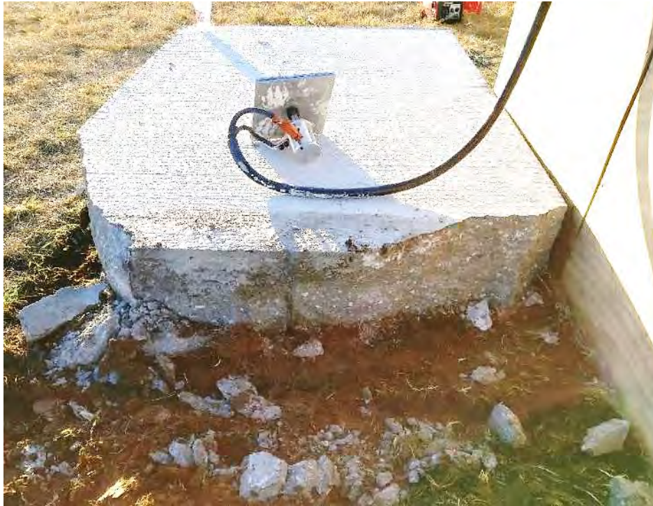
Figure 133. Shot 11: Slab after Removal of Large Concrete Chunks Separated by Shots 8–11
