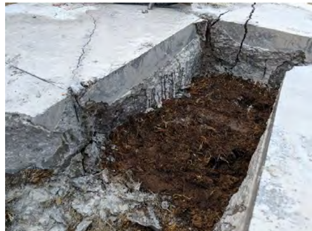
Figure 180. Shot 19: Crack Propagation along Pre-cut Lines from Borehole
