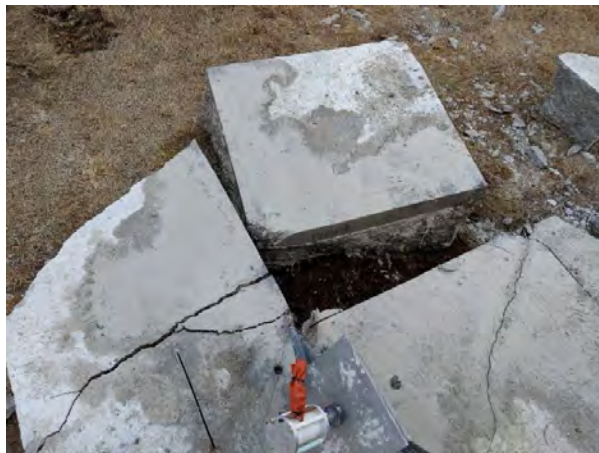
Figure 179. 6-in-deep Pre-cuts Directed Crack Propagation
