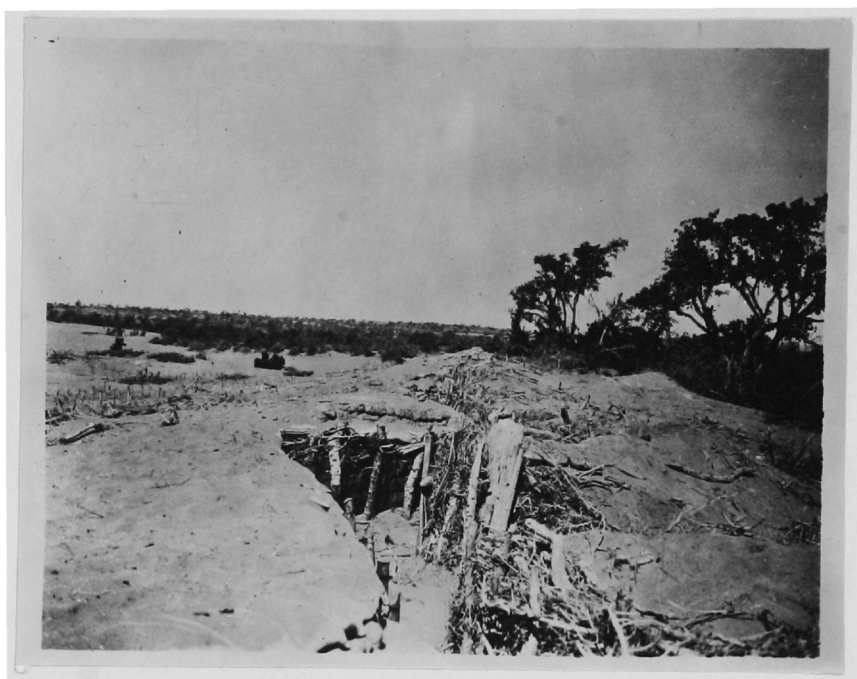
Showing poor revetting material available for Turkish trenches. To get better material they pulled down all the houses of GAZA.
