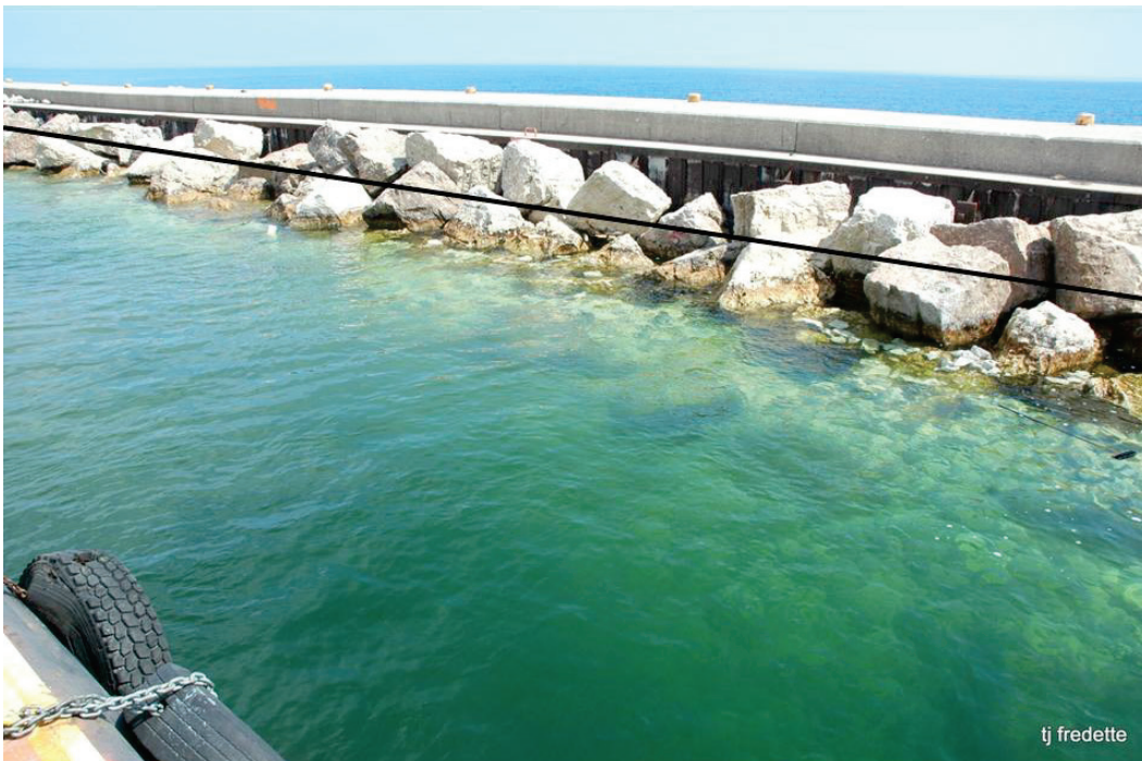
Figure 6. A typical section of the GBW shortly after the stone had been deposited in April 2014. The black line approximates the water level for summer 2015 and 2016, which is about 0.5 m higher. Currently there are numerous caves created by the boulders being inundated; these caves were absent at the time of construction. The caves served as hiding places for diverse fishes to catch prey among the adjacent cobble (Photo: Tom Fredette, USACE).
