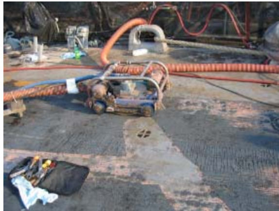
Figure 1 – Nonskid removal by UHPWJ on a flight deck
