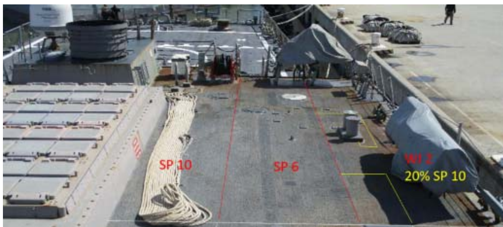
Figure 40 – 19 month follow-up inspection of the shipboard nonskid test on a DDG missile deck
