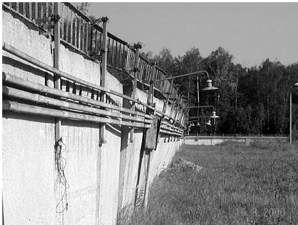
Figure 5: Unstable Perimeter Fence at a Biological Site in Russia, before Security Upgrades
