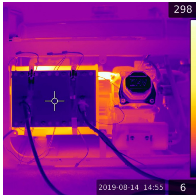
Figure 19. FLIR image of water-cooled prototype
